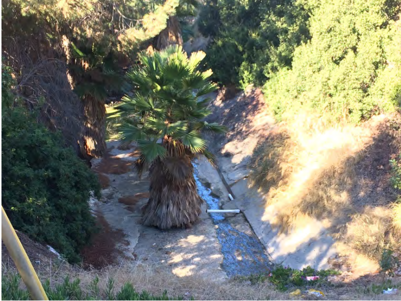
1 – East end of Reach 2, facing west.
