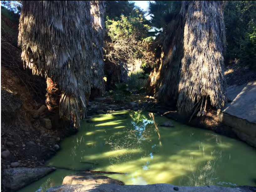
3 – End of concrete-lined channel, facing west.
