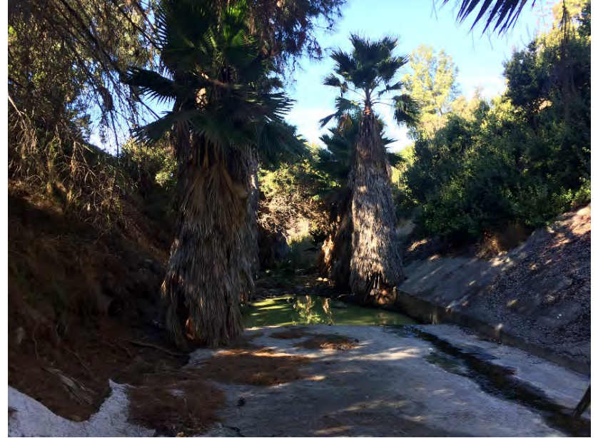
2 – Concrete-lined channel segment facing west.
