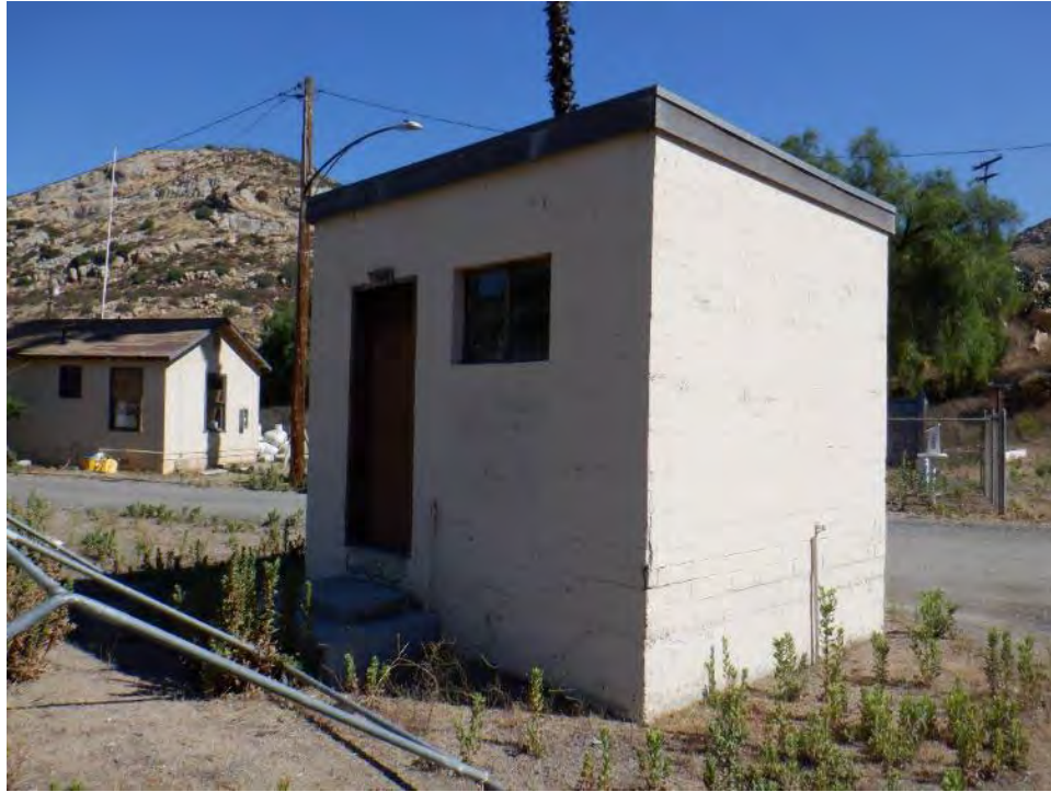
Plate 21. Auxiliary structure, looking north.
