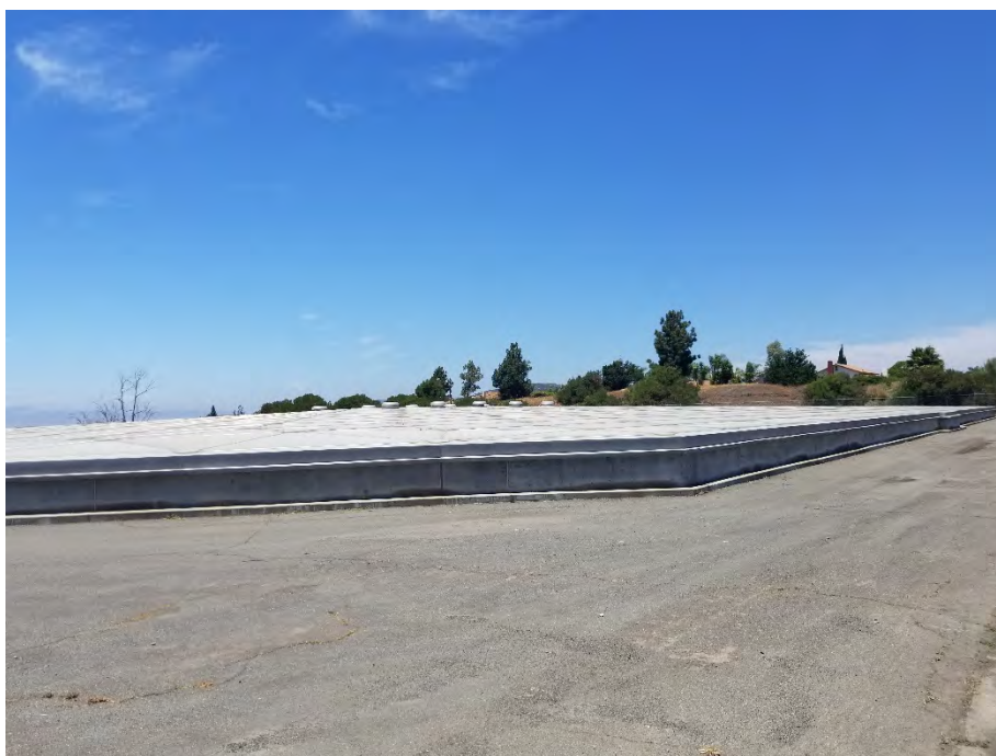
Photo 10: Covered Reservoir (southwest corner). HELIX 2019.
