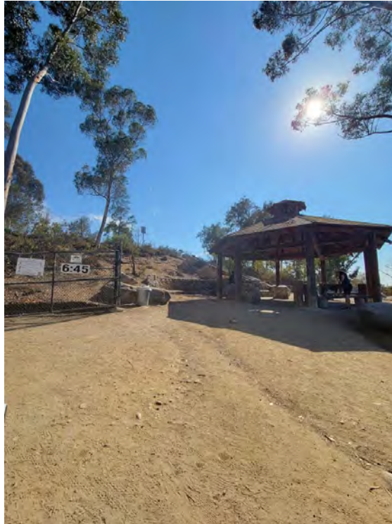
Photo 10. View of shade shelter on earthen embankment. Looking southwest
