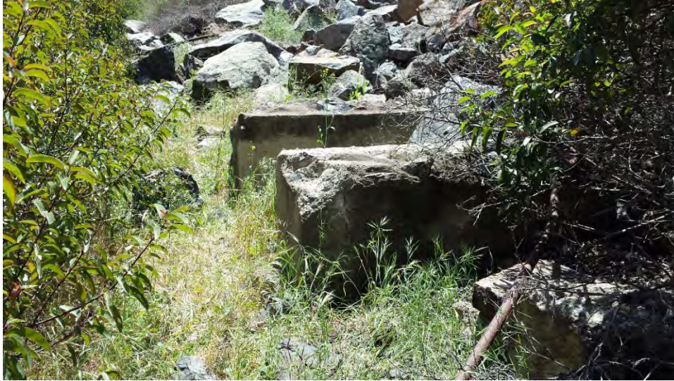
Plate 24. Original dam concrete infrastructure.
