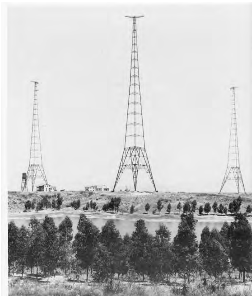
The Naval Radio Transmitting Facility, Chollas Heights, as it appeared upon completion in 1917. "This is a high-powered radio station and contains three 600-foot steel towers, with necessary power house, office building, shop, water tank, main barracks, four quarters for operators and quarters for the officer in charge." —Rear Admiral Roger Welles, first Commandant of Naval Operating Base, San Diego, 1920.
