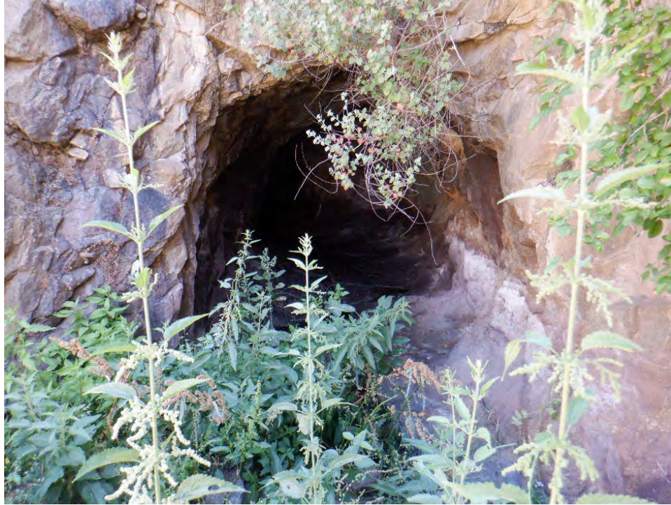
Plate 15. Outlet tunnel entrance, looking southeast.
