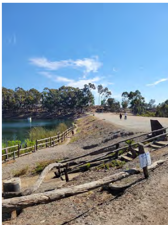
Photo 9. View of walkway and stairs over earthen embankment, looking south.
