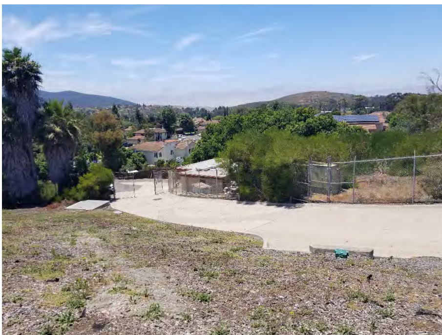
Photo 4: Access Road, Earthen Dam. HELIX 2019.
