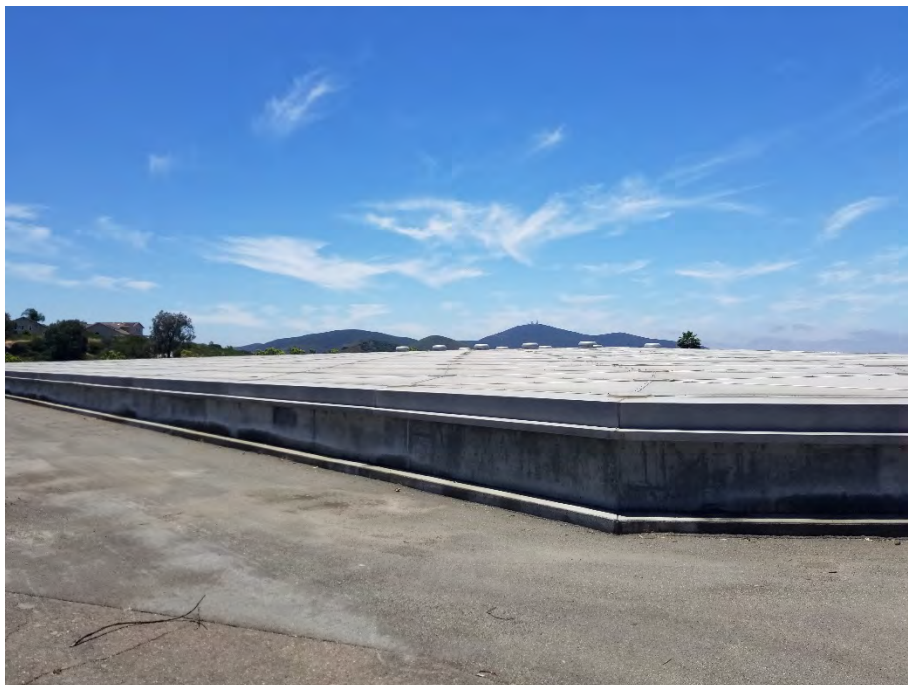
Photo 7: Covered reservoir (southeast corner). HELIX 2019.
