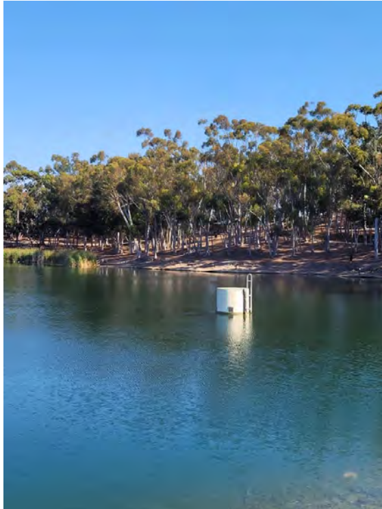
Photo 6. View of outlet tower from earthen embankment. Looking southeast.
