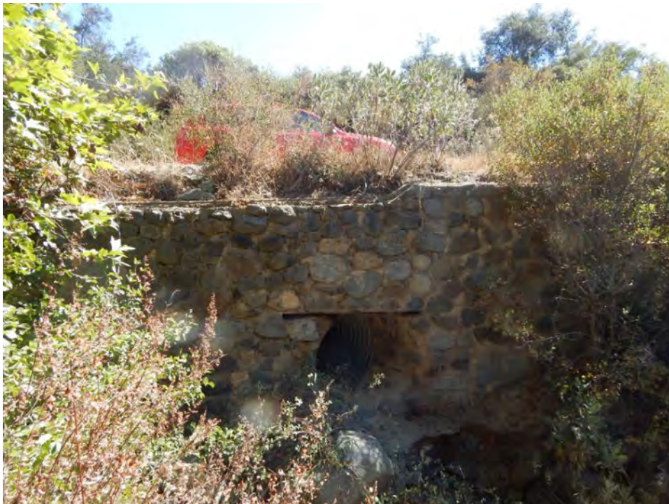
Plate 8. Masonry culvert located on Barrett Lake Road, looking south.
