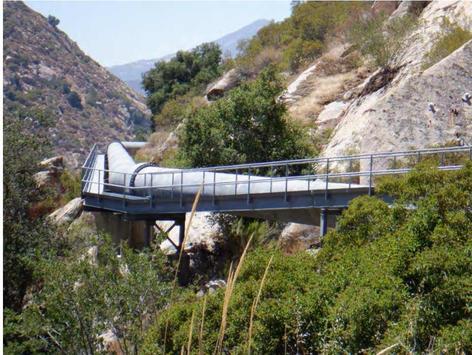
Plate 34. Dulzura Conduit metal flume and trestle near Barrett Dam, looking south.
