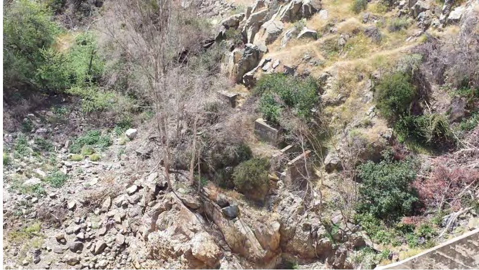
Plate 26. Original dam concrete infrastructure remnant, looking southwest.
