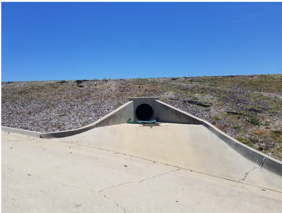
Photo 2: Discharge Outlet and earthen dam, HELIX 2019.
