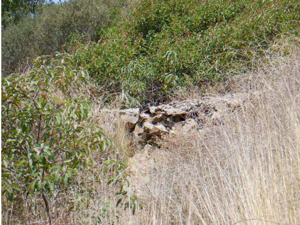
Plate 11. Remnant of masonry structure, looking north.
