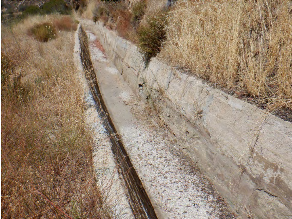
Plate 37. Section of Dulzura Conduit concrete flume near Barrett Dam, looking southwest.
