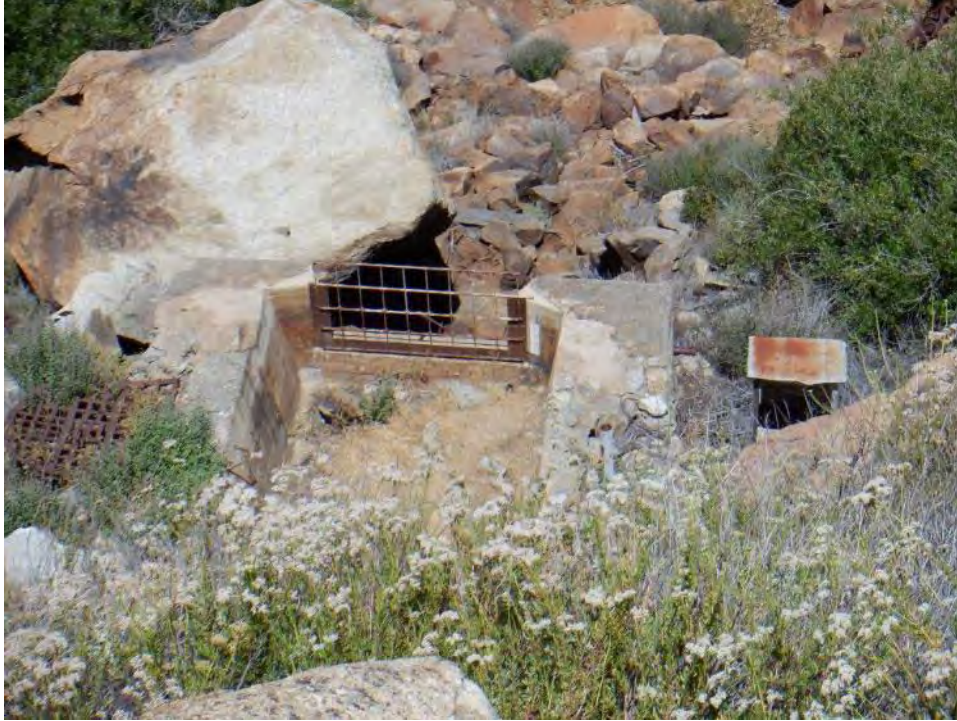
Plate 13. Upper weir and iron outlet gate, looking from above, facing west. The outlet gate is lying on the south side of the weir (left side of the photo).
