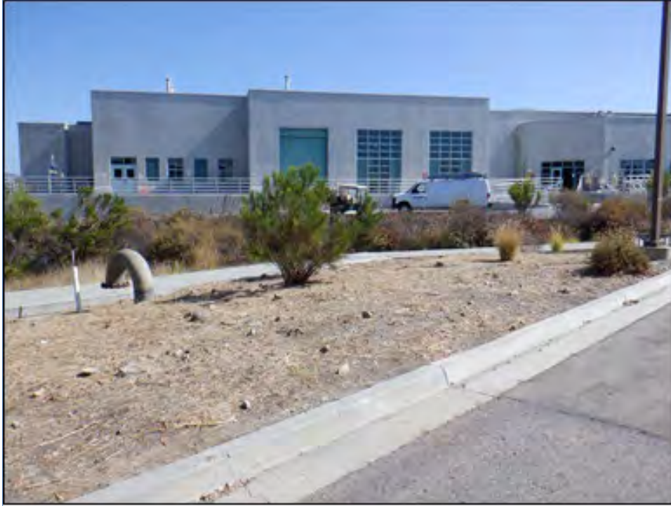
Plate 19. Murray Dam Keeper's House site, looking north.
