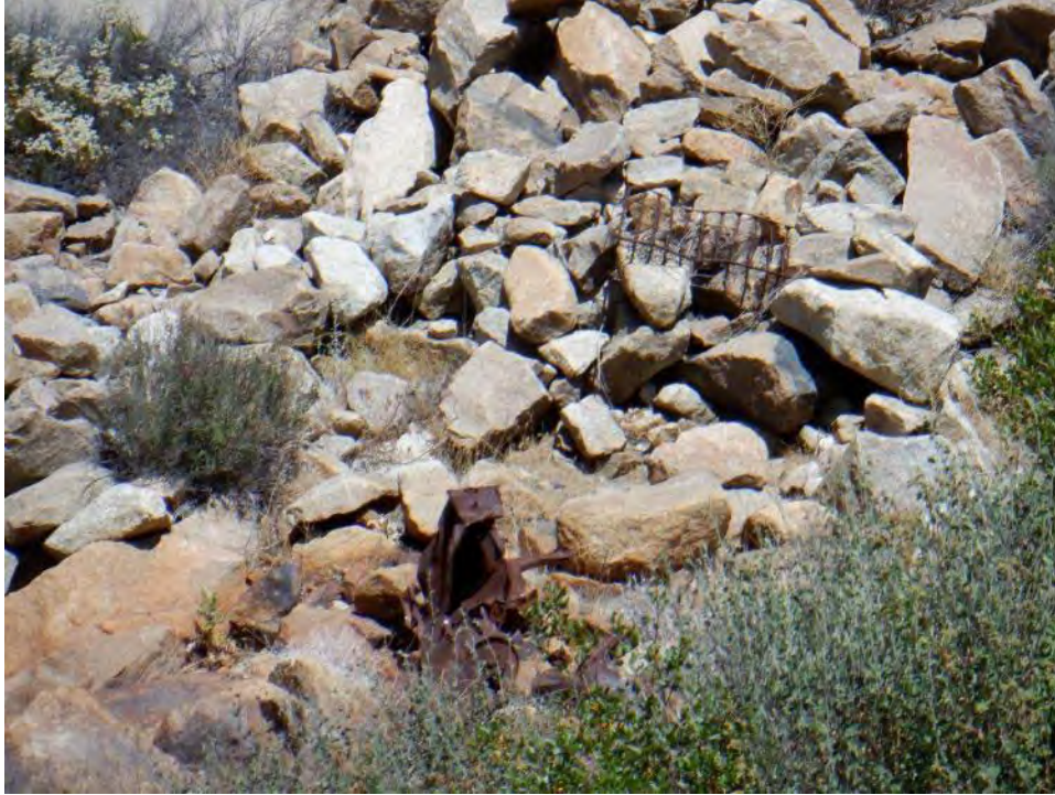
Plate 16. Iron remnants on the downstream face of the dam, looking northwest.
