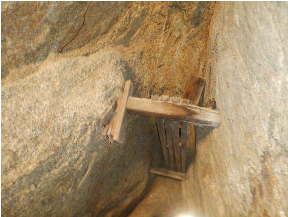
Plate 36. Close-up of timber support structure in Tunnel 2.
