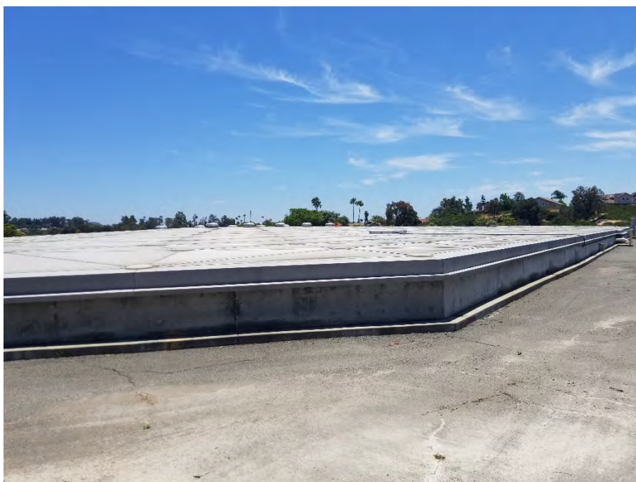
Photo 6: Covered Reservoir (northeast corner). HELIX 2019.
