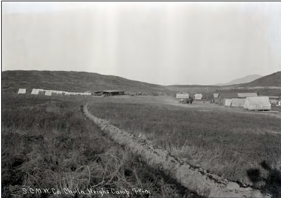
Figure 6: Chollas Heights Construction Camp, 1901 (UCR Collection)
