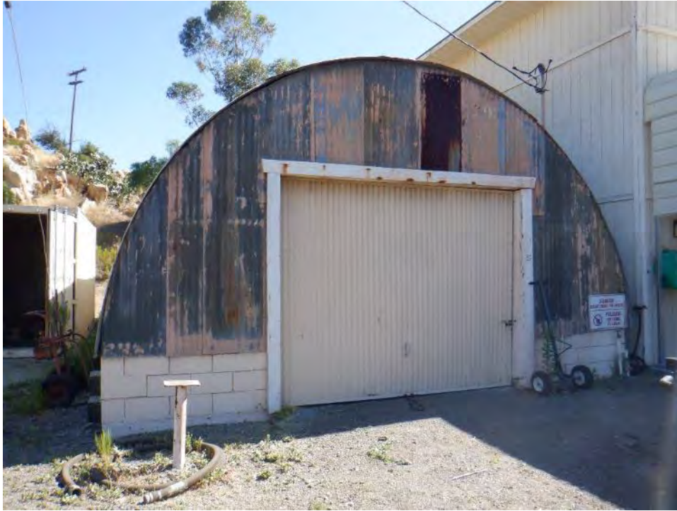
Plate 22. Primary south façade of Quonset hut, looking north.
