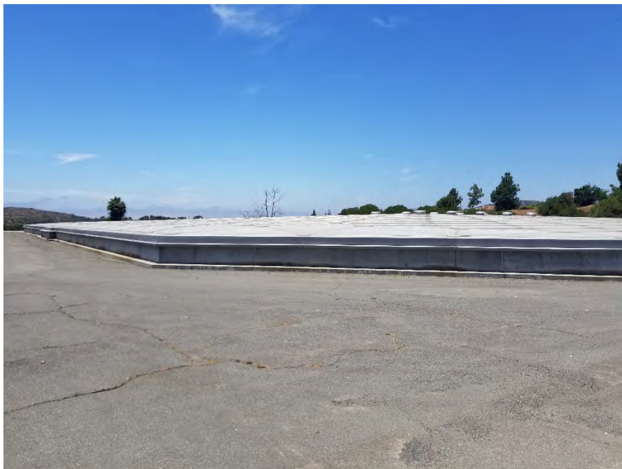
Photo 9: Covered reservoir (southwest corner). HELIX 2019.
