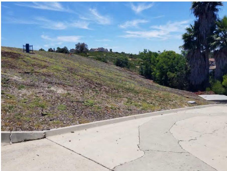
Photo 3: Access Road, Earthen Dam. HELIX 2019.
