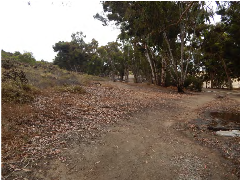
Photo 15. Overview of base of Dam slope. View to the south.
