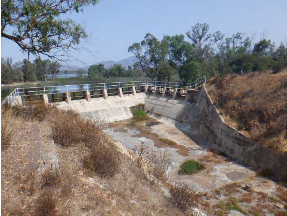
Plate 29. Concrete approach slab on the west side of the spillway, looking north.
