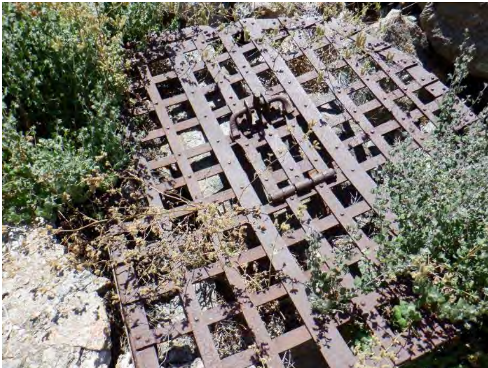
Plate 14. Outlet tunnel iron gate.
