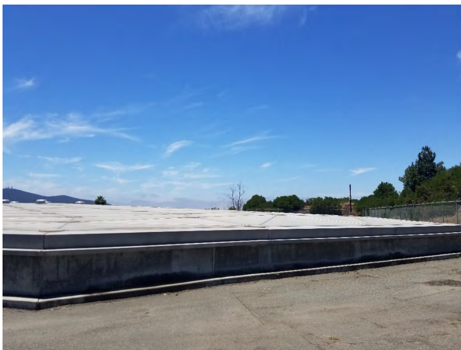
Photo 8: Covered Reservoir (southeast corner). HELIX 2019.
