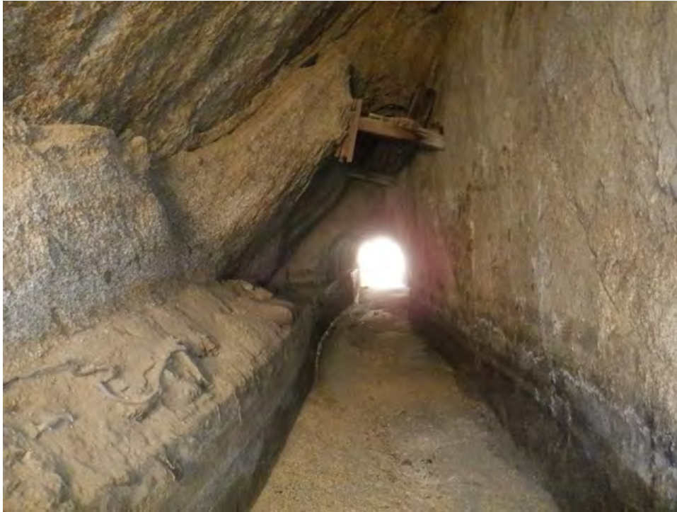
Plate 35. Timber support structure within Tunnel 2, looking southwest.
