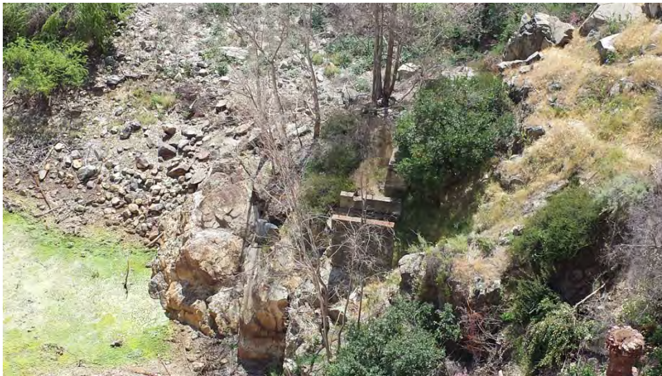
Plate 25. Original dam concrete infrastructure remnant, looking south.
