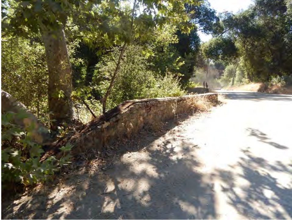
Plate 7. Masonry water crossing on Barrett Lake Road, looking west.
