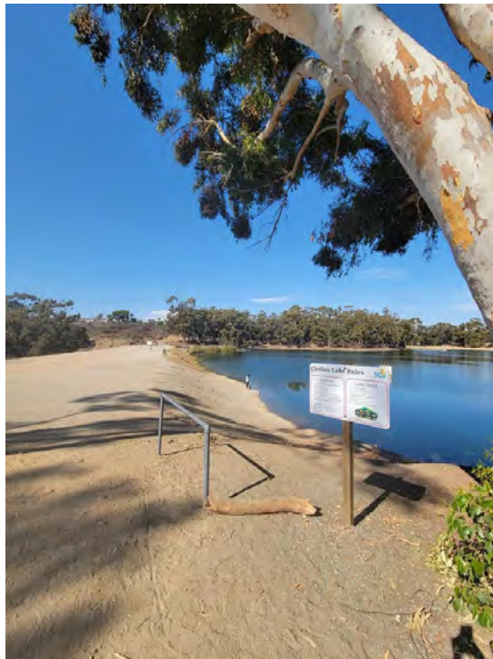
Photo 7. View of walkway over earthen embankment, looking north.
