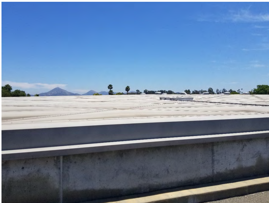
Photo 5: Covered reservoir (northwest corner). HELIX 2019.
