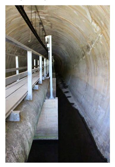
Figure 7. Diversion tunnel with El Capitan Pipeline below concourse, metal and concrete supports visible below (IMG\_2009)
