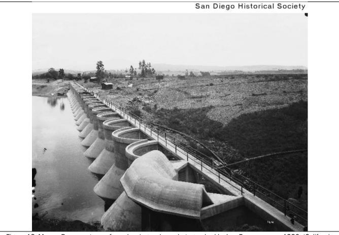
Figure 12. Murray Dam, upstream face showing arches, photographed by Lee Passmore, ca. 1920. (California Border Region Digitization Project: 1870–1939, San Diego History Center)
