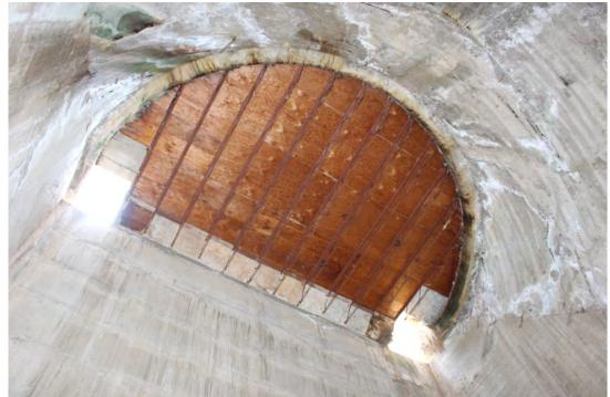
Figure 9. Supporting joists of plywood for the roof structure, view looking upwards, IMG 0522
