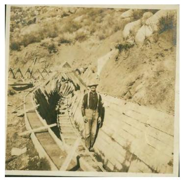
Figure 6. Photograph showing pouring of Dulzura Conduit concrete canals, 1907 (M.M. O'Shaughnessy Photograph Collection, NUI Galway Digital Collections)
