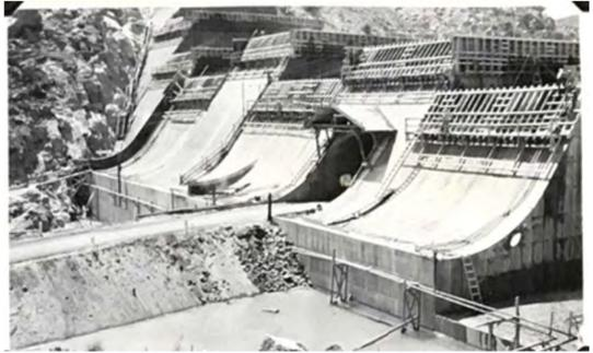
Figure 16. Dam construction showing tunnel through base of the dam, August 1942 (City of San Diego Public Utility Department records)
