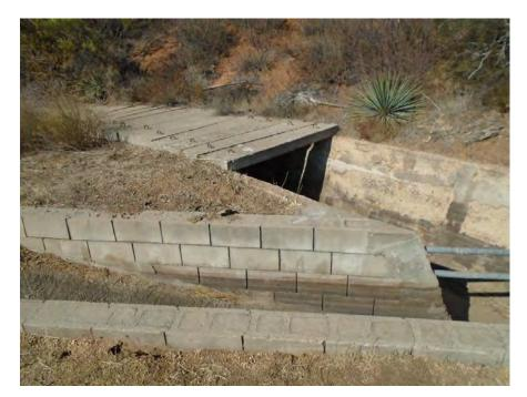
Figure 3. Example of alteration to original line with addition of cinderblocks, DSC00713
