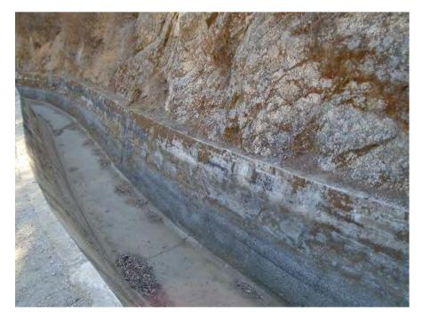
Figure 1. Board formed concrete trench segment, DSC00617
