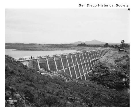
Figure 11. Photograph of completed Murray Dam with the spillway at the bottom left, 1919 (Lee Passmore, San Diego Historical Society Archives)
