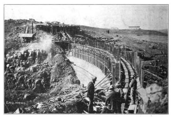
FIG. 11. VIEW OF UPPER OTAY CONCRETE DAM UNDER CONSTRUCTION. Figure 8. Construction of Upper Otay Dam (Engineering News 1904)
