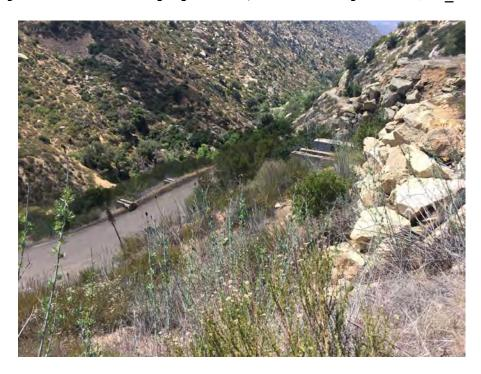
Figure 6. Two pairs of concrete support walls for the concrete sluice, view looking south (IMG\_5936)
