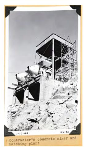
Figure 9. Historical photograph of concrete mixer and batching plant foundation. (City of San Diego Public Utility Department records)
