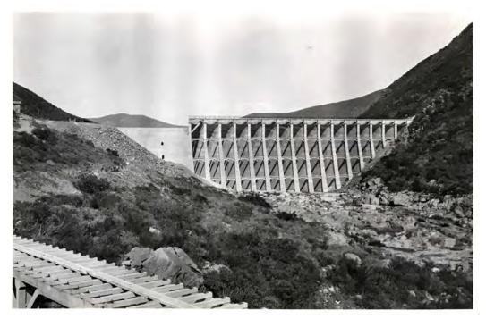
Figure 16. Lake Hodges Reservoir Complex after completion 1919, flume trestle in foreground (Walter L. Huber Papers Collection, Water Resources Collections and Archives, University of California, Riverside)
