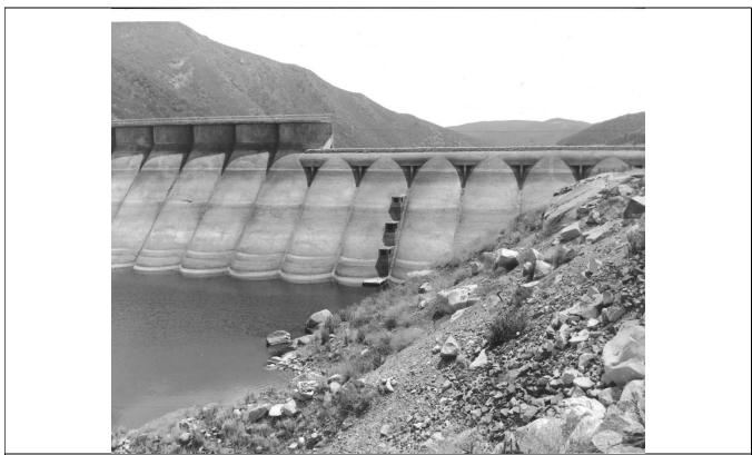
Figure 20. Sutherland Dam, upstream face showing multiple arch type of construction, 1954. (City of San Diego Public Utilities Department Archives, Box 10, Folder 103)
