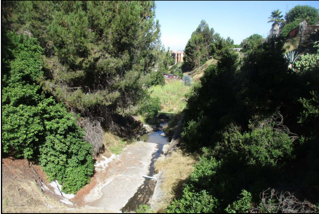
PHOTOGRAPH 3 Slope West of 54th Street, Looking West
