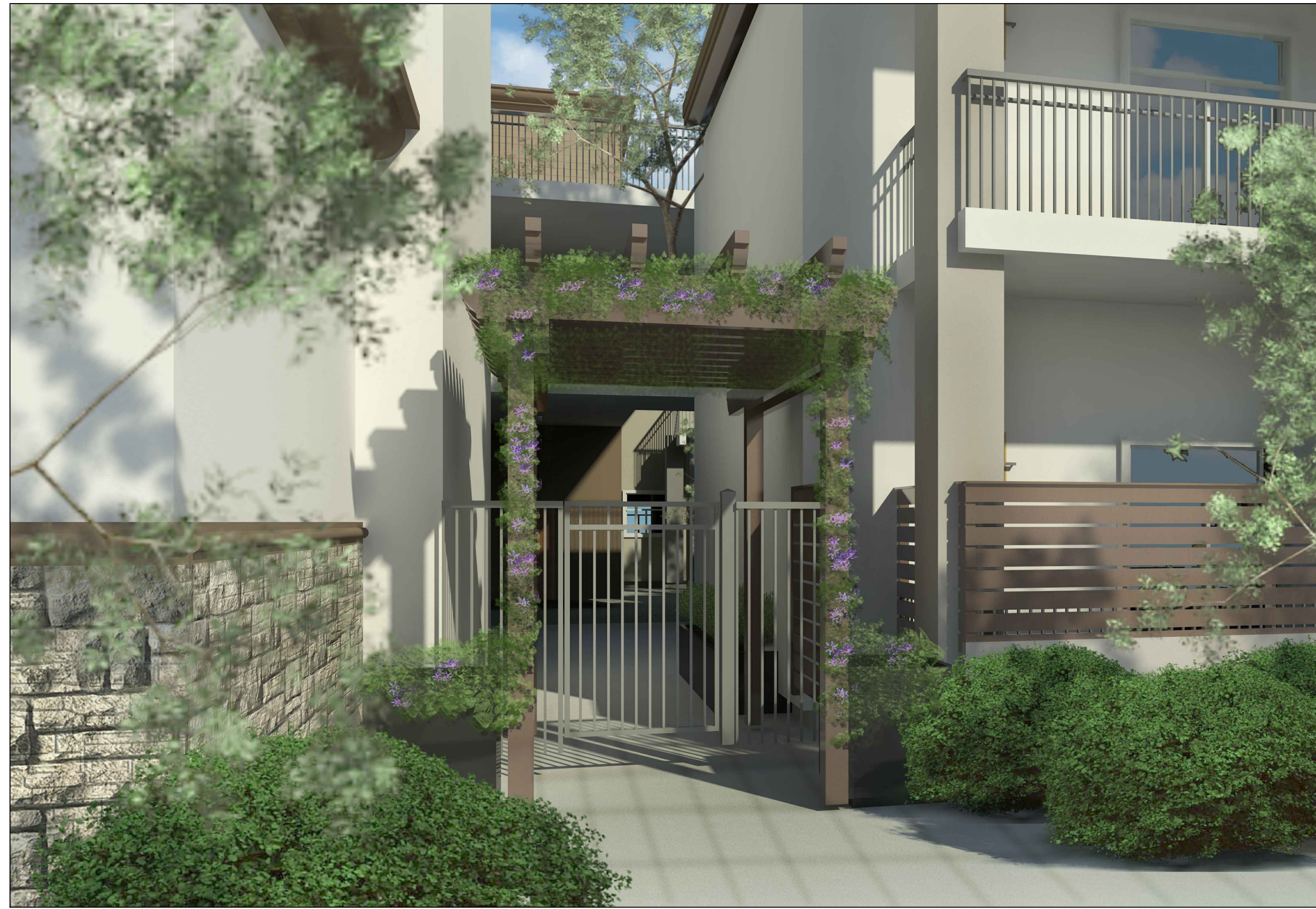
TYPICAL FRONT ENTRY FROM "C" STREET
