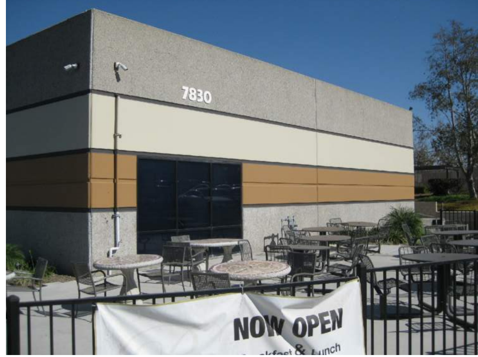
(E) BUILDING RIGHT SIDE
