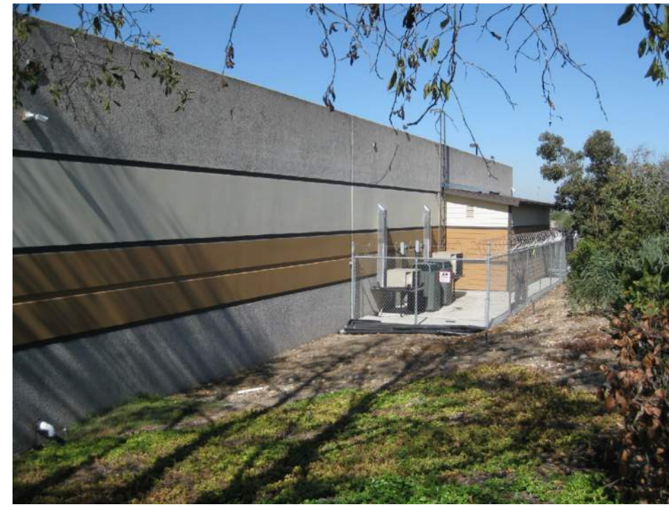
(E) BUILDING REAR
