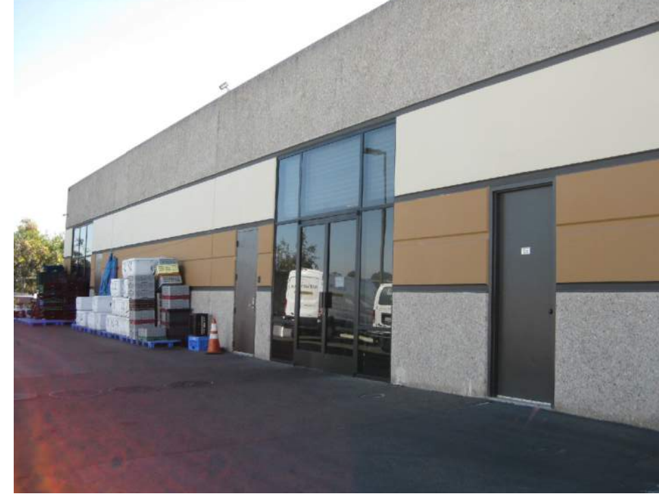
(E) BUILDING LEFT SIDE
