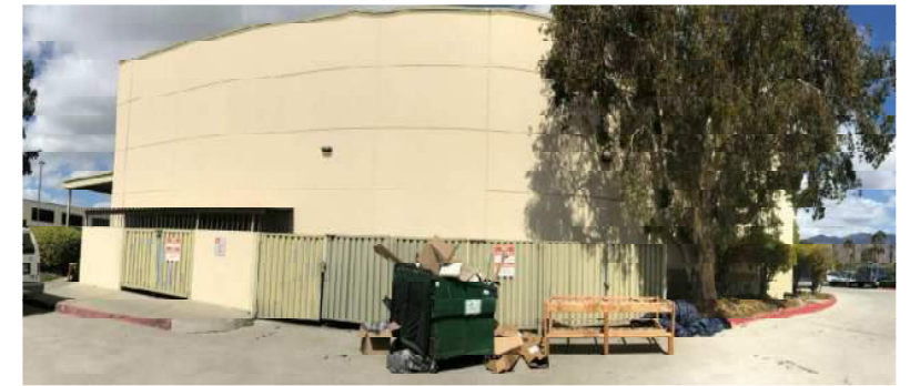
(E) BUILDING SOUTH FACADE
