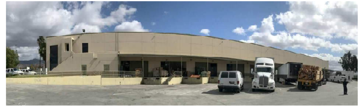
(E) BUILDING WEST FACADE
