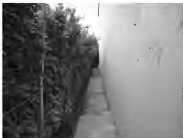
⑤ SIDE YARD VIEW LOOKING NORTH
