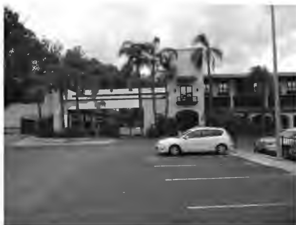
② PARKING LOT LOOKING SOUTH
