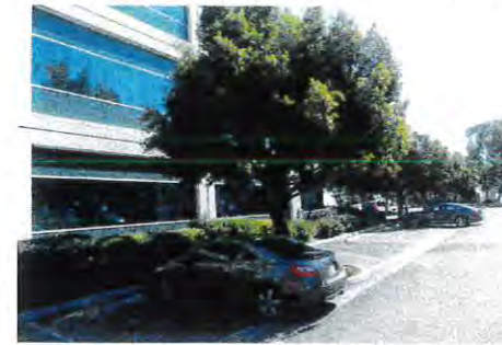
PHOTO 1 LOOKING SOUTHWESTERLY AT BUILDING ZONE ONE
