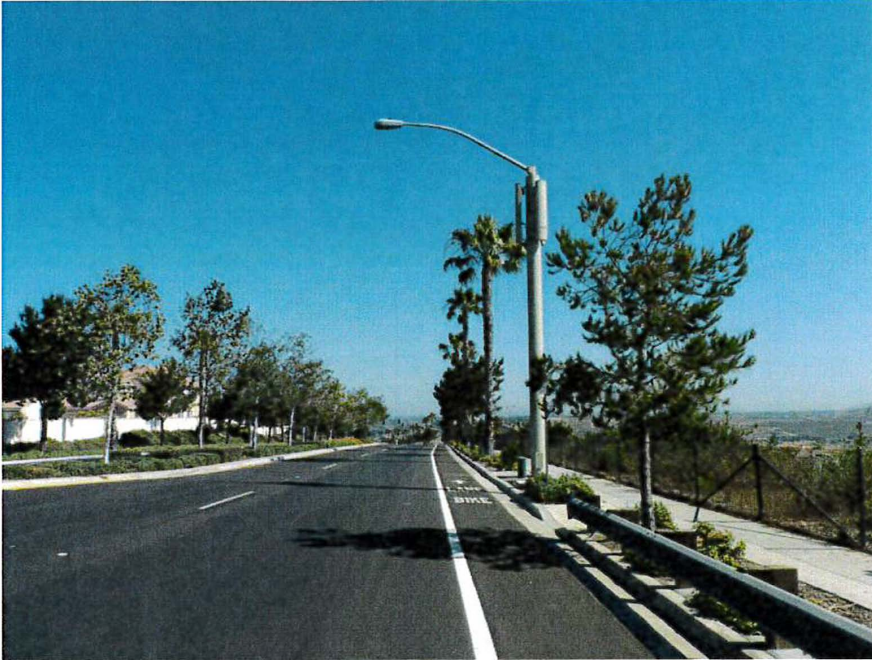
(1) View of the subject property looking north
