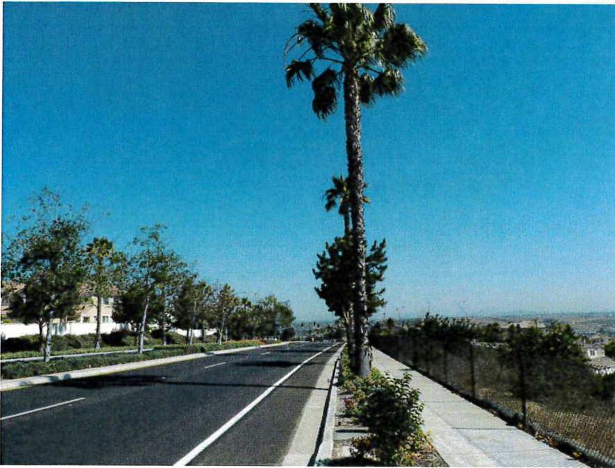
(1) View from the subject property looking north
