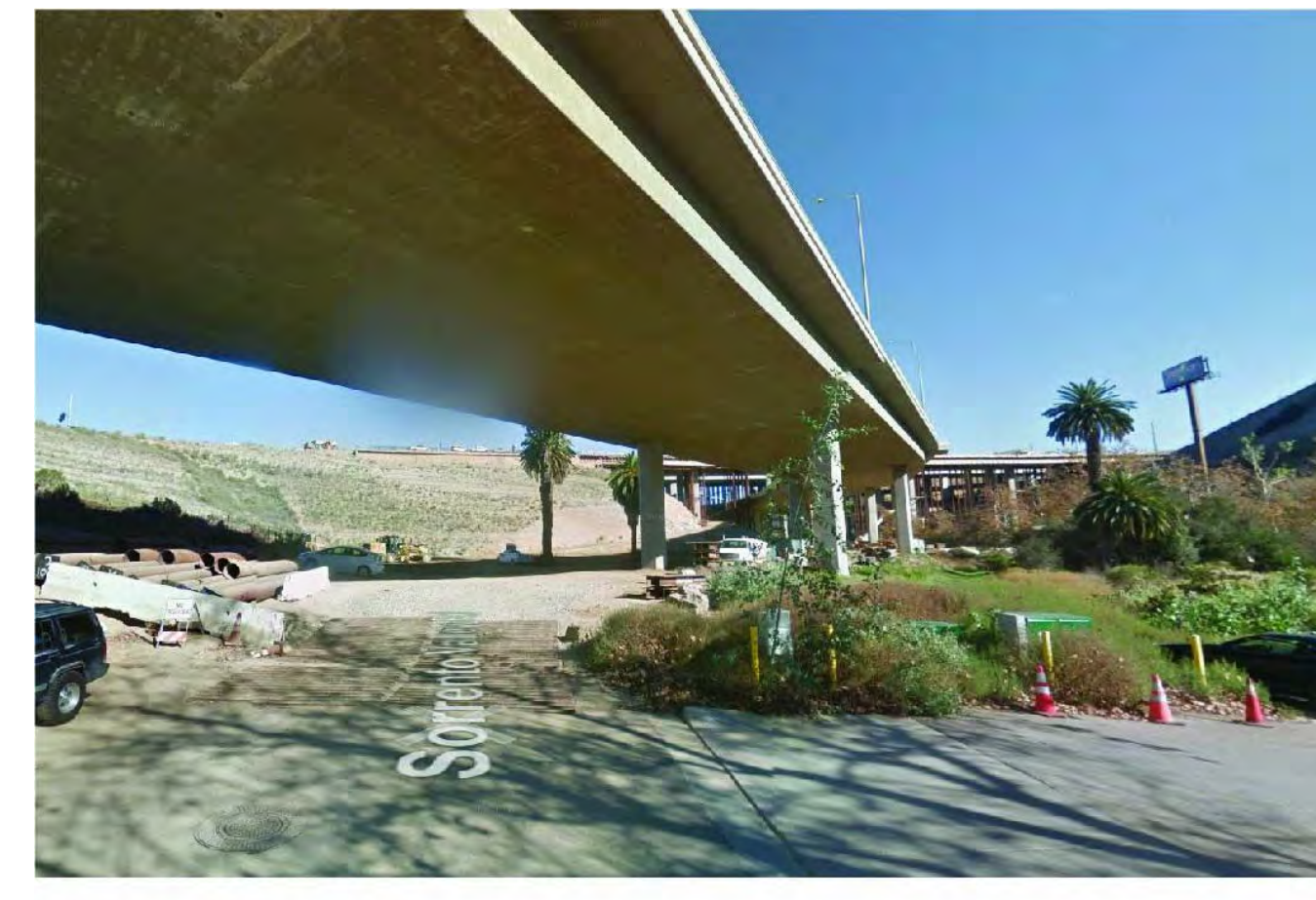
EAST DRIVEWAY - FACING EAST
