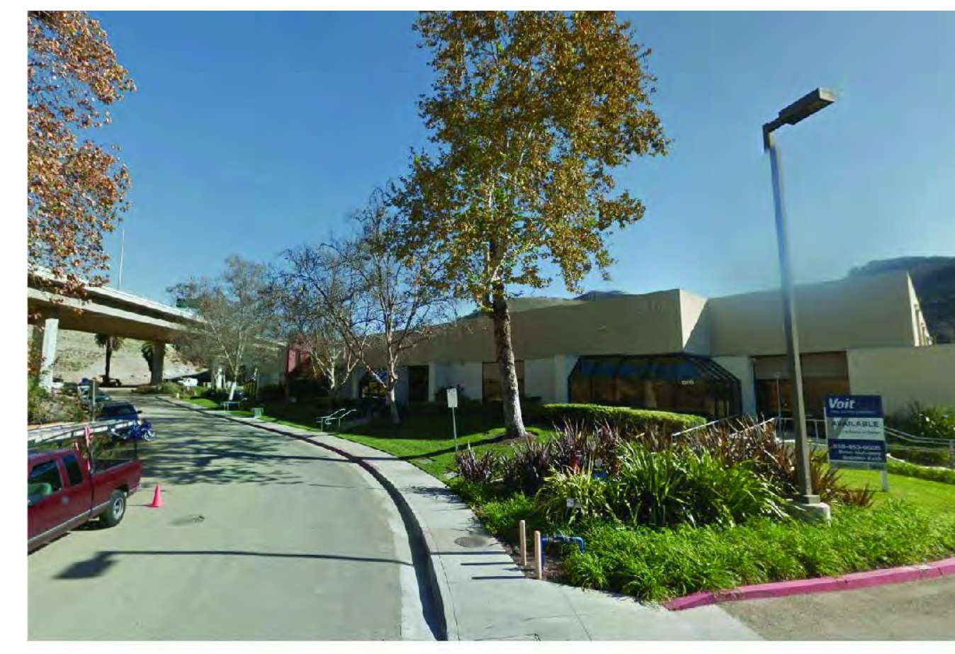
CENTER DRIVEWAY - FACING EAST
