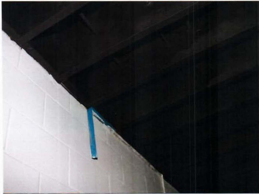
Image #1 shows the joist perpendicular to CMU wall Without any tie connection to two story CMU wall
