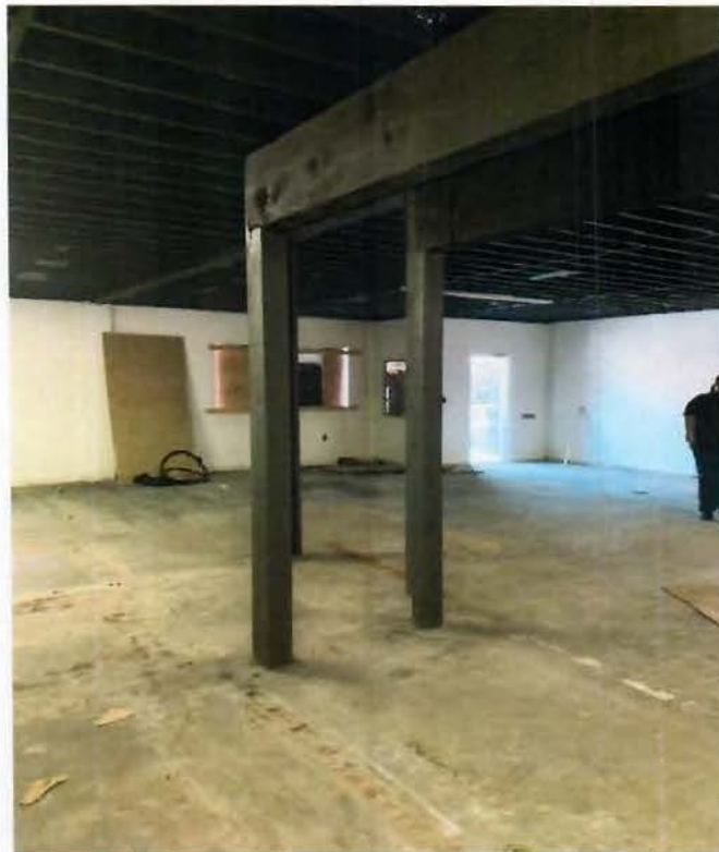
Image #3 shows the floor joist supported with wood beam which support with 2-2x6 stud
