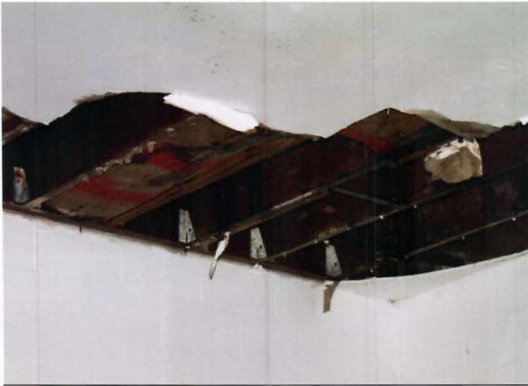
Image #7 shows the roof framing deteriorated wood as well as notched joist
