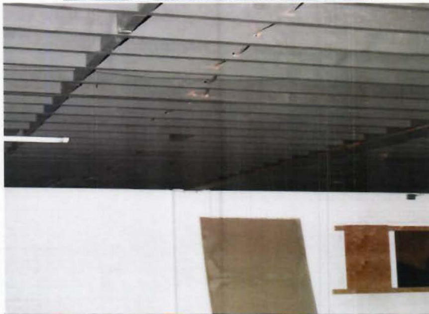
Image #1 shows the joist perpendicular to CMU wall Without any tie connection to two story CMU wall
