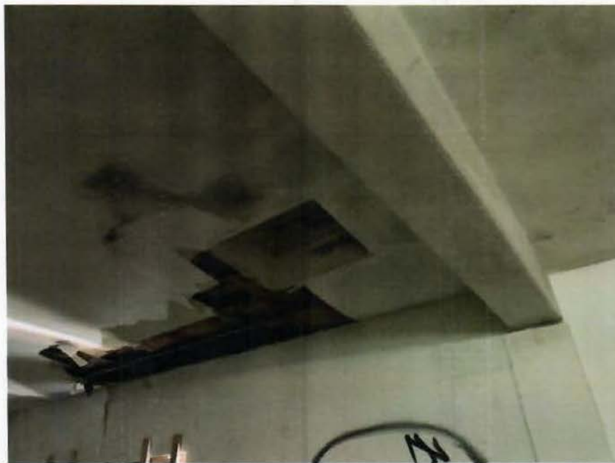
Images #4 shows the concrete beam support the flexible diaphragm and deterioration of the roof framing
