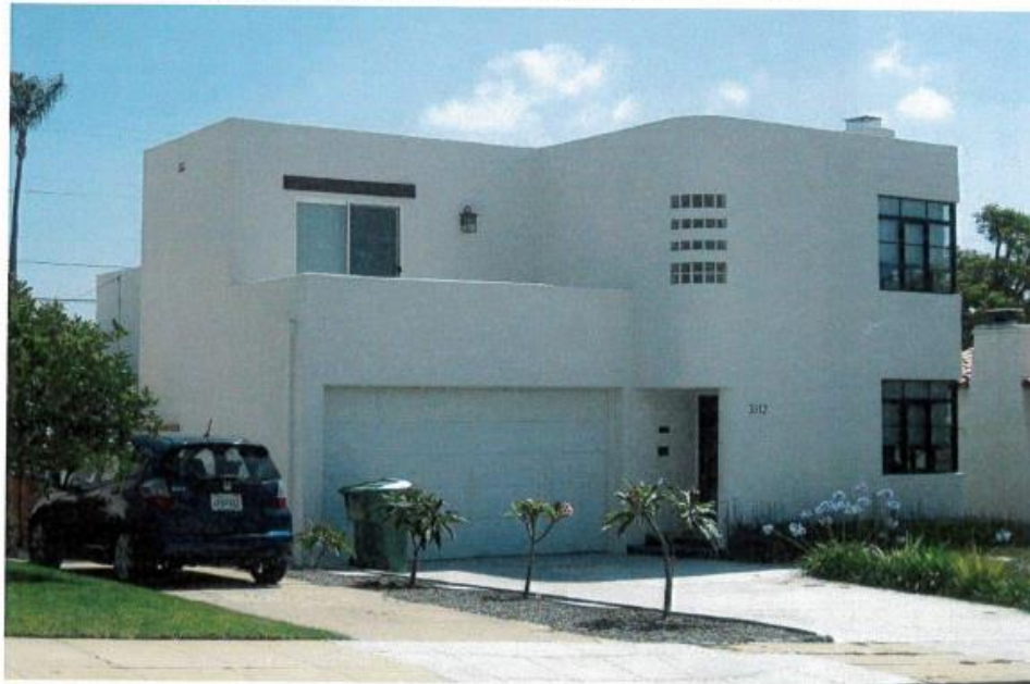
Photo 1: Looking southeast at the primary facade.
