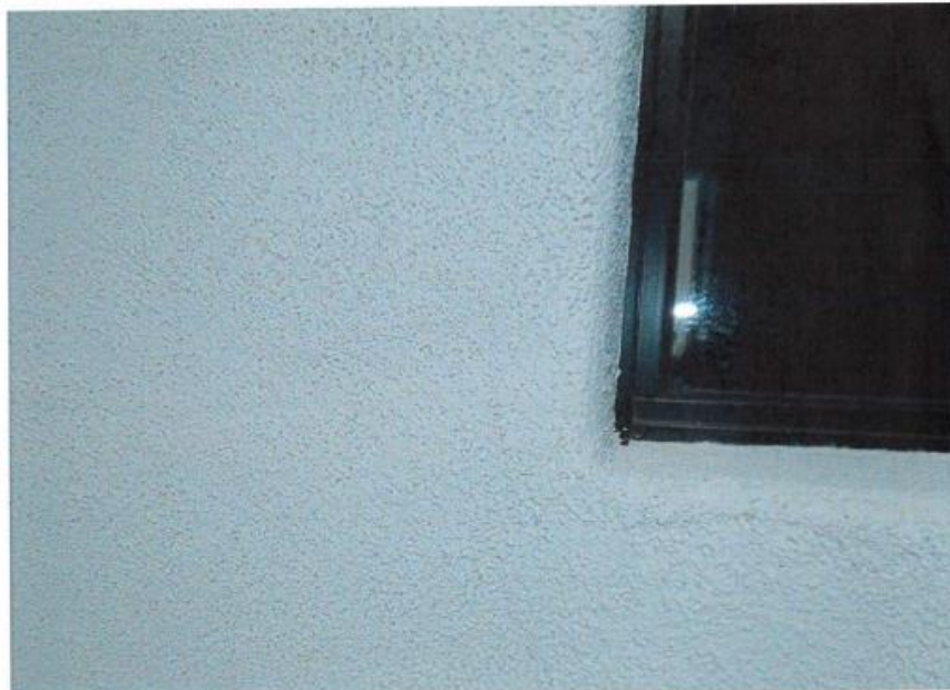
Photo 3: Detail of the re-stucco exterior finish.
