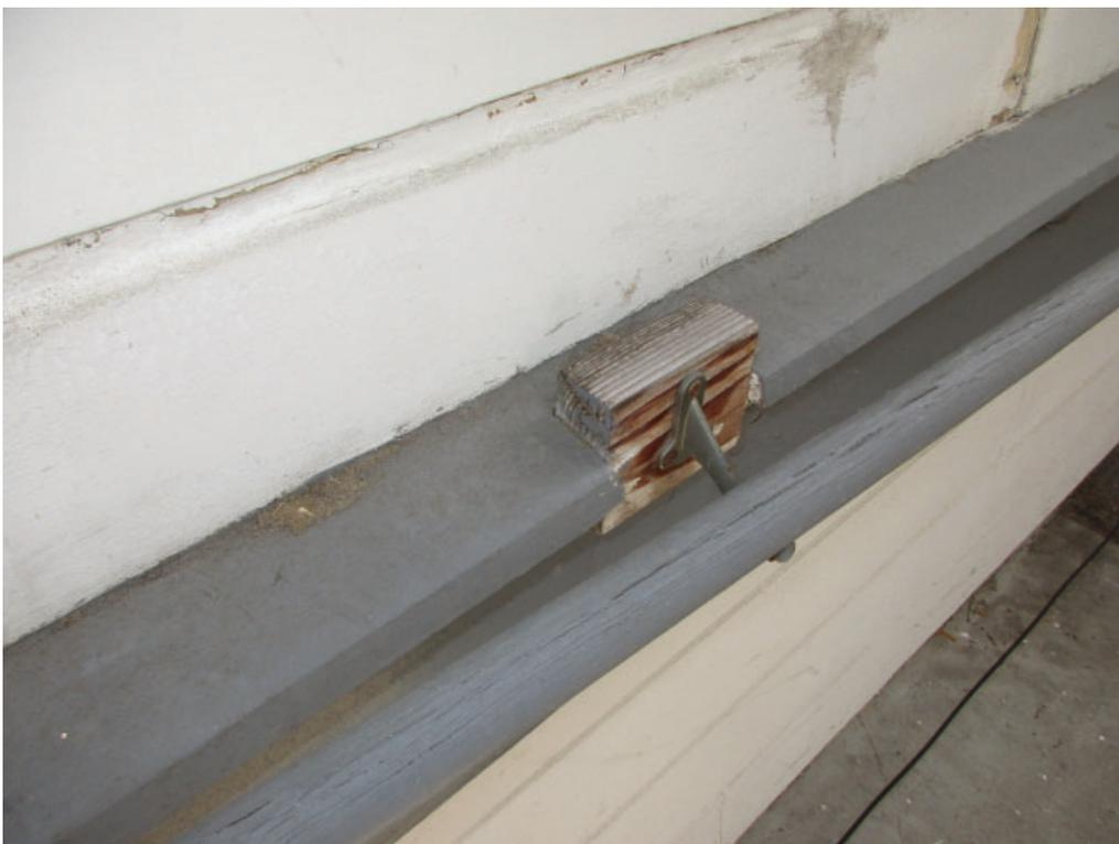
Figure 3-14: Detail photo showing the impact to the base trim boards from the accessibility ramp handrail attachments.
