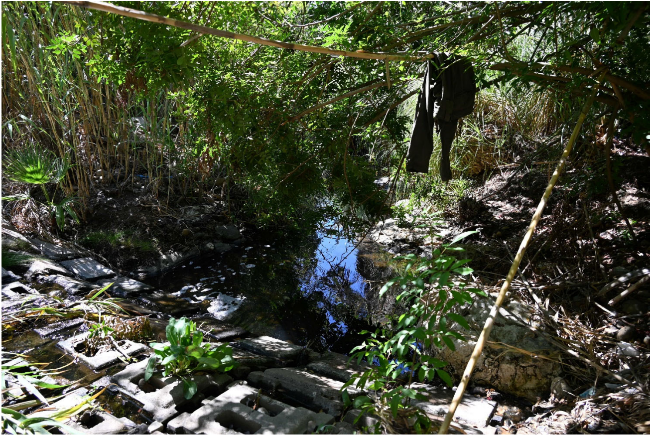
Figure 5. Looking Downstream towards Reach 2 from Upper End at First Grade Control
