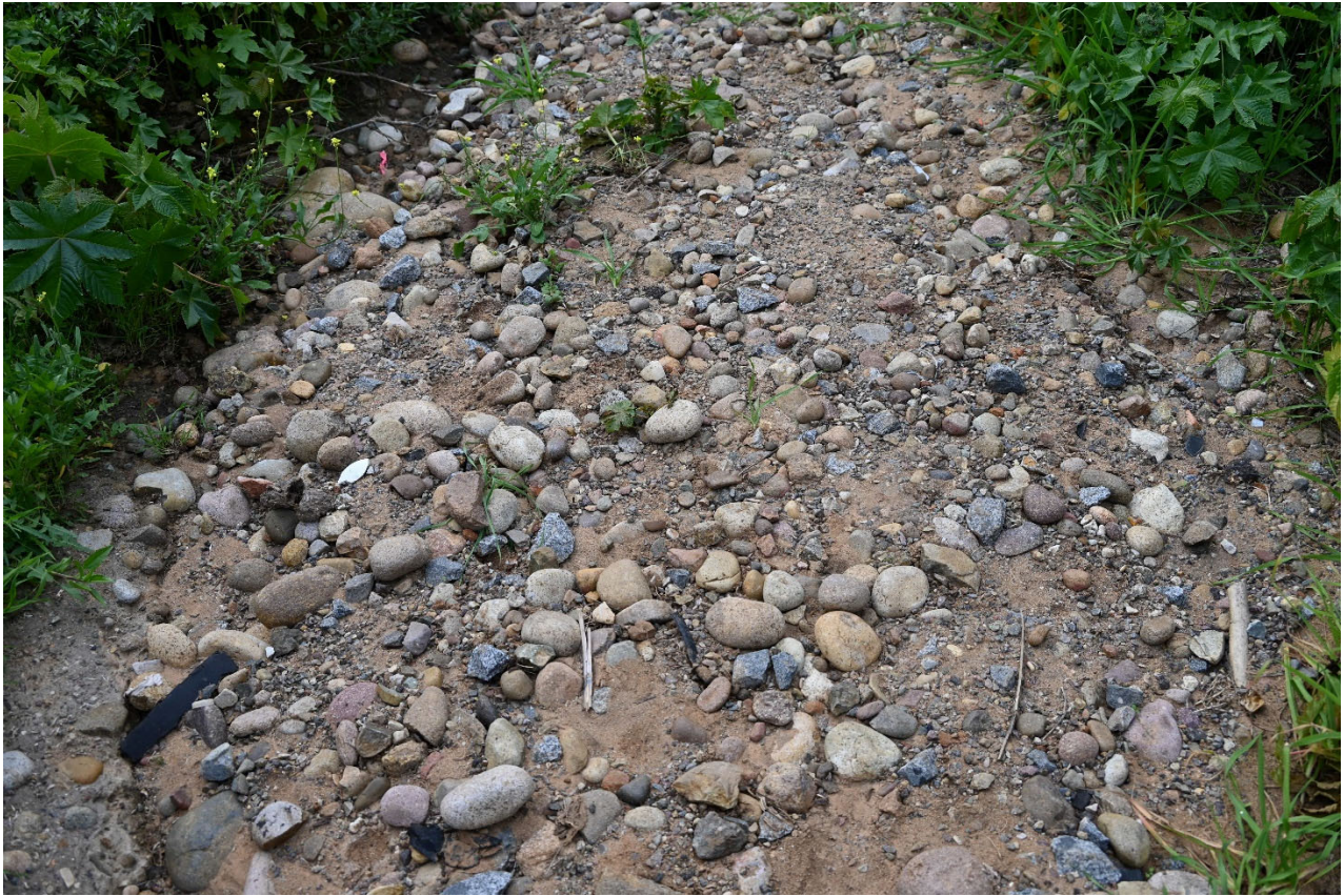
Figure 11. Cobble Lining Along Reach 1
