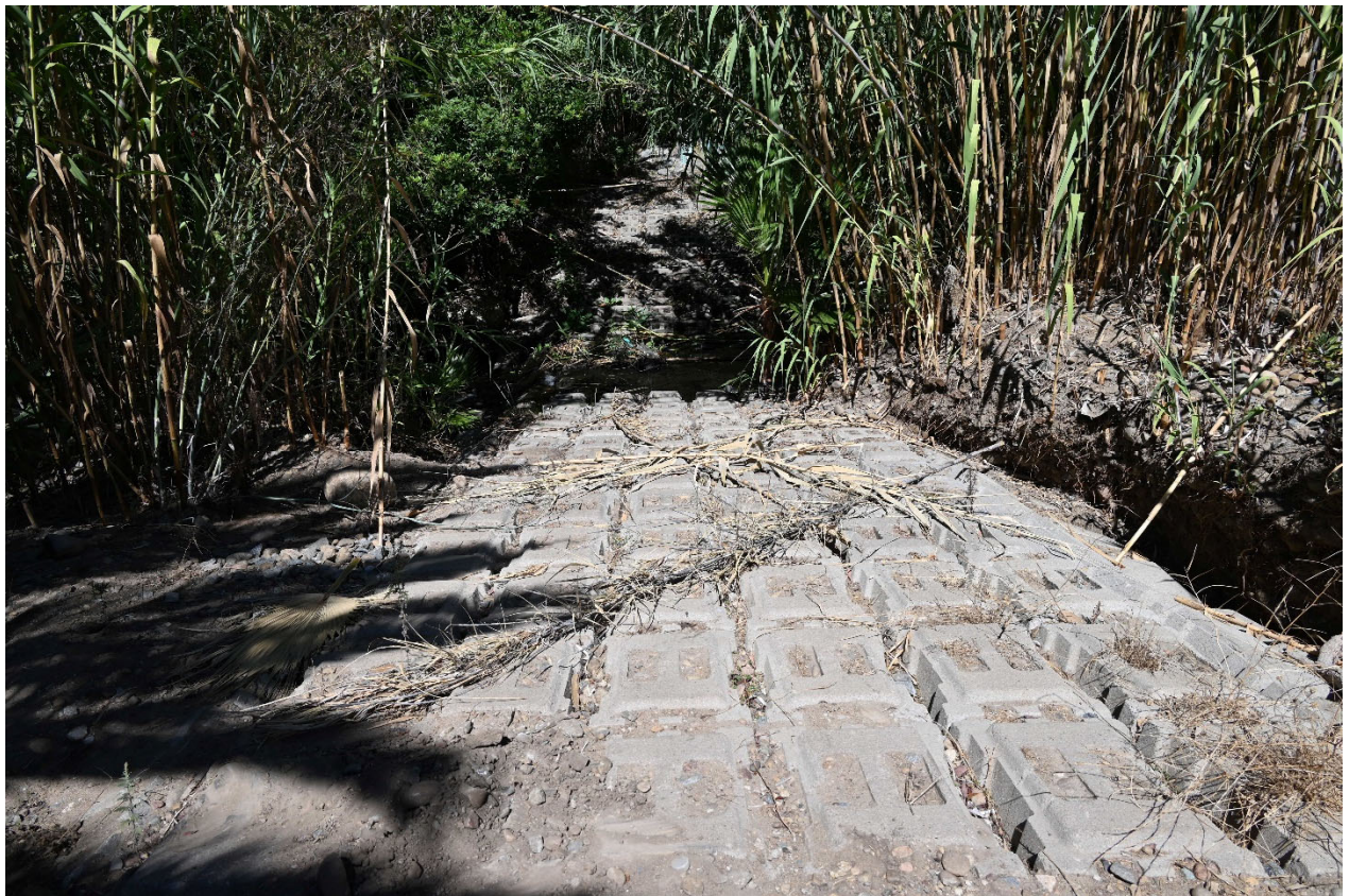
Figure 4. Articulated Concrete Block Grade Control between Reach 1 and 2
