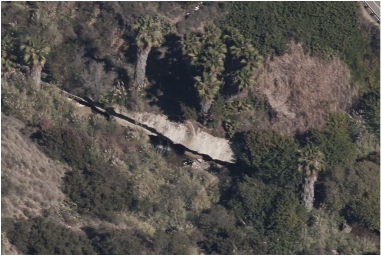
Figure 7. Concrete Channel at Lower End of Reach 2 (Second Grade Control)
