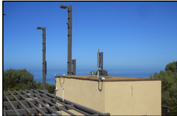
Temporary Antennas on Equipment Shelter Rooftop
