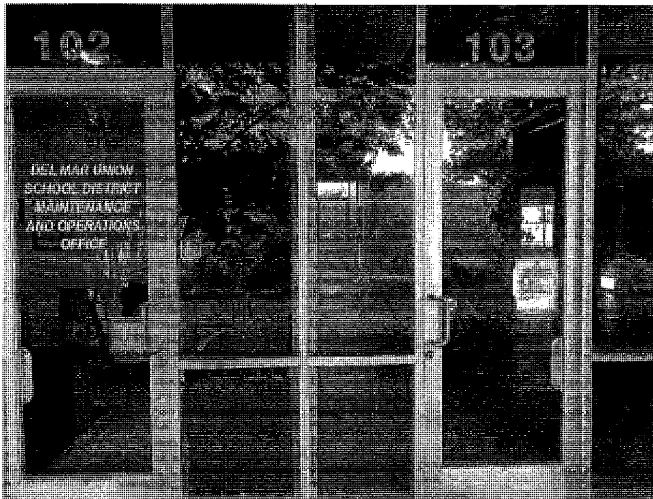
Entrance to DMUSD Offices, Unit 102. Entrance to proposed Marijuana Outlet, Unit 103
