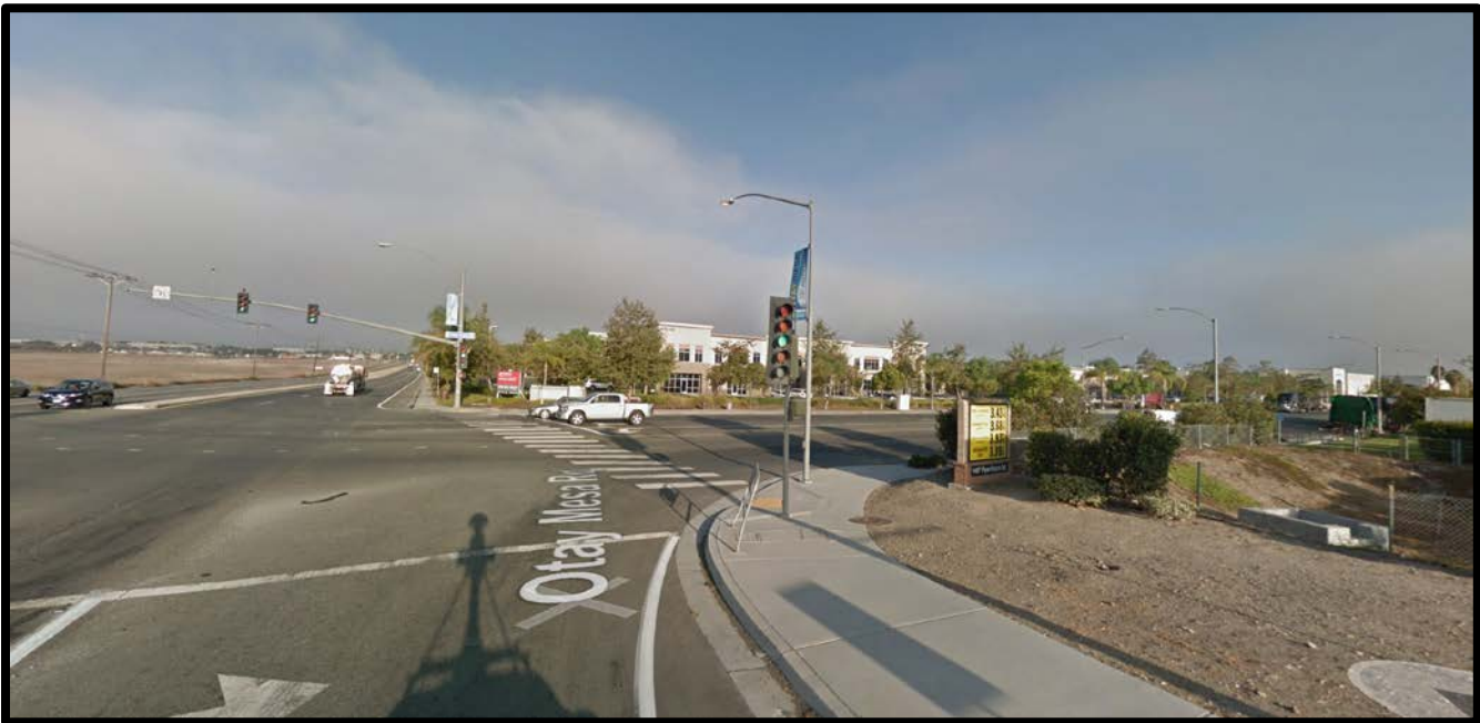
Looking west at intersection of Otay Mesa Road and Piper Ranch Road. Existing commercial and industrial development on the right, vacant project site on the left.
