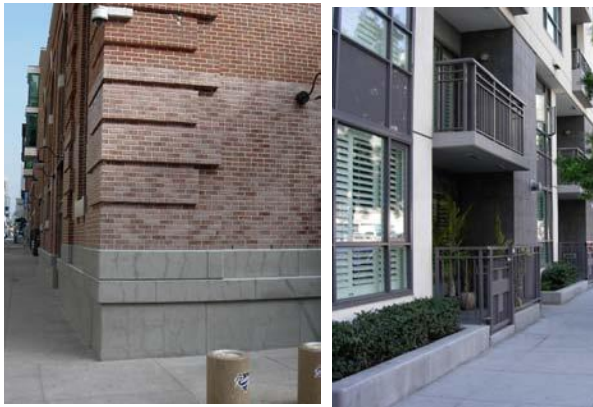
Building design should use a durable upgraded material for the building base. Above, San Diego, CA.
