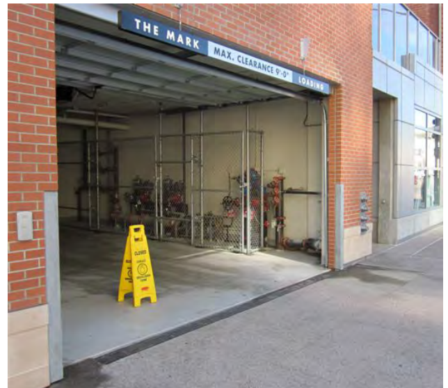
Backflow-prevention devices are to be located in a building alcove, landscaped area, or utility room within the building, outside of the public right-of-way, and completely screened from view. Above, San Diego, CA.
