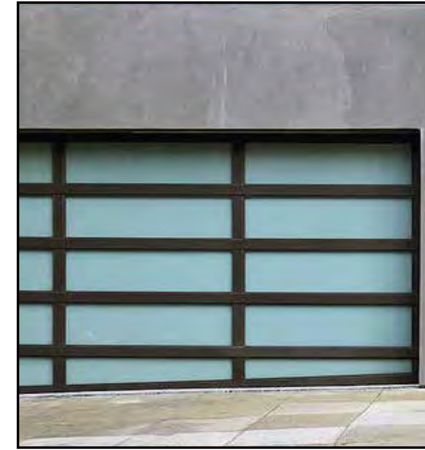
GL-04 Description: Pre-Finished Garage Glass Door Color: Clear Location: Parking Entry Door, Loading Door
