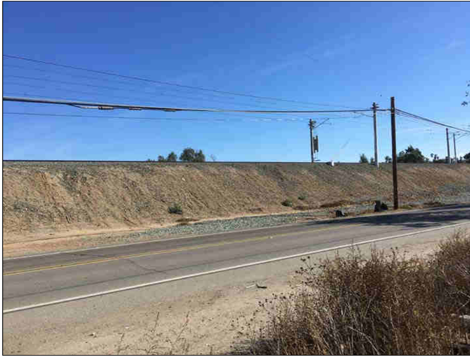
Photograph #11 Hollister Street and San Diego Trolley line to the east.
