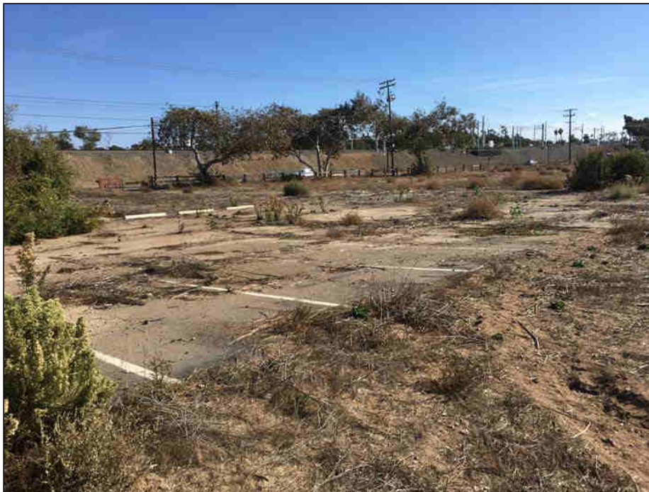
Photograph #7 Asphalt paving in northeastern portion of the Site.
