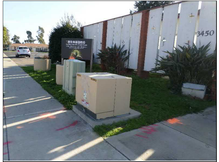
20. Pad-mounted transformer
