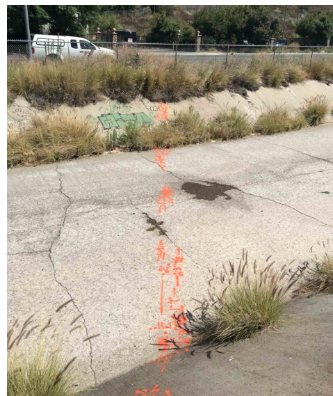
Figure 7: Markout from Duct-Rodding
