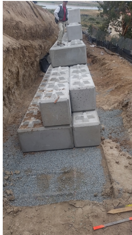
Figure 10: Typical Enviro-Block Wall Installation
