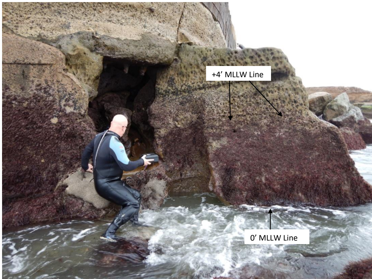
Figure 3. Small opening observed along the existing vertical seawall. The vertical limit of marine algae growth along the vertical seawall as shown here marks the +4' MLLW elevation boundary. Elevations are approximate and based on rough measurements to the water line and observed tidal elevations at Scripps Pier (NOAA Tidal Station 9410230).
