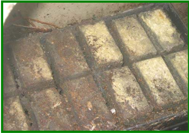
Remove Spent BioMediaGREEN Filter Blocks
