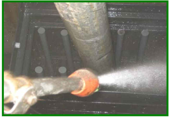
Spray Down and Clean Cartridge Filter Housing
