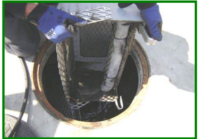
Remove Catch Basin Filter
