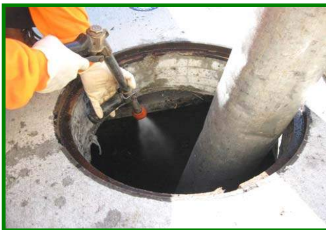
Vacuum out the Sediment Chamber
