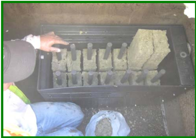
Replace with New BioMediaGREEN Filter Blocks and Replace Lid, then Catch Basin Filter and Replace Manhole or Grate
