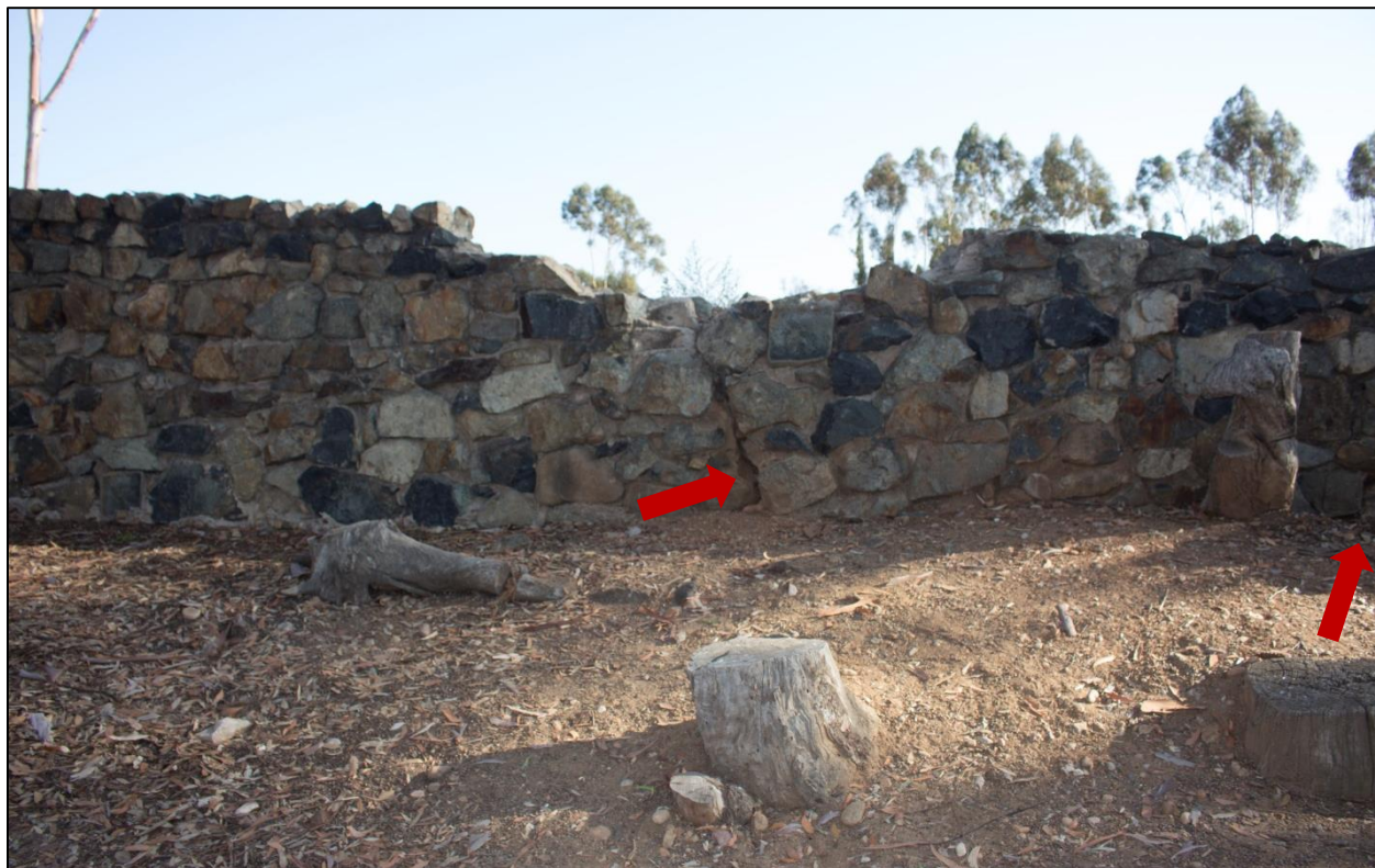
Figure 16. View of wall section showing missing portions and cracks (red arrows) (Photo credit: Dudek).
