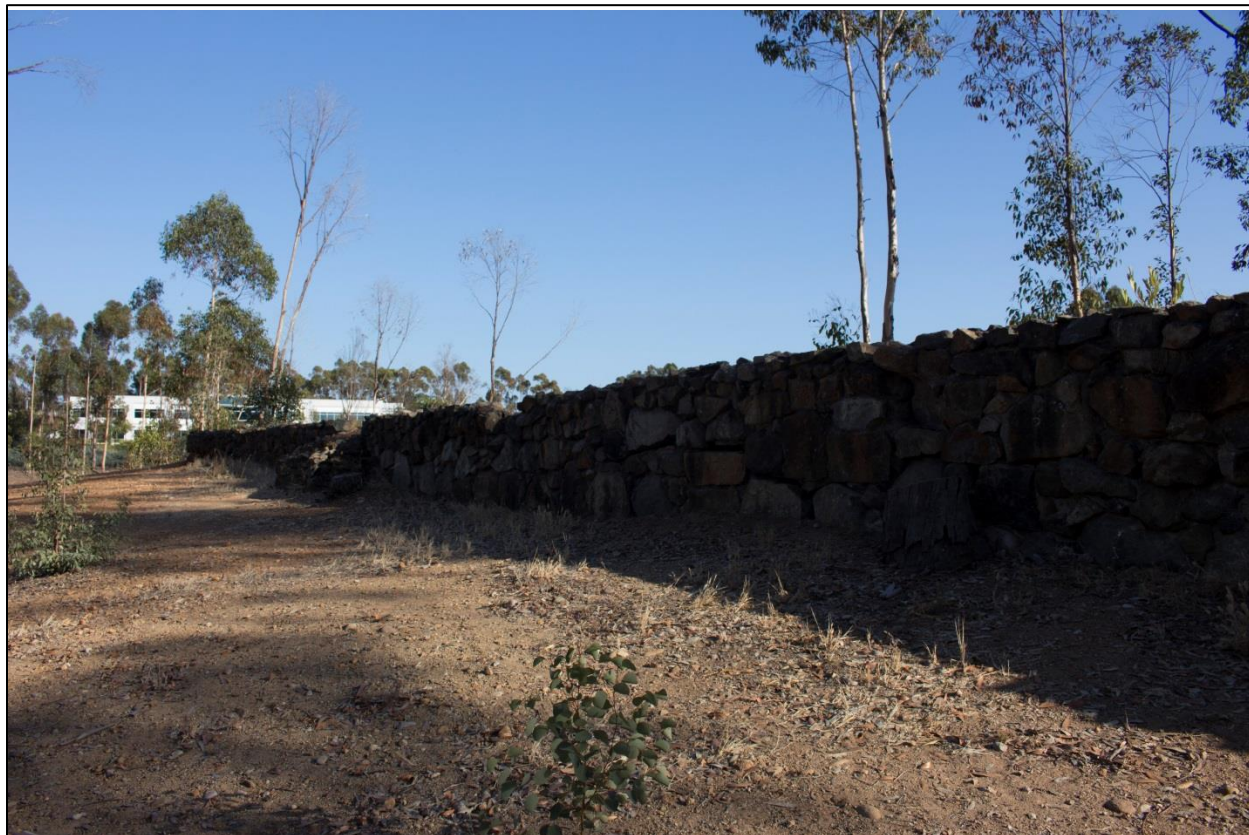
Figure 18. Length of wall; notice the large crack near center-right of the picture (Photo credit: Dudek).
