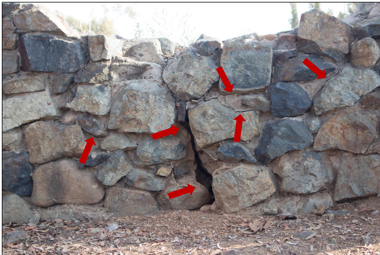
Figure 17. Detail view of above wall section showing missing portions and cracks (red arrows) (Photo credit: Dudek).
