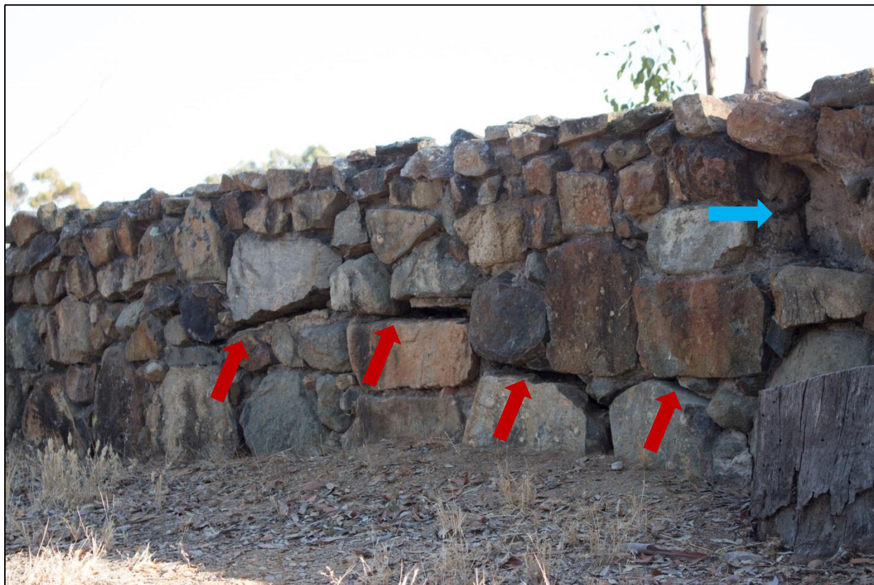
Figure 19. Detail view of above wall section showing large crack (red arrows) and a missing cobblerstone (blue arrow) (Photo credit: Dudek).
