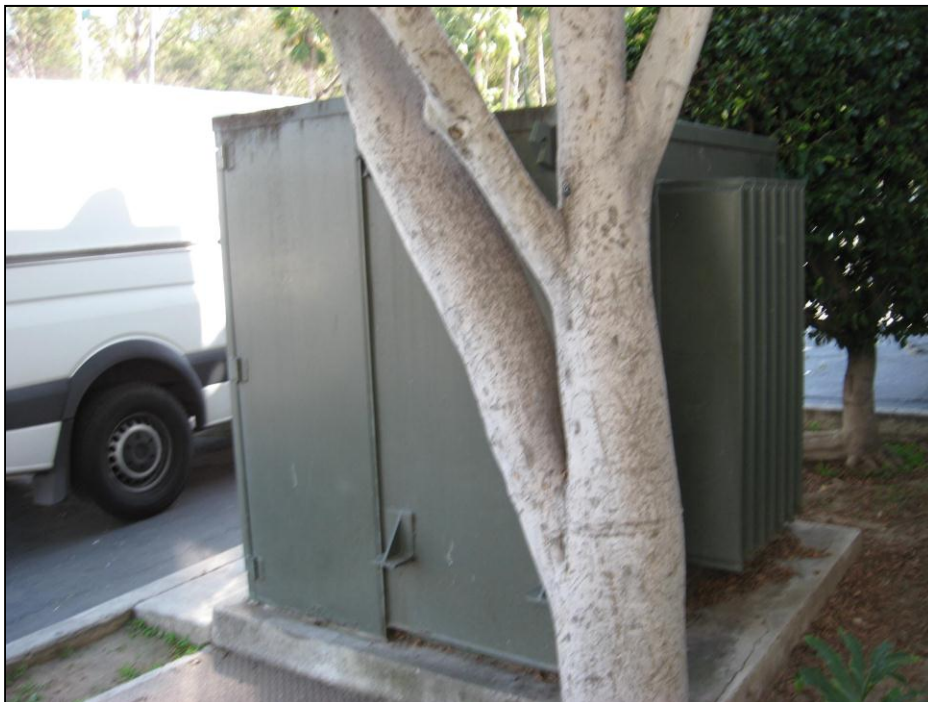
Photograph #30 Finned transformer east of building 1.
