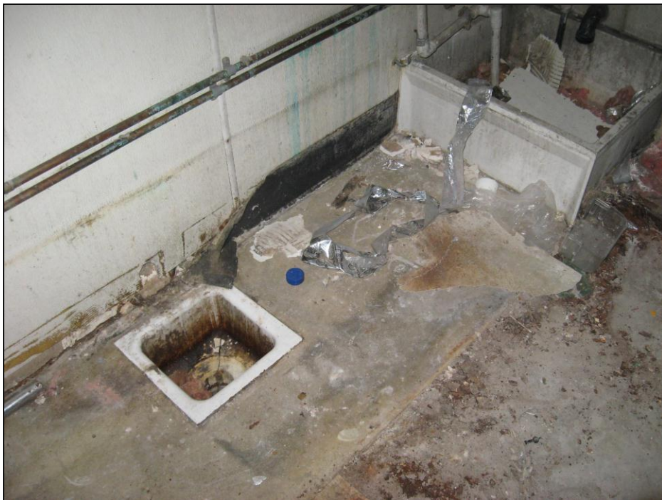
Photograph #28 Floor drains in cleaning room of vacant health club.
