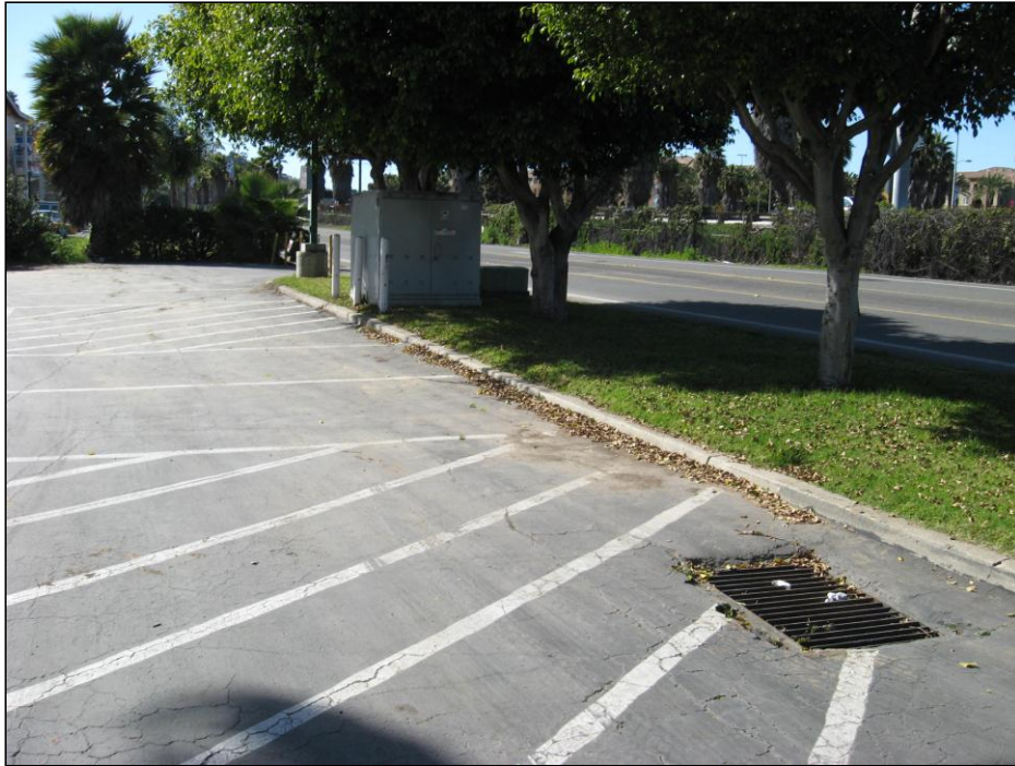
Photograph #11 Storm Drain inlet and pad mounted transformer on northwest corner of the Site.
