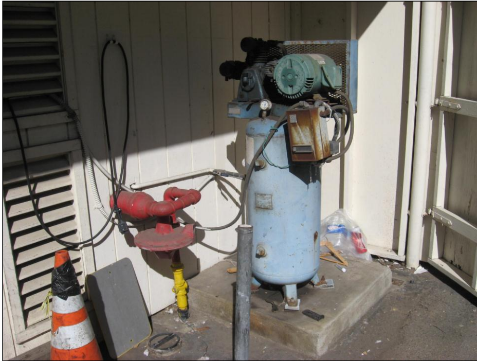
Photograph #23 Air compressor with de minimis staining behind maintenance building.
