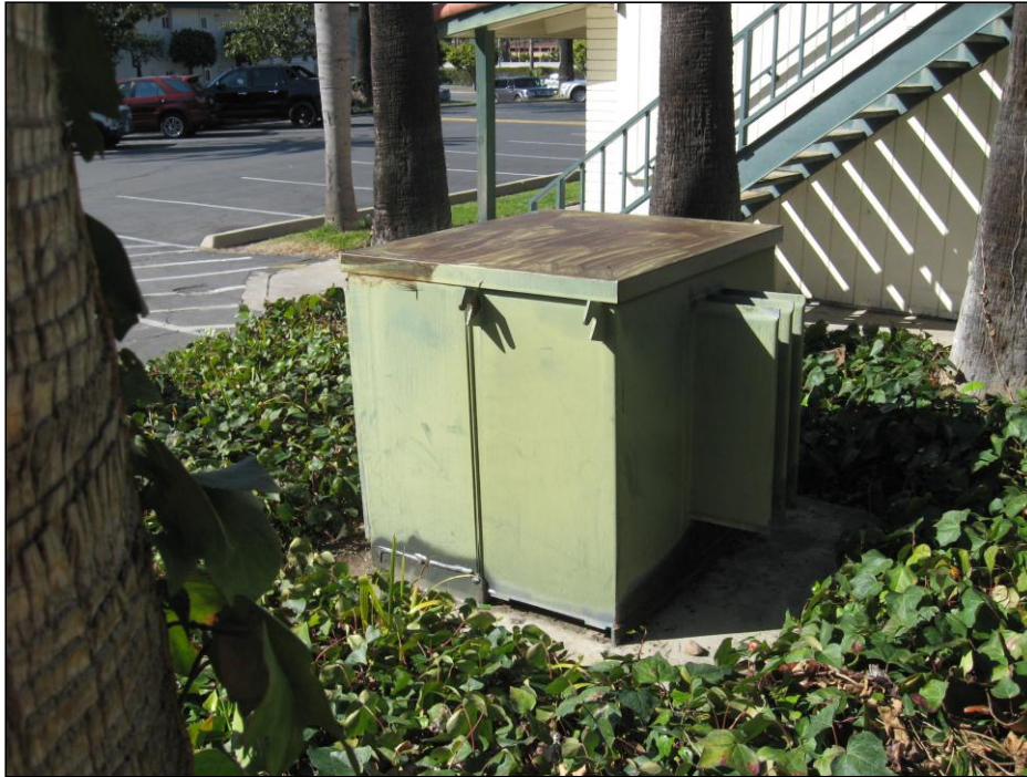
Photograph #29 Finned transformer south of Building 4.
