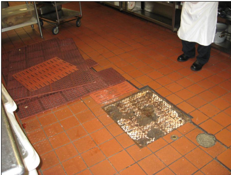
Photograph #8 Grease trap in restaurant kitchen.
