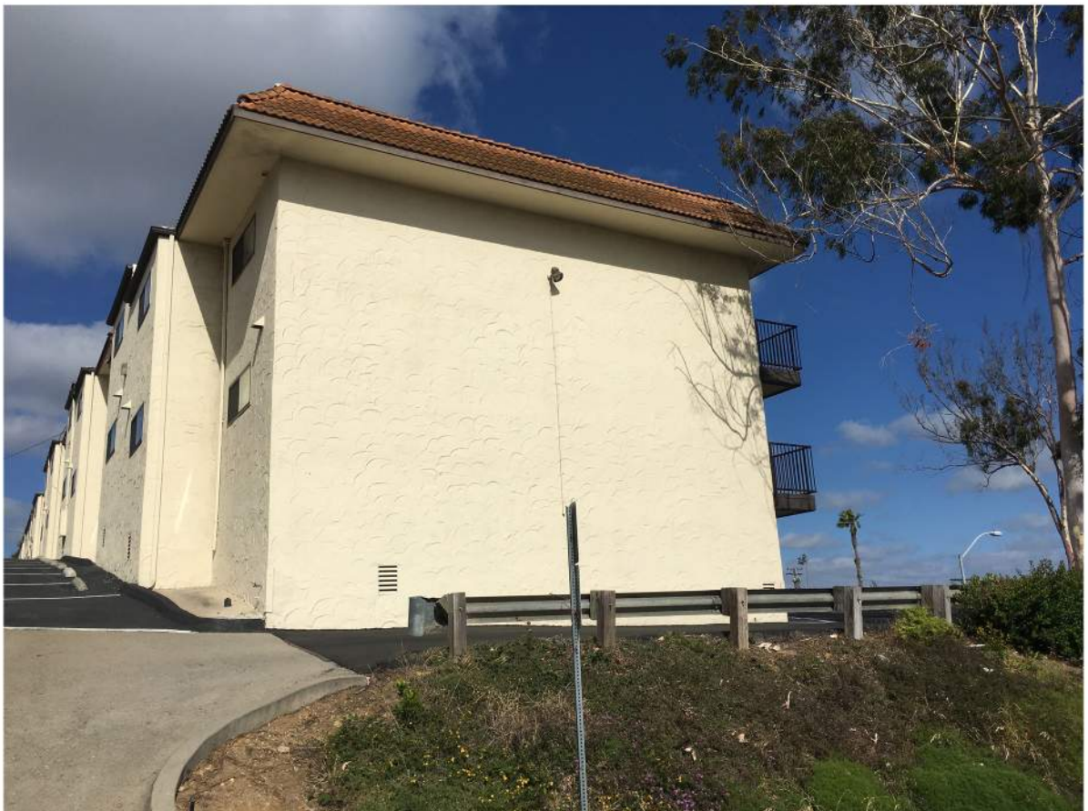
Presidio Terrace Apts - West Elevation.JPG
