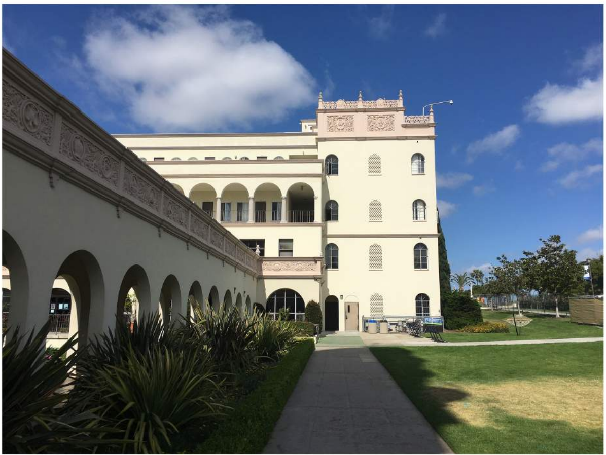
Maher Hall - West Elevation-01.JPG
