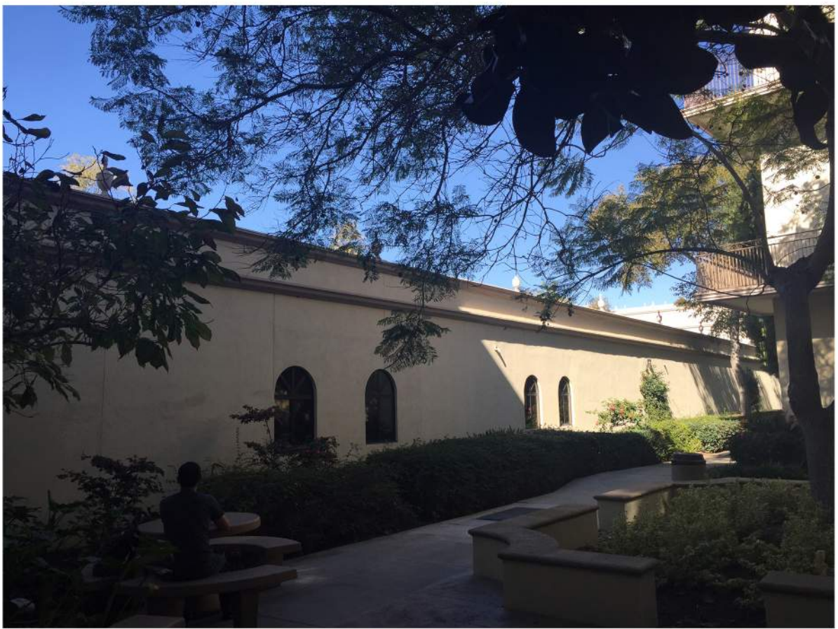
Loma Hall East Elevation-02.JPG
