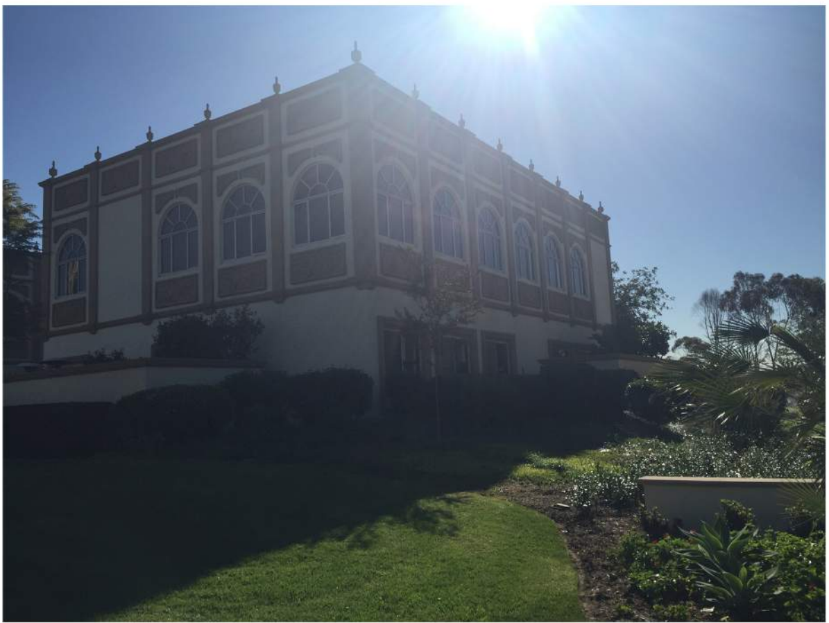
Hahn School West Elevation-01.JPG
