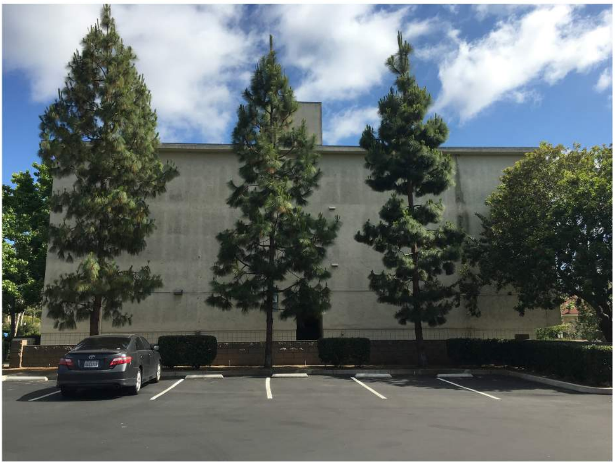
San Antonio de Padua - East Elevation-01.JPG
