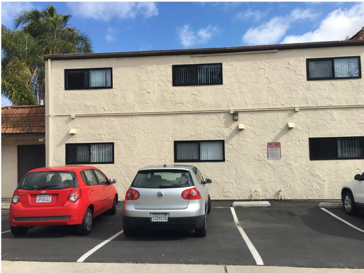
Presidio Terrace Apts - North Elevation-01.JPG
