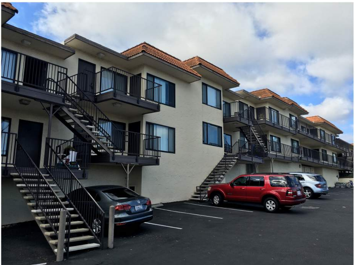
Presidio Terrace Apts - South Elevation-01.JPG
