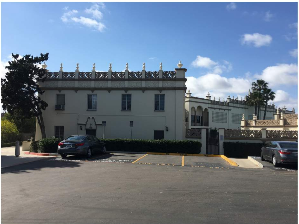
Sports Center - South Elevation.JPG
