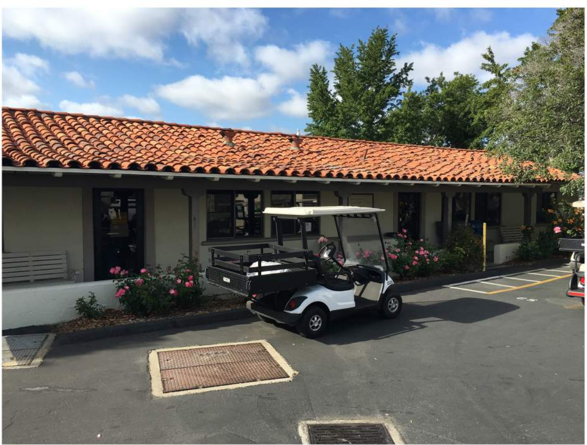
Facilities Management - South Elevation-01.JPG
