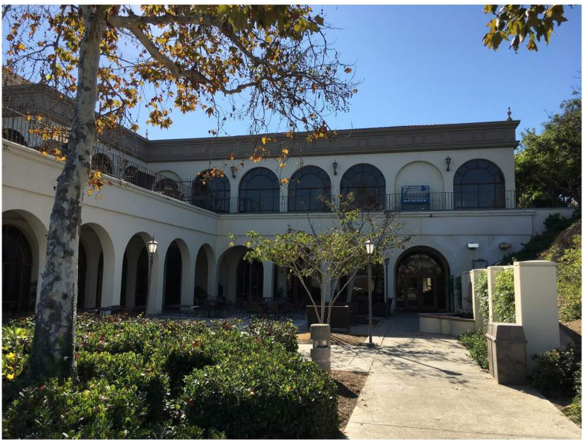
University Center - West Elevation-01.JPG
