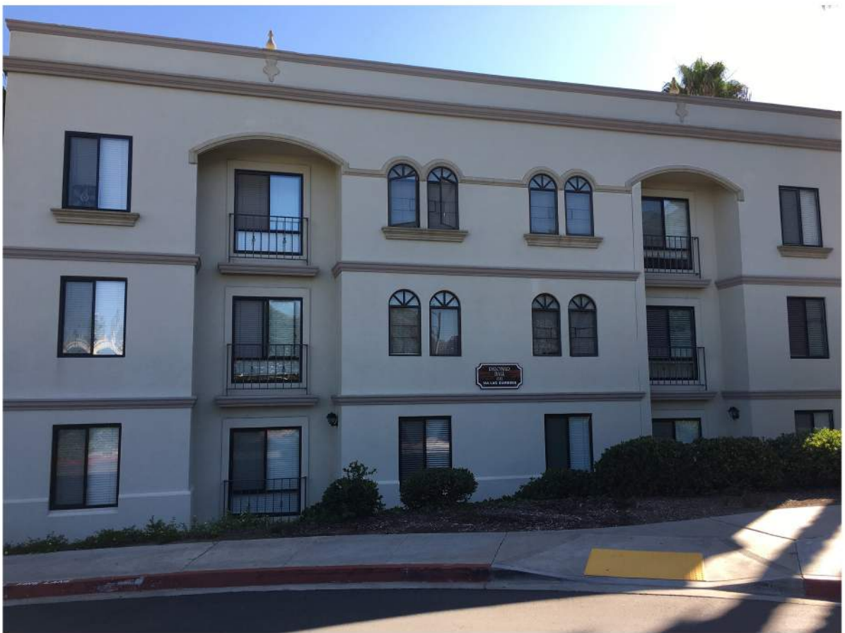
Alcala Vista Apts - Typical Front Elevation-02.JPG
