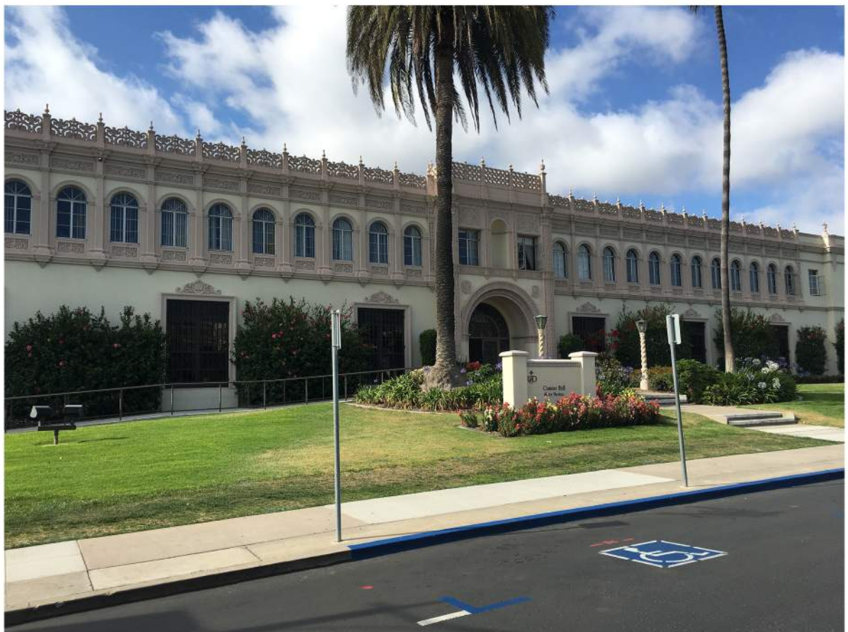
Camino Hall - South Elevation-01.JPG
