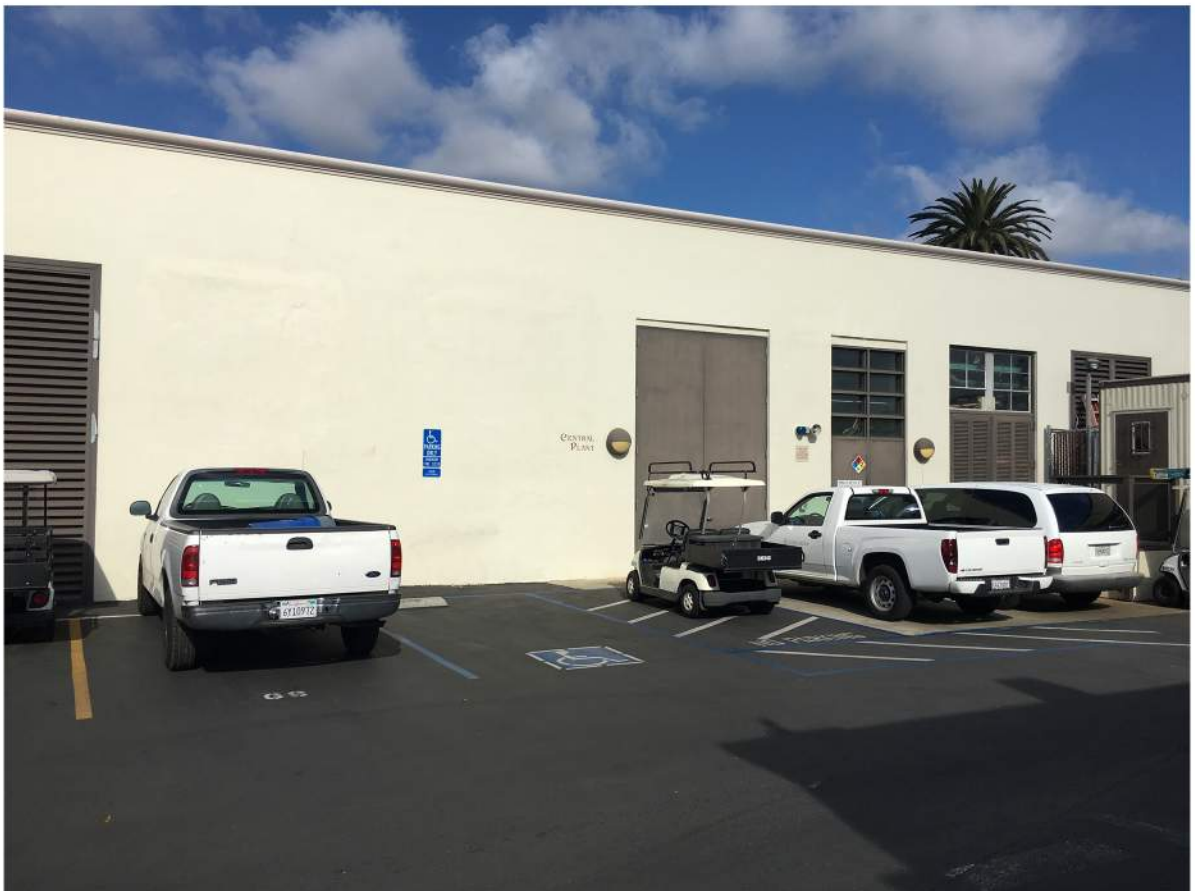
Central Utility Plant - West Elevation.JPG
