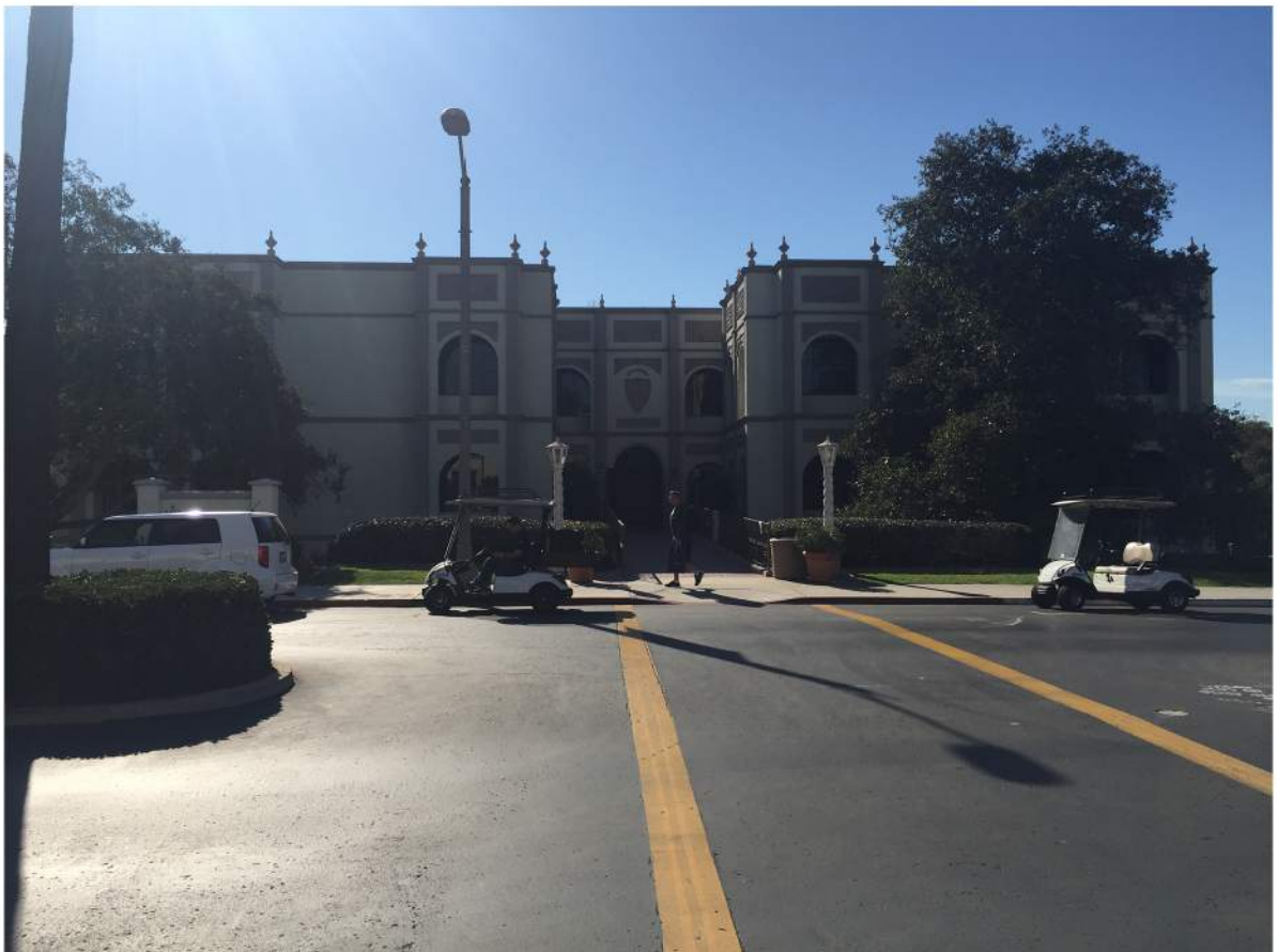
Olin Hall - North Elevation.JPG
