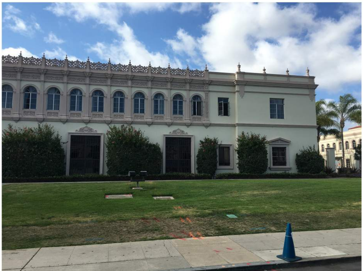
Camino Hall - South Elevation-03.JPG
