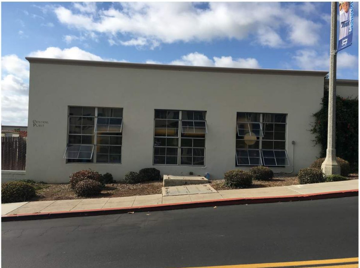
Central Utility Plant - South Elevation-01.JPG
