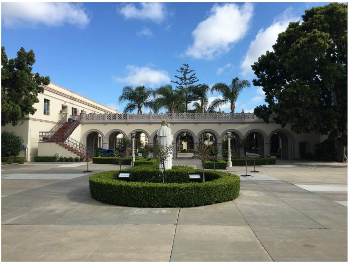
Camino Founders Hall Courtyard North Elevation.JPG
