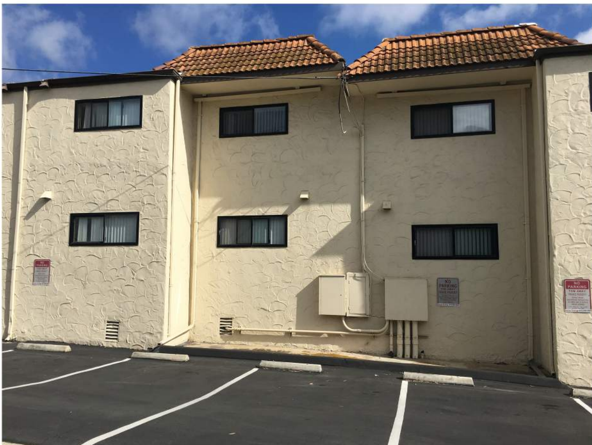
Presidio Terrace Apts - North Elevation-02.JPG
