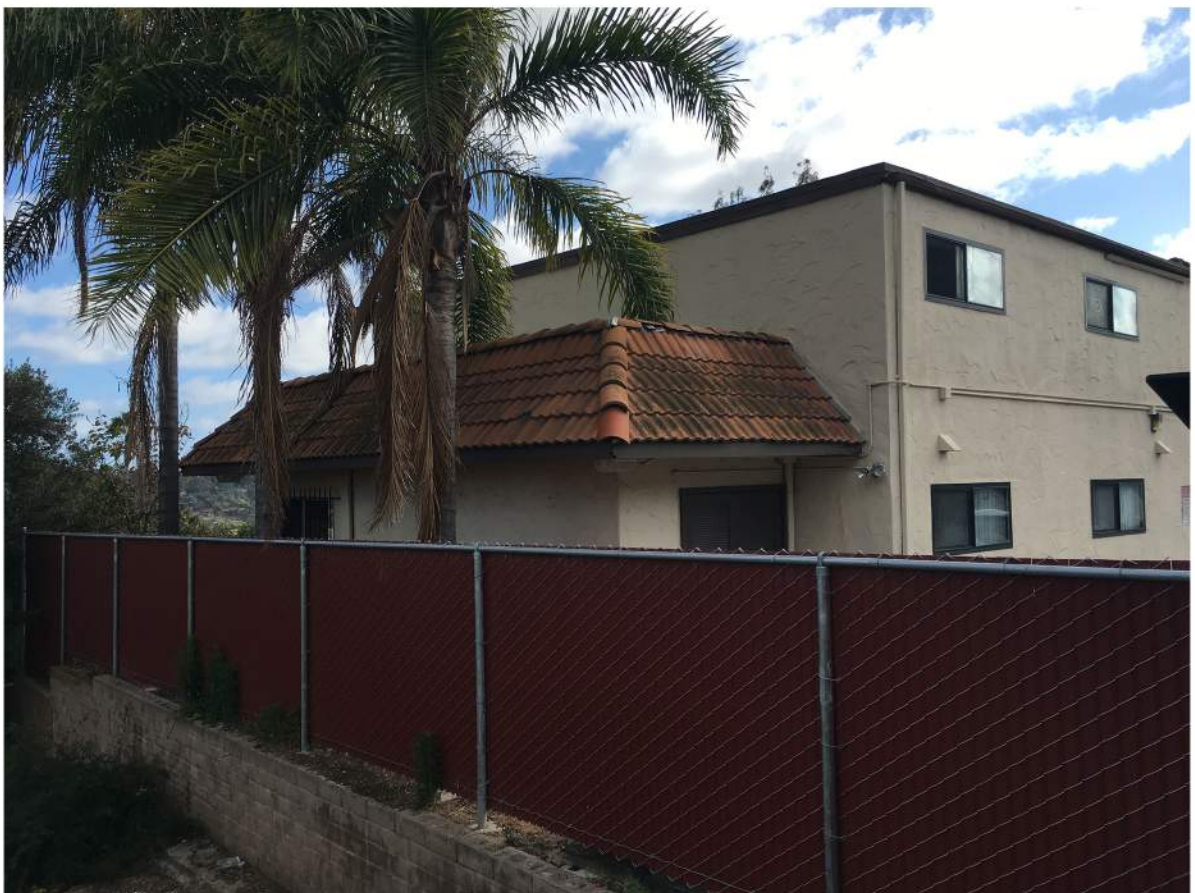
Presidio Terrace Apts - East Elevation.JPG
