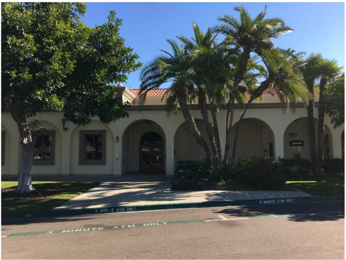
University Center - West Elevation-03.JPG
