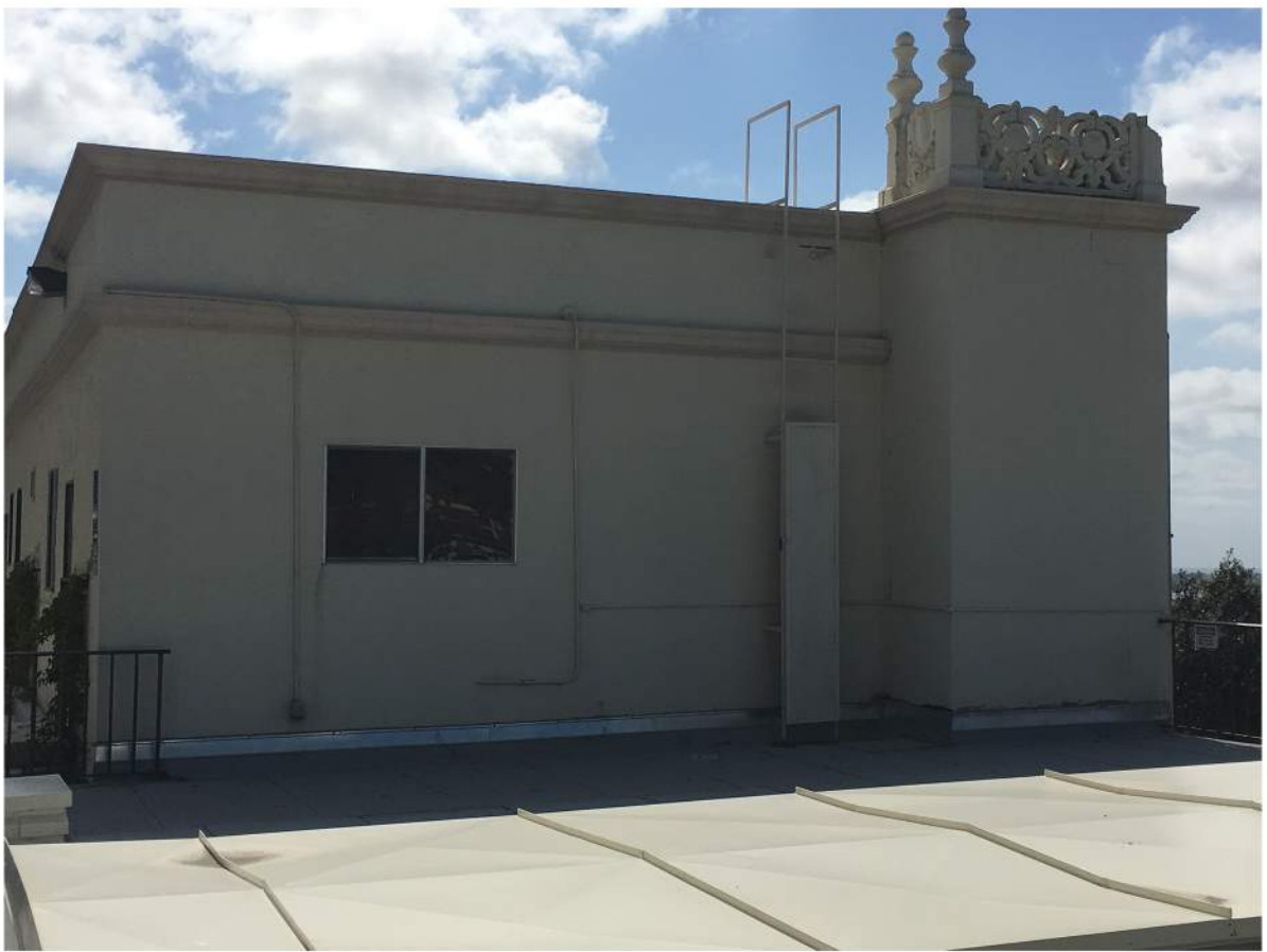
Print Shop - East Elevation.JPG
