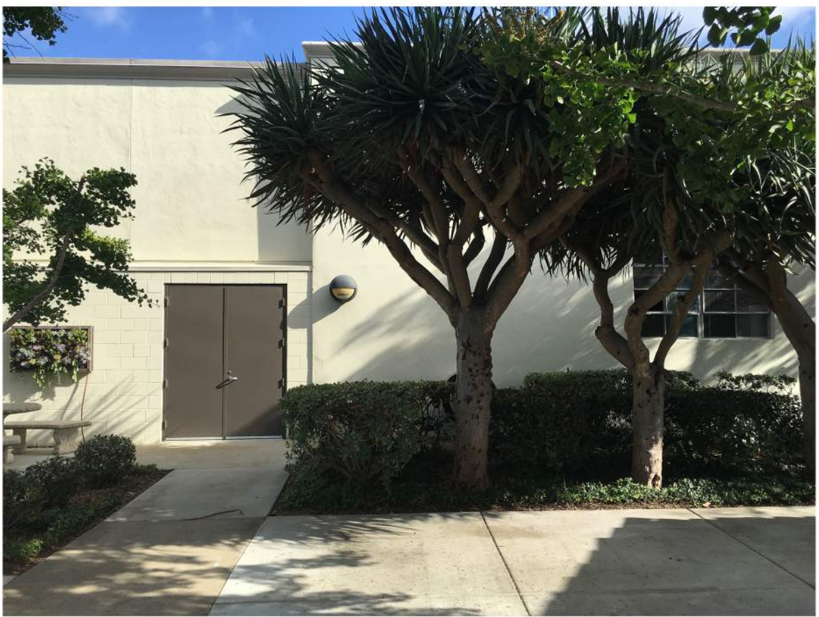
Central Utility Plant - South Elevation-02.JPG
