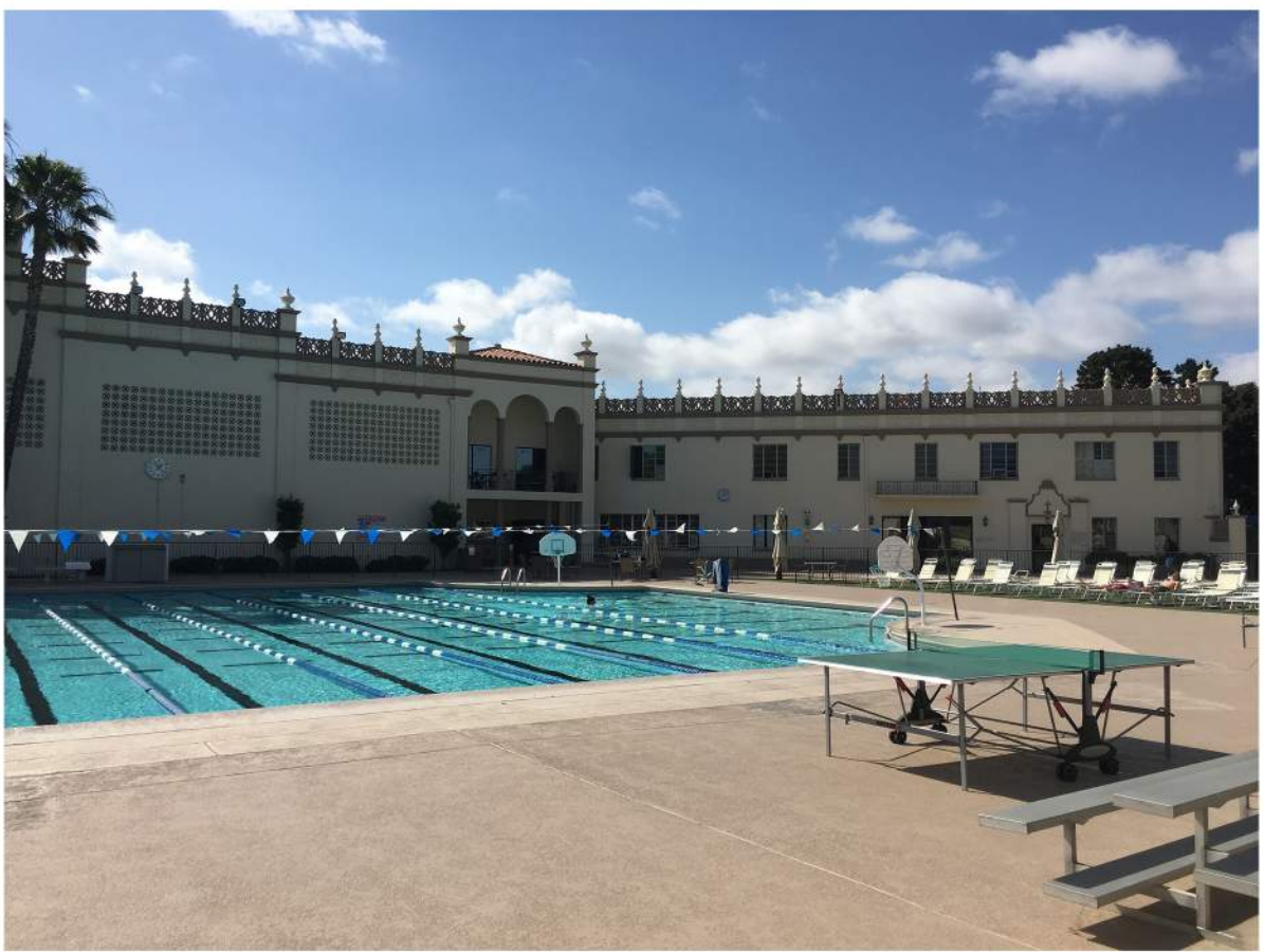
Sports Center - East Elevation-02.JPG
