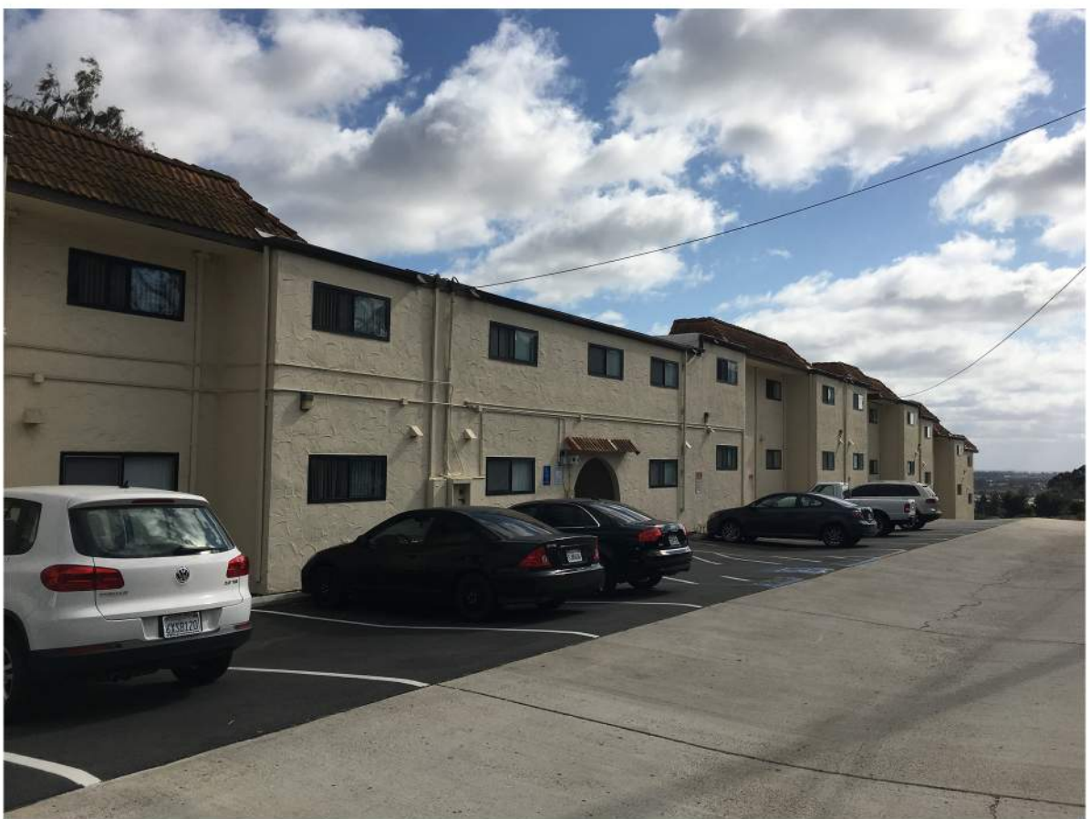
Presidio Terrace Apts - North Elevation-03.JPG
