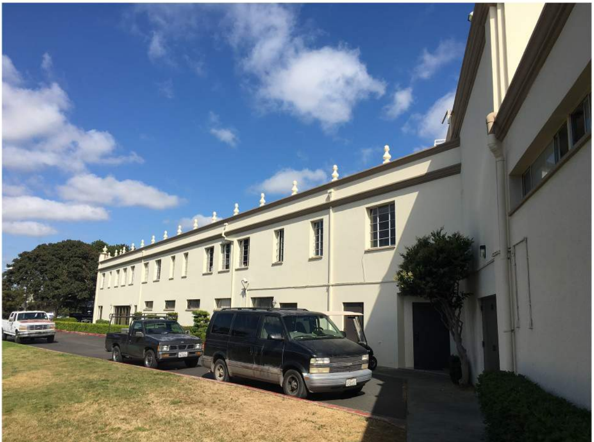
Sports Center - North Elevation-02.JPG
