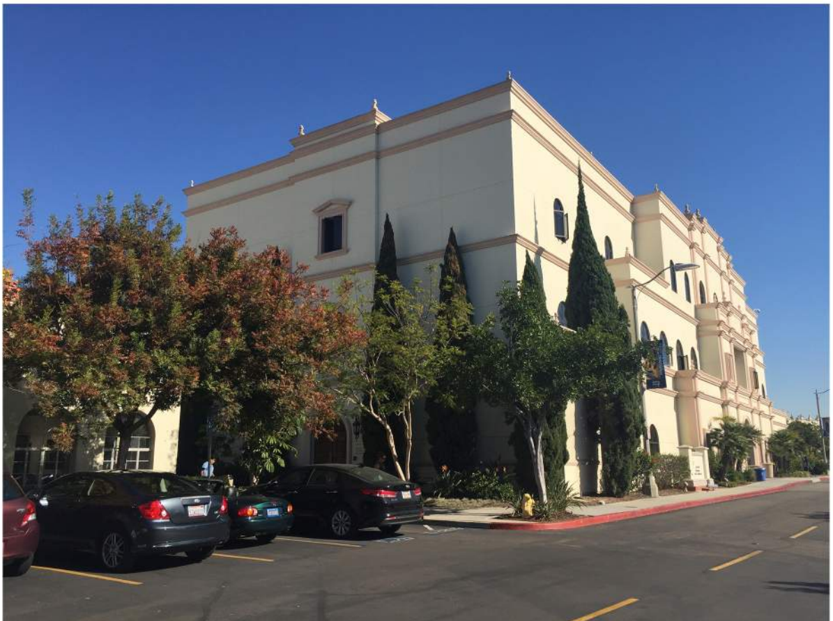
Loma Hall West Elevation-01.JPG
