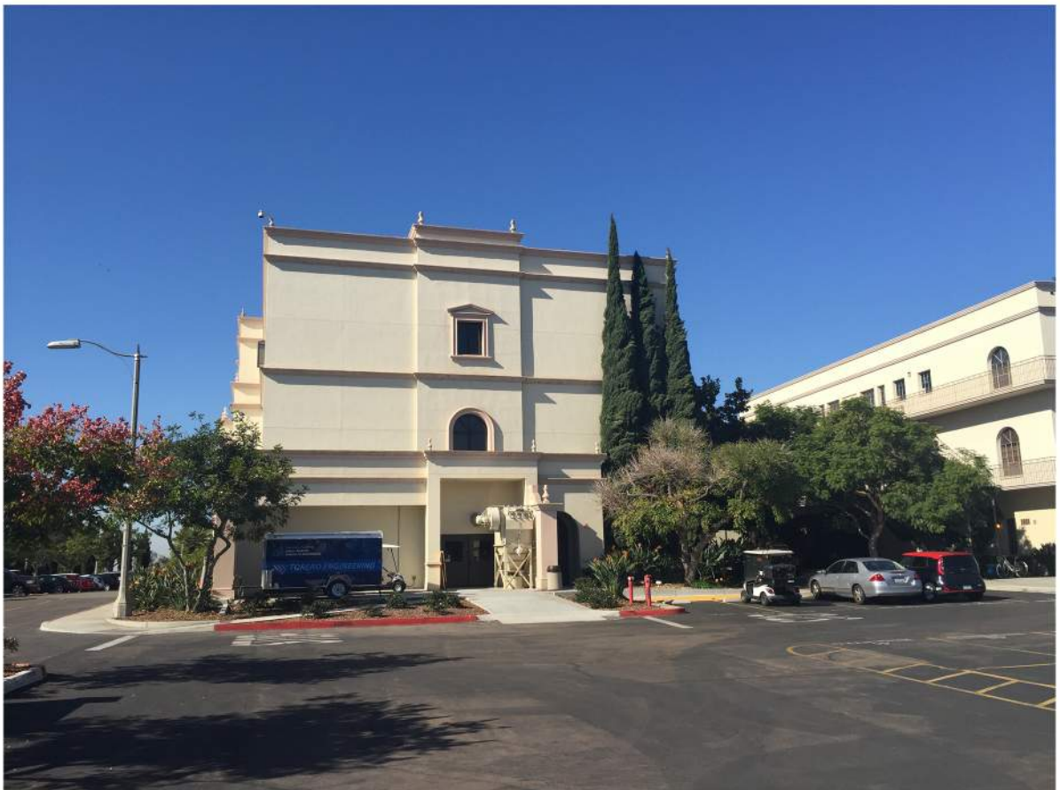
Loma Hall - East Elevation-01.JPG
