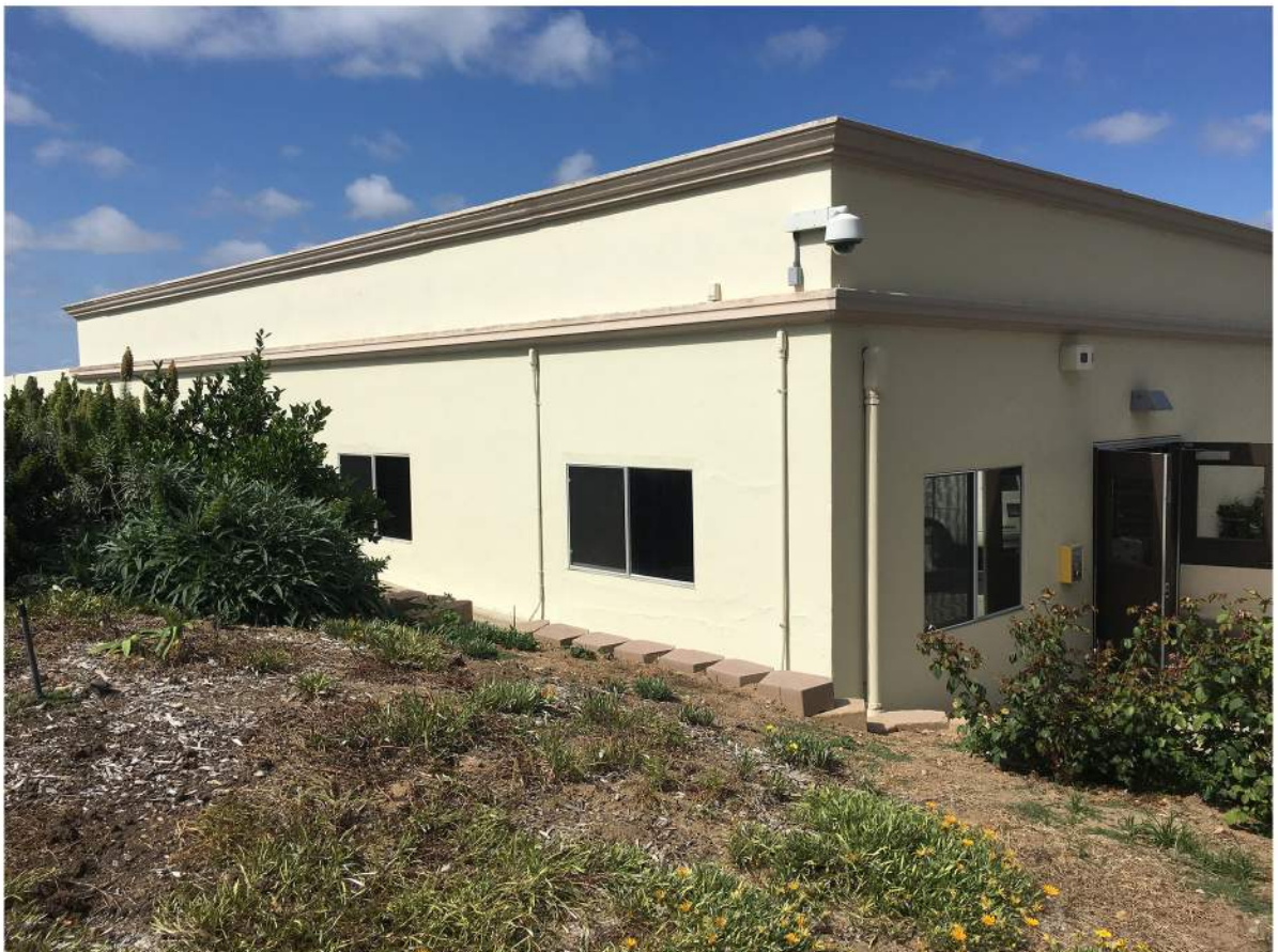
Print Shop - West Elevation.JPG
