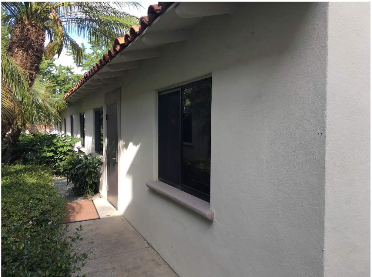
Facilities Management - North Elevation.JPG
