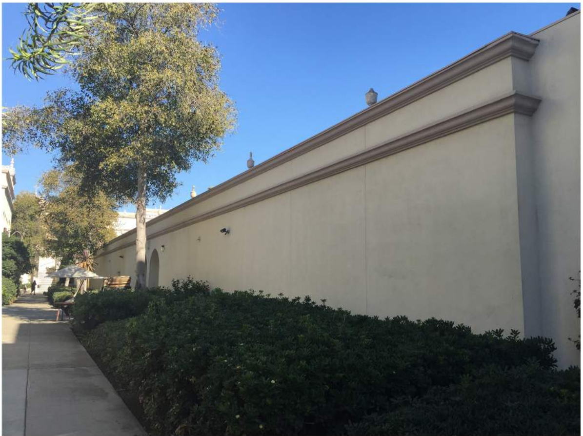
Loma Hall West Elevation-02.JPG
