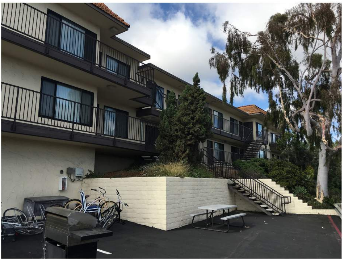
Presidio Terrace Apts - South Elevation-02.JPG
