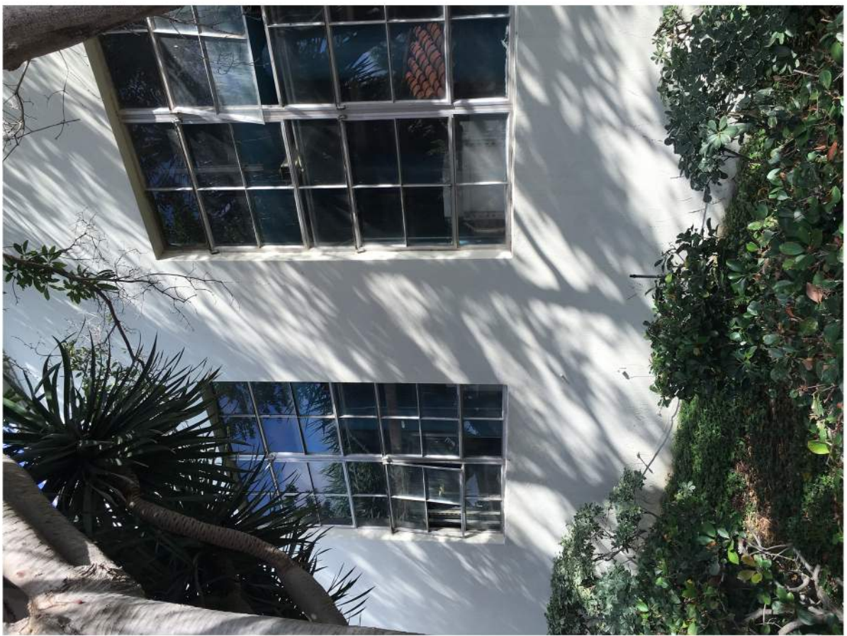
Central Utility Plant - North Elevation.JPG
