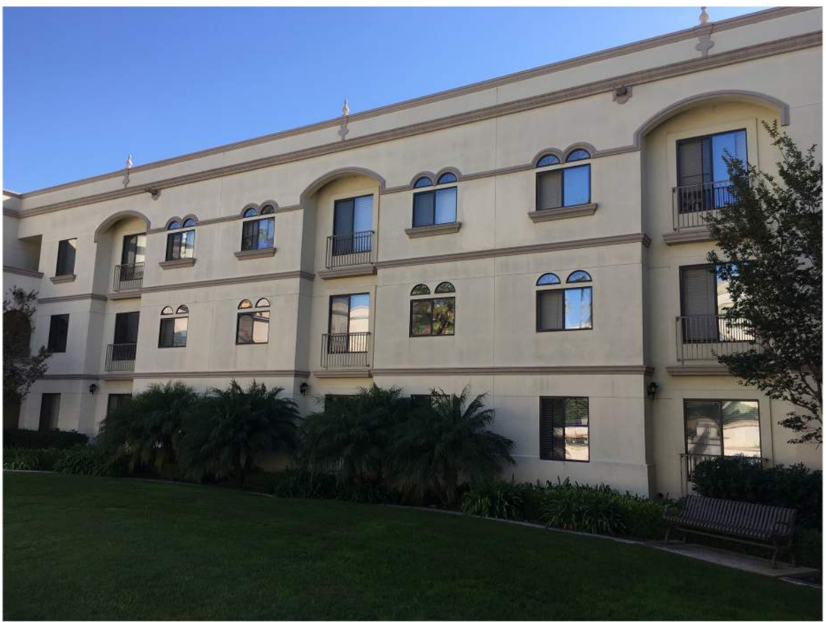
Alcala Vista Apts - Typical Rear Elevation-01.JPG
