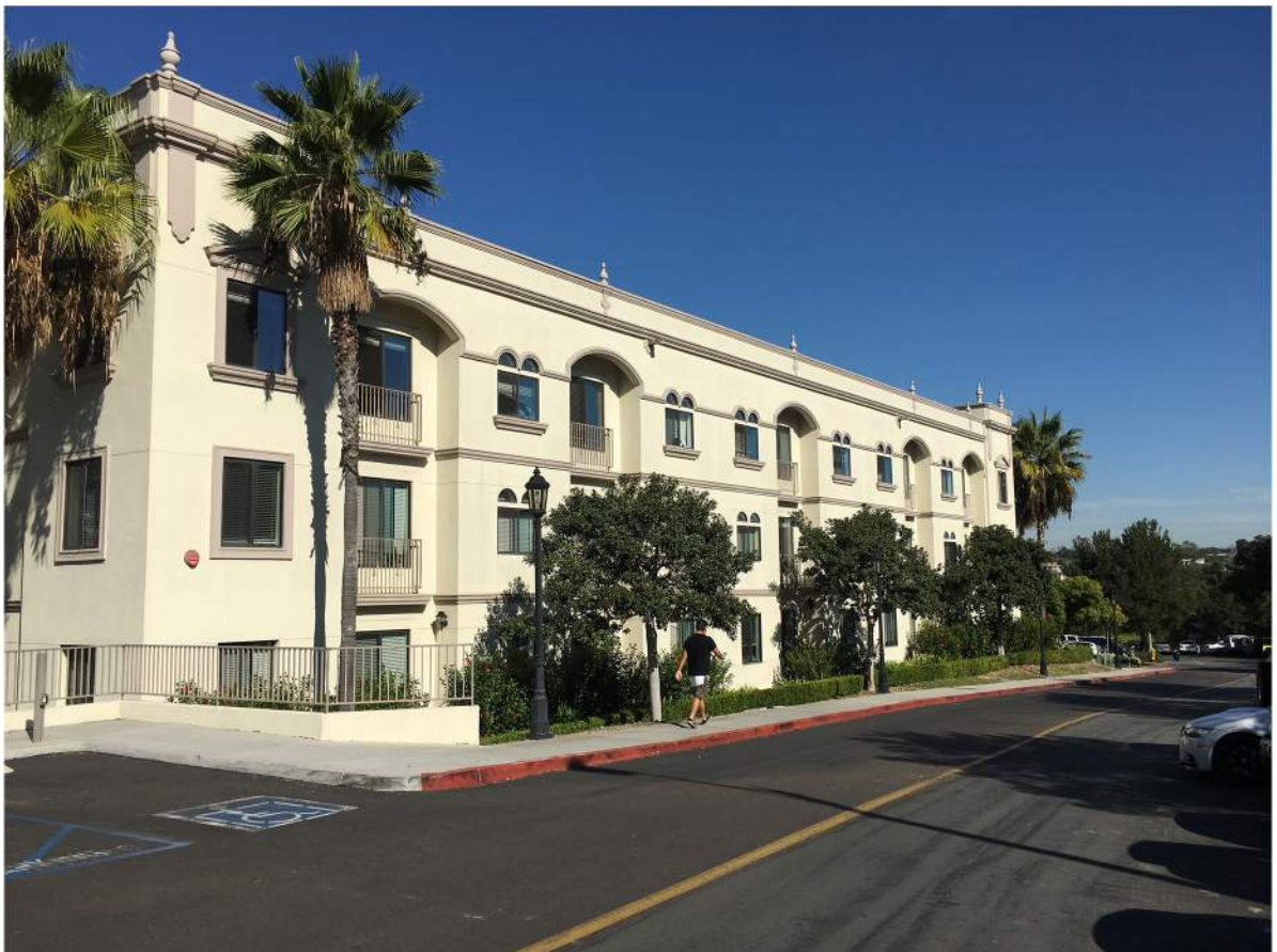
Alcala Vista Apts - Typical Rear Elevation-02.JPG
