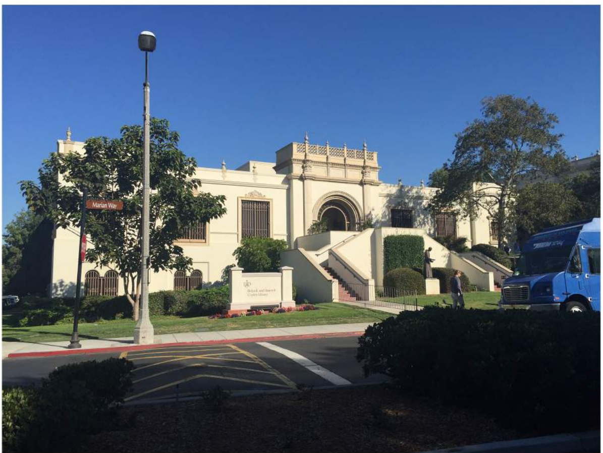
Copley Library South Elevation.JPG
