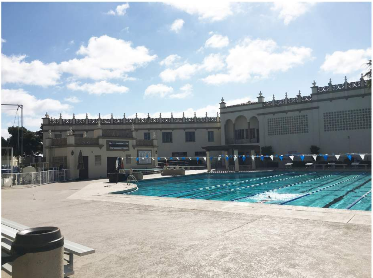
Sports Center - East Elevation-03.JPG
