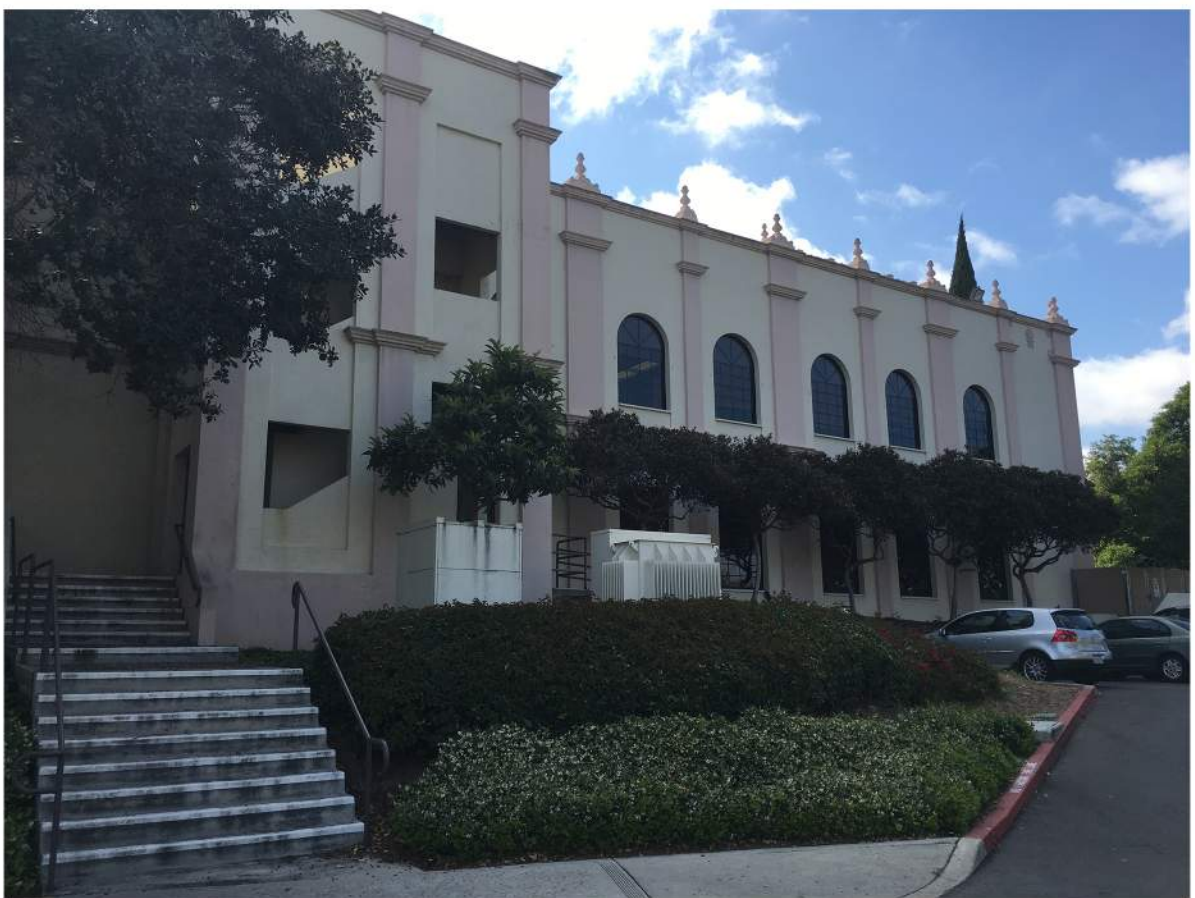
Pardee LRC - South Elevation.JPG
