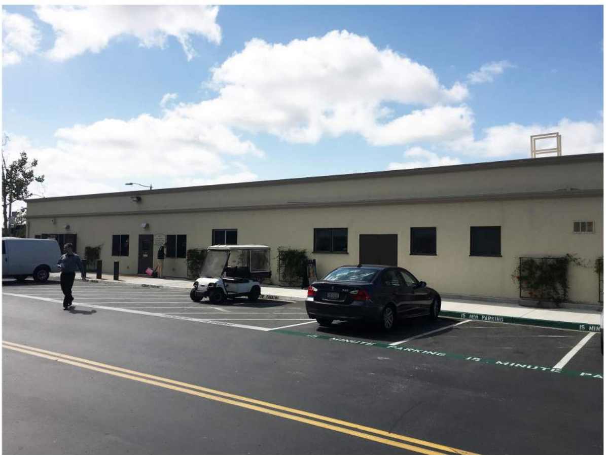
Print Shop - South Elevation.JPG
