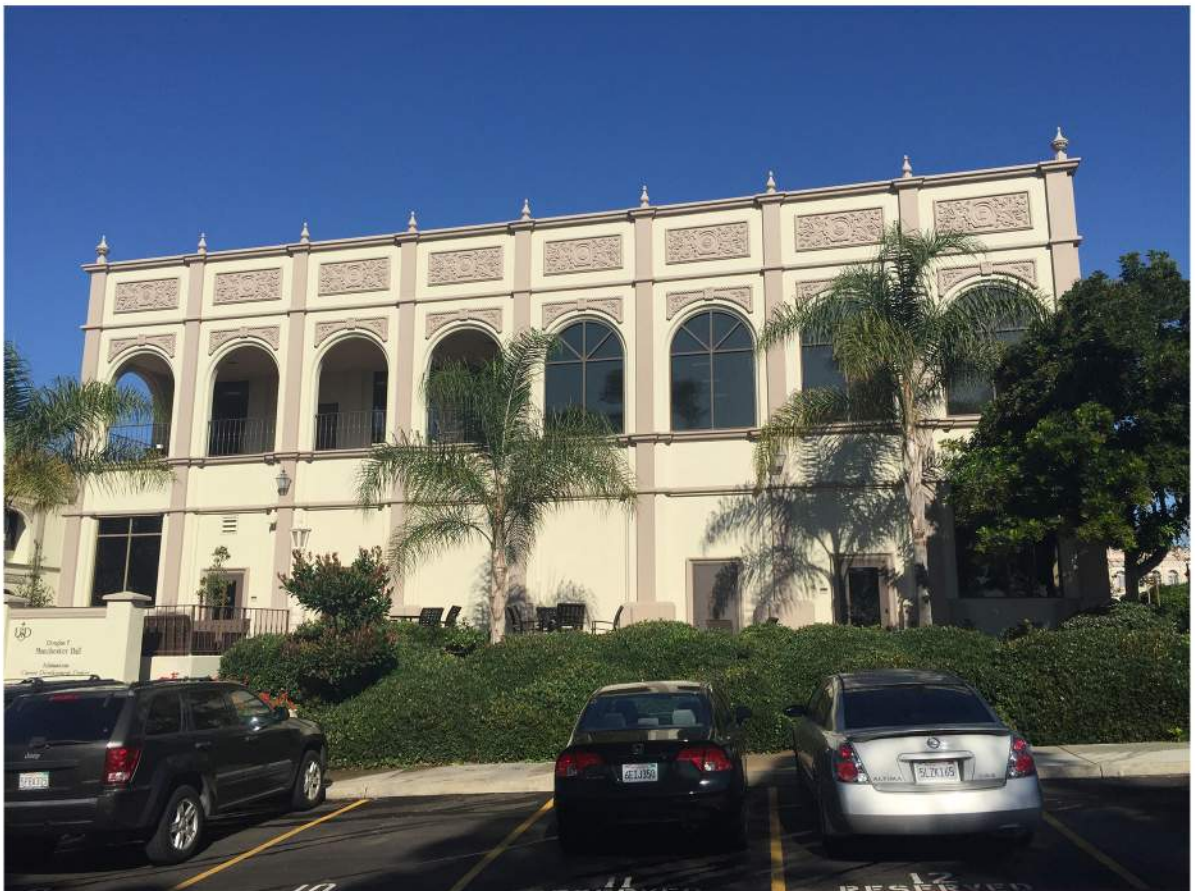
Manchester Conf Ctr - East Elevation.JPG
