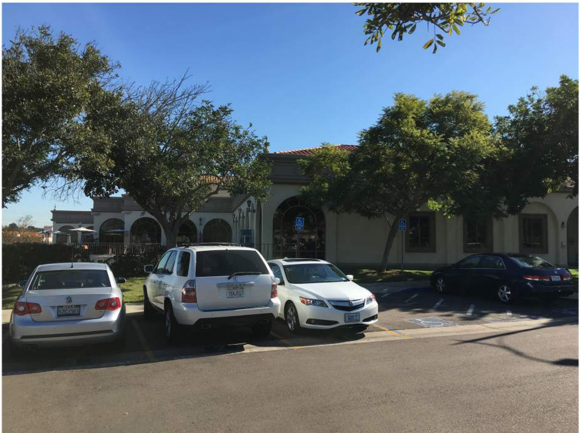
University Center - West Elevation-02.JPG
