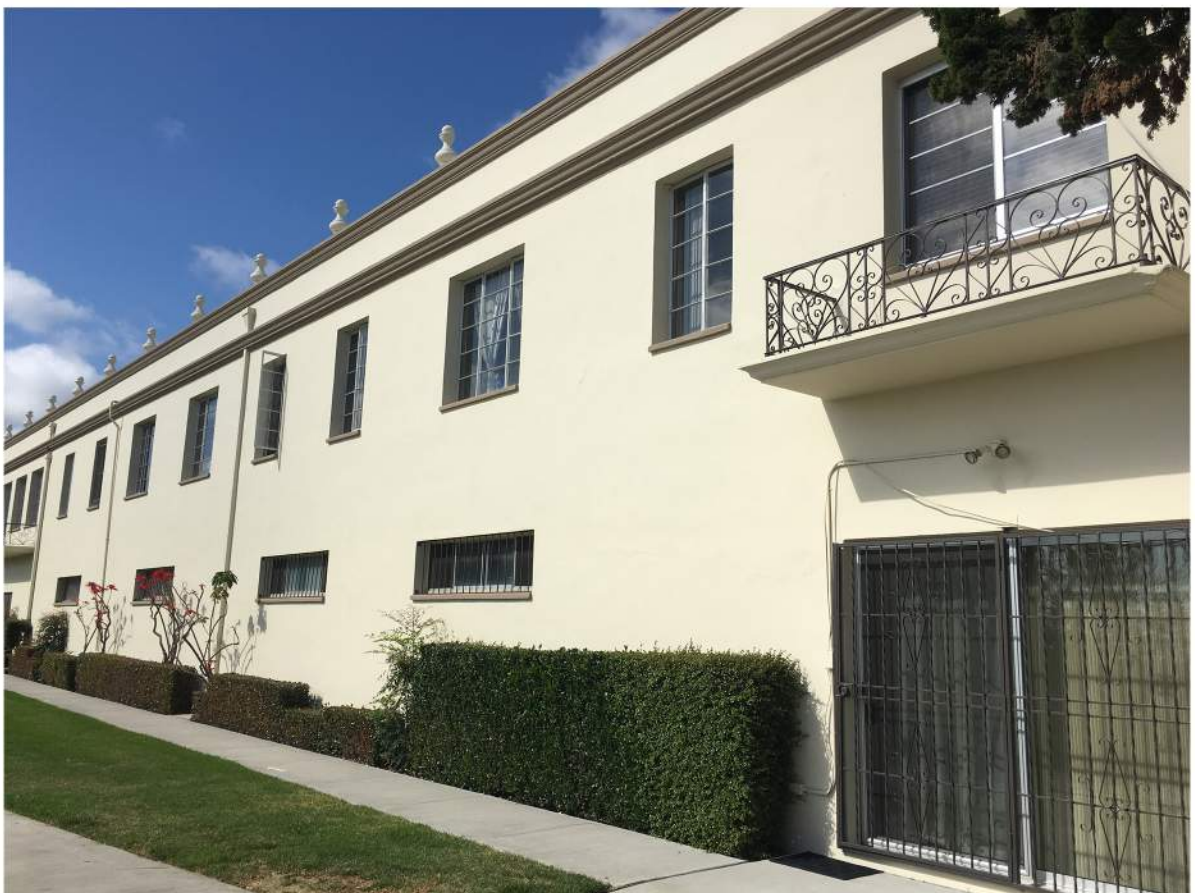
Sports Center - West Elevation-01.JPG
