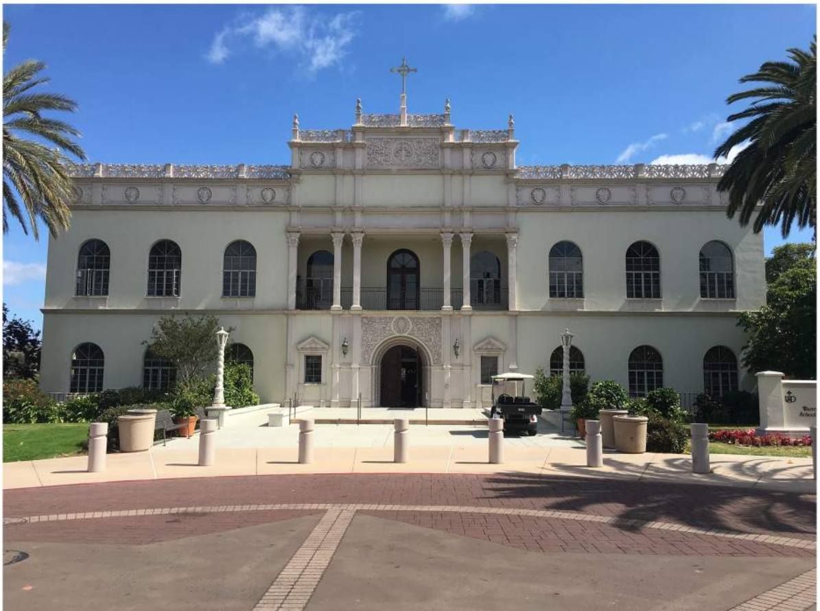
Warren Hall - North Elevation.JPG
