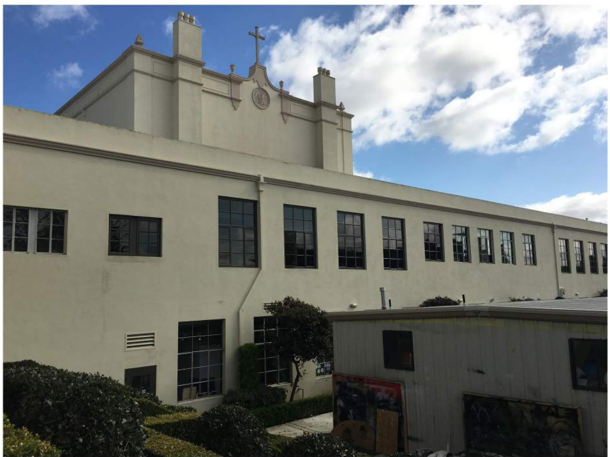
Camino Hall - North Elevation-04.JPG
