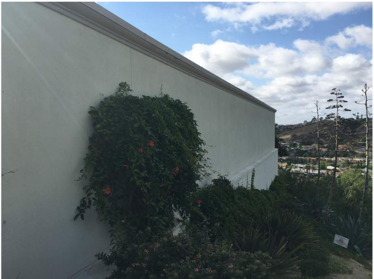
Central Utility Plant - East Elevation.JPG
