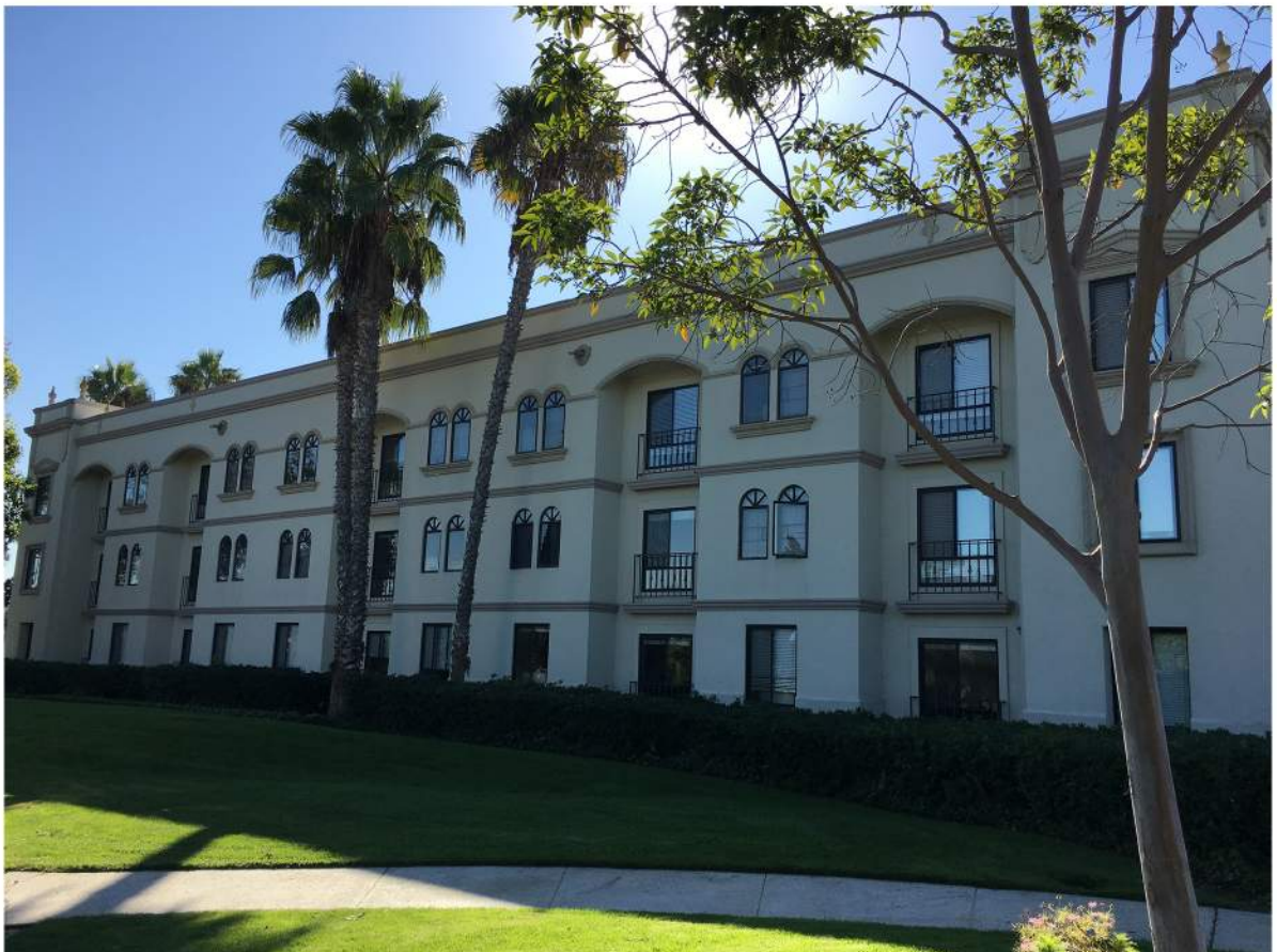
Alcala Vista Apts - Typical Front Elevation-01.JPG
