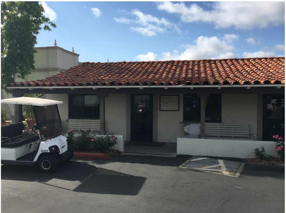
Facilities Management - South Elevation-02.JPG
