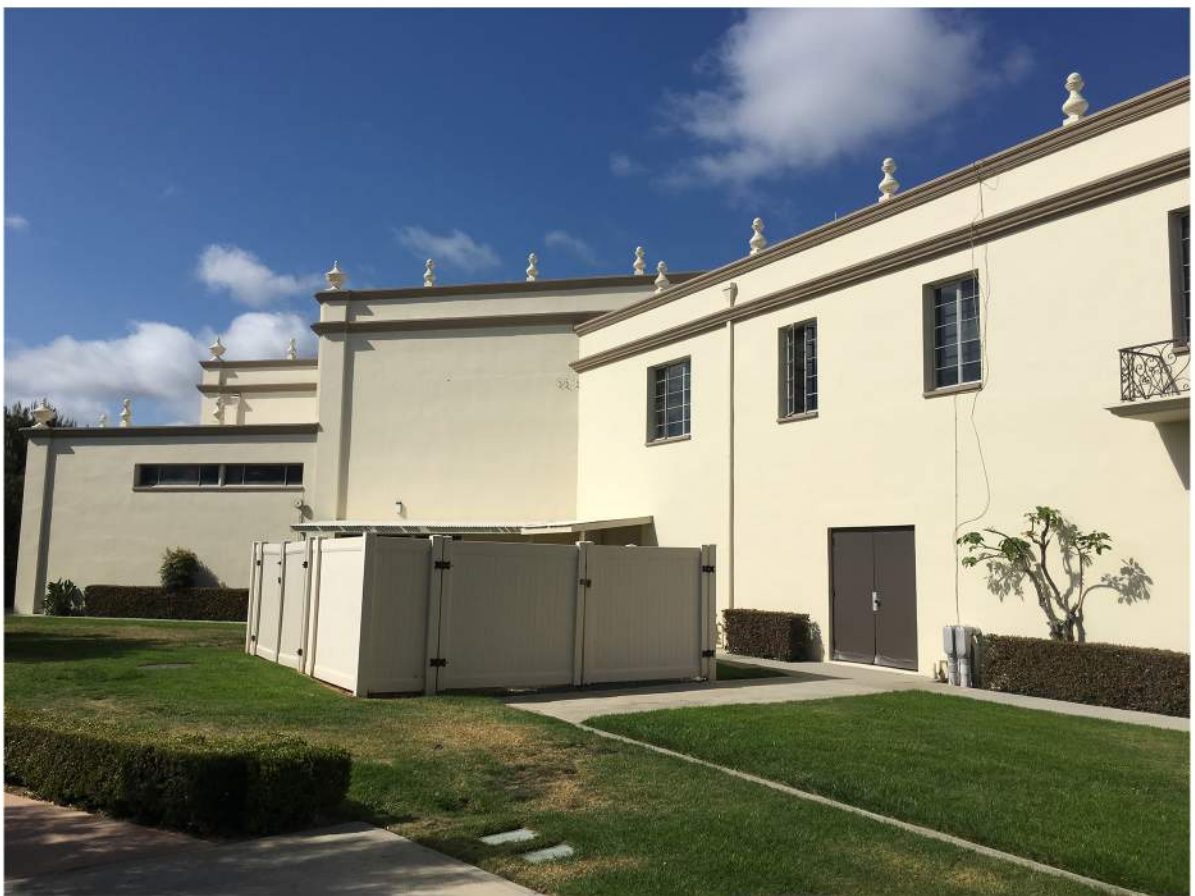
Sports Center - West Elevation-02.JPG
