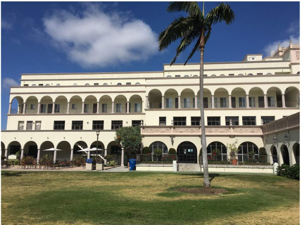
Maher Hall - West Elevation-02.JPG
