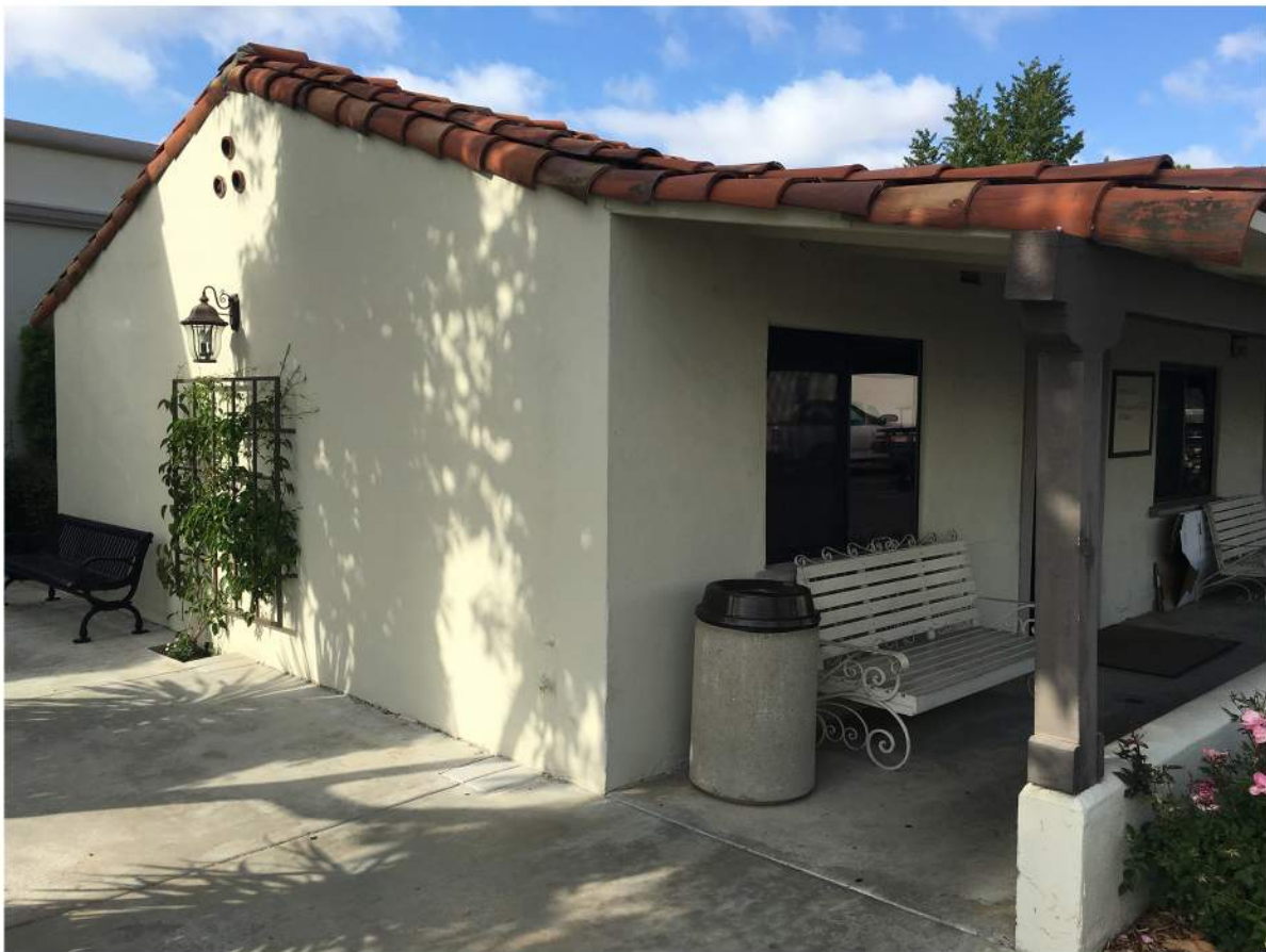
Facilities Management - West Elevation.JPG
