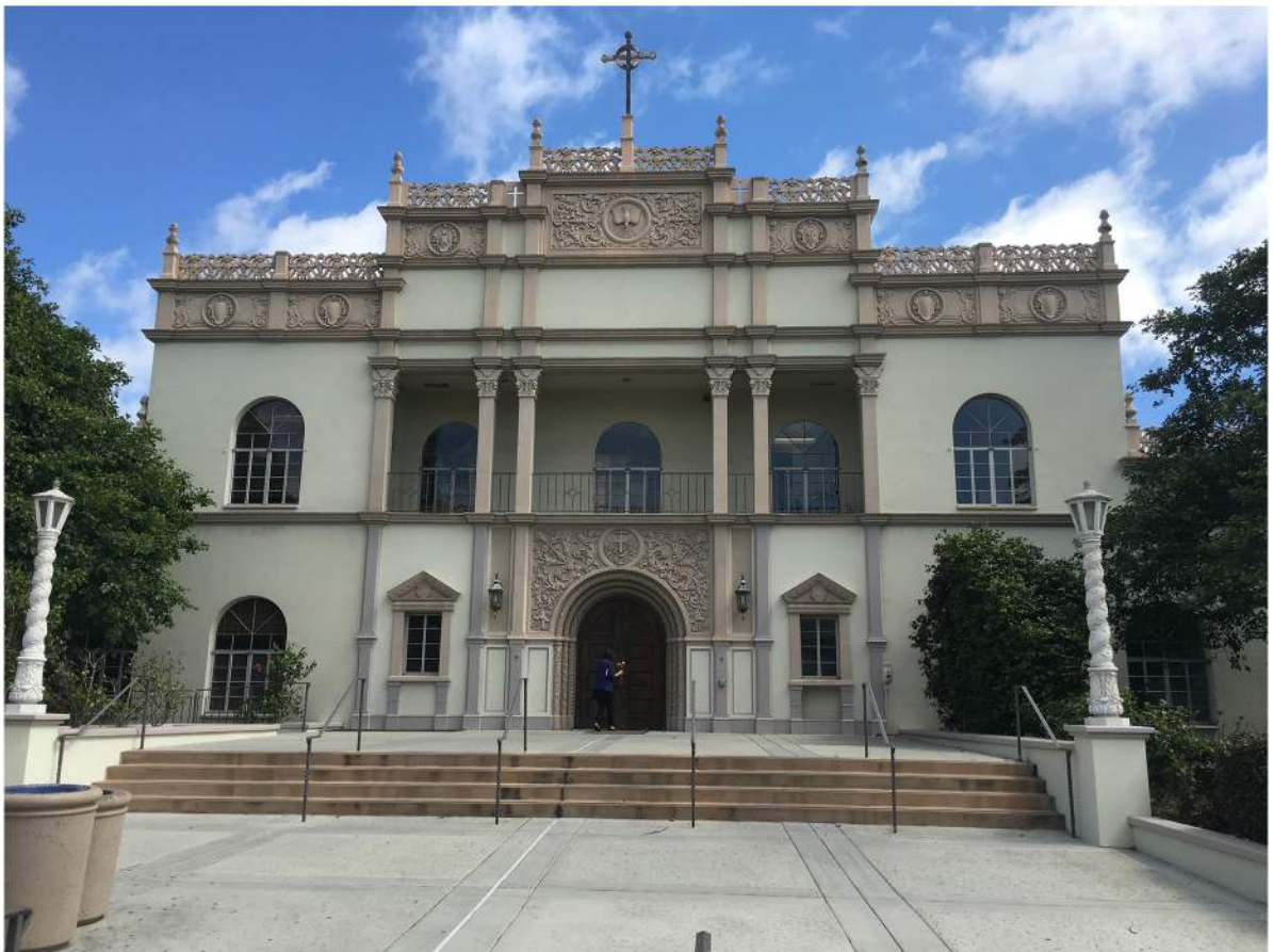
Serra Hall - North Elevation.JPG
