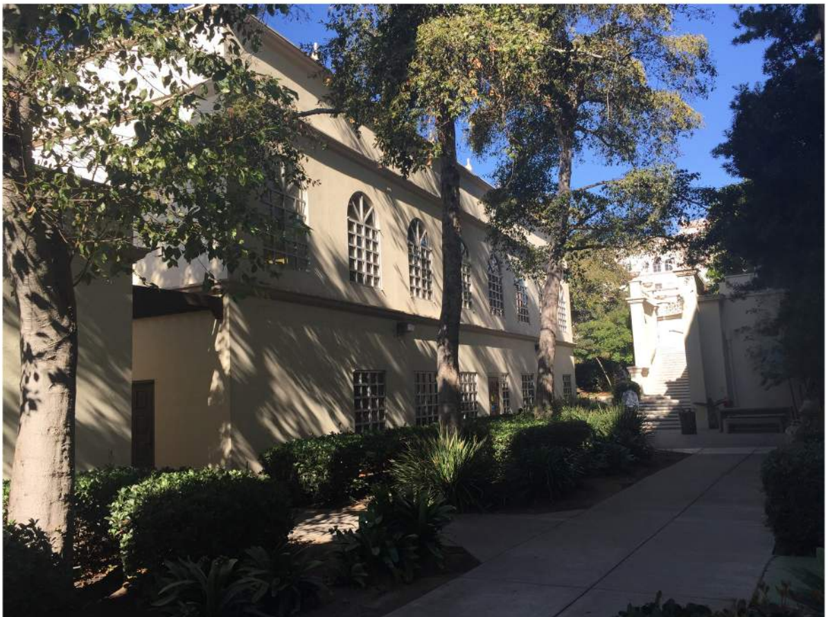
Guadalupe Hall - East Elevation.JPG
