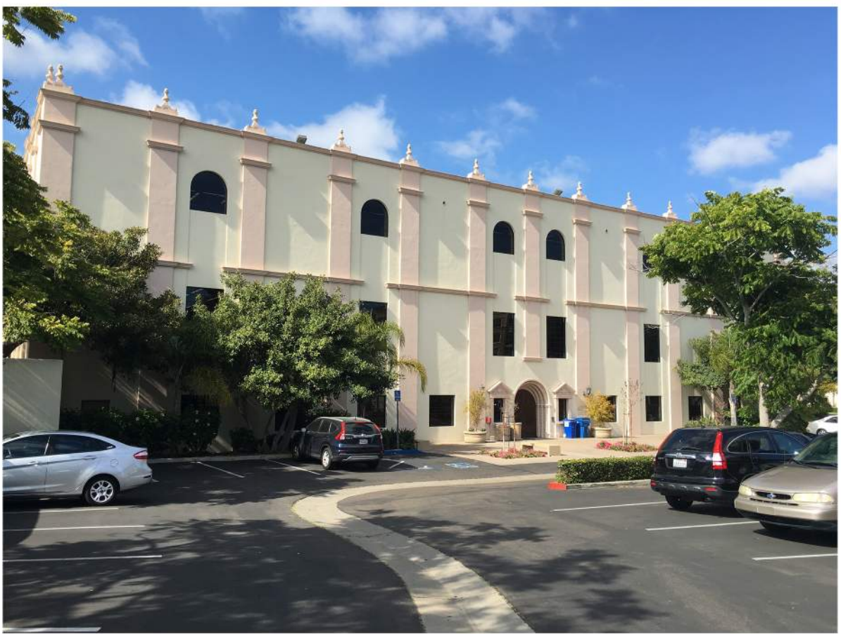
Pardee LRC - East Elevation.JPG
