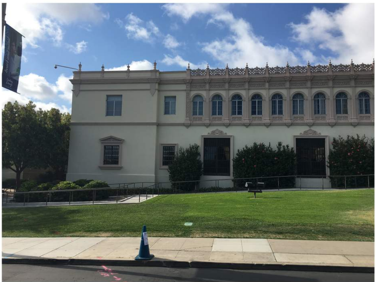
Camino Hall - South Elevation-02.JPG
