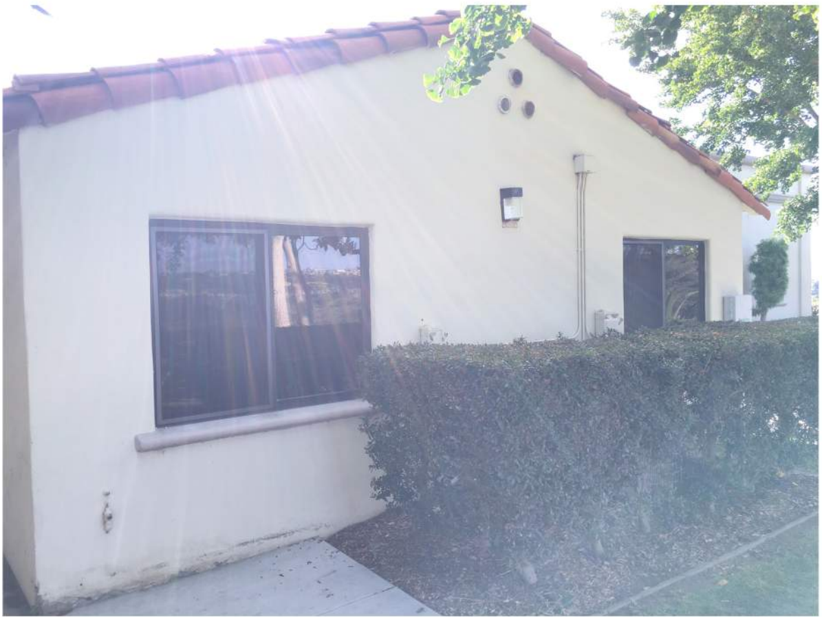
Facilities Management - East Elevation.JPG
