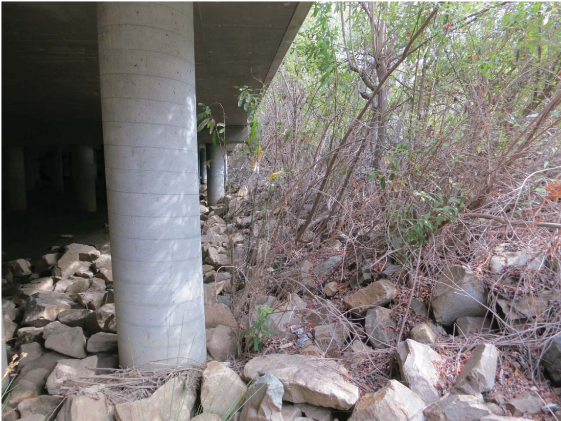
Figure 6. Lower End of Reach 2 at Interstate 5 Bridge
