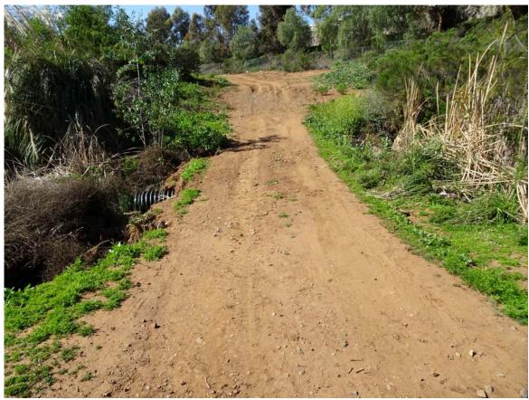
Figure 4. HDPE Pipe and Access Road Grade Control between Reach 1 and 2
