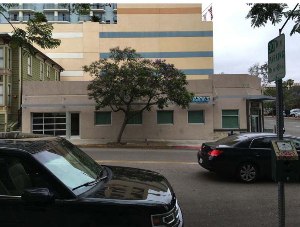
23. EXISTING ON SOUTHWEST CORNER OF CEDAR AND FRONT
