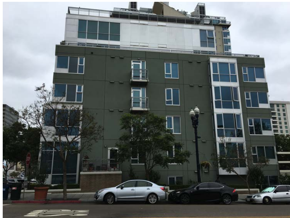
11. LOOKING SOUTH FROM SITE
