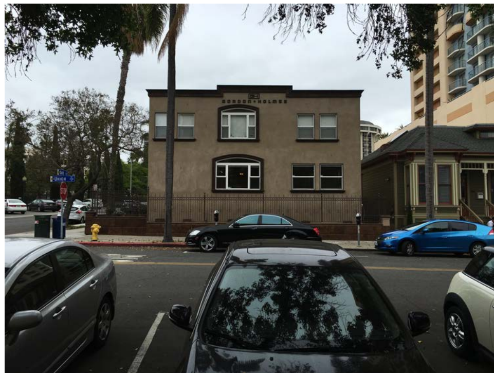
16. SOUTHEAST CORNER OF UNION & DATE
