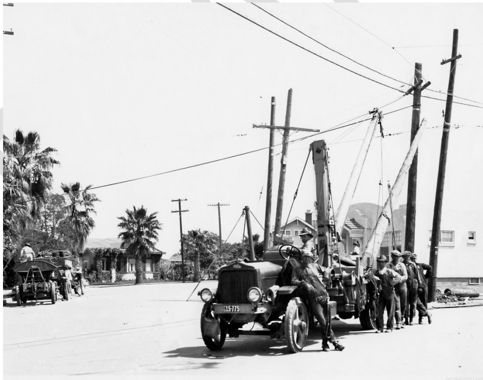
Figure 12. Electrical pole maintenance and replacement on Adams Avenue with Panorama Drive in the background, 1924 (San Diego History Center)
