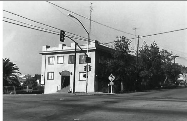
HRB #208-222 - 1830 Market St (note roofline cornice)
