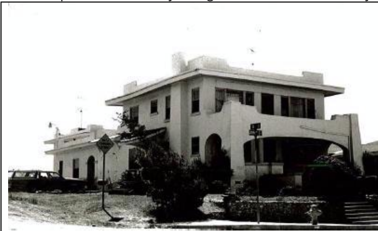
HRB #218 - 643 26 th St (note battered columns)
