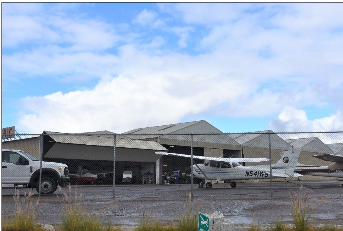
Fig. 11. Pre-engineered aviation hangars belonging to the National Air College and located at Montgomery-Gibbs Executive Airport. Notice the metal siding, flat and gabled roofs, as well as the large sliding and bi-folding hangar doors. IS Architecture, 2018.
