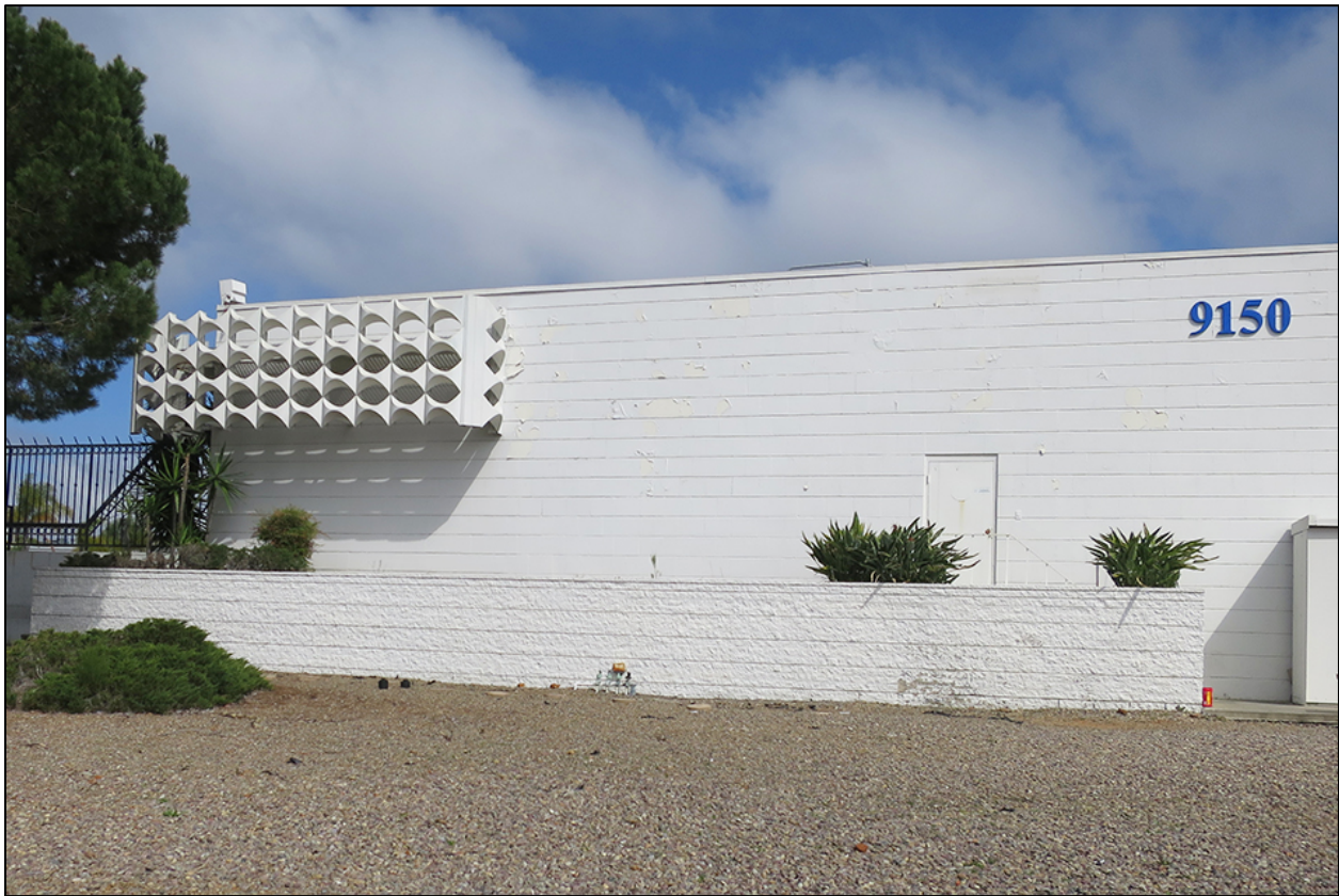
Fig. 24. Decorative pierced metal wraps around the corner of this CMU industrial building at 9150 Balboa Avenue. IS Architecture, 2018.
