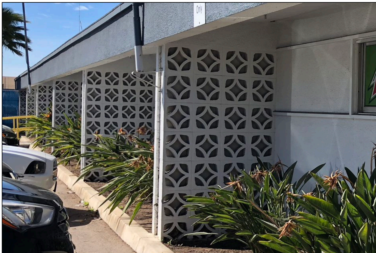
Fig. 22. Decorative pierced block screens on the Pepsi Cola bottling plant at 7995 Armour Street. IS Architecture, 2018.
