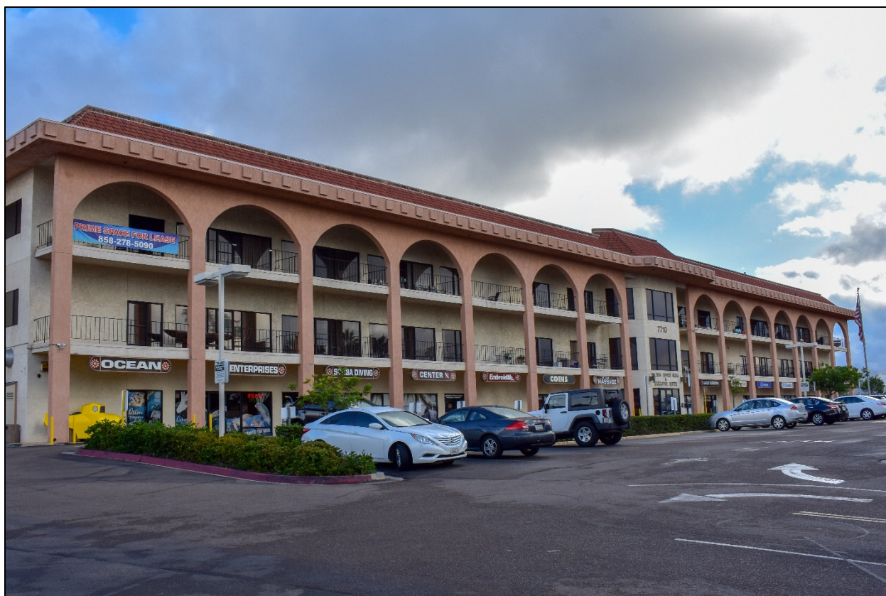
Fig. 35. The Neo-Spanish Eclectic elements of this low-rise office park building at 7710 Balboa Avenue include a red tile roof, arched colonnade, stucco façade, and red, faux tile roof. IS Architecture, 2018.
