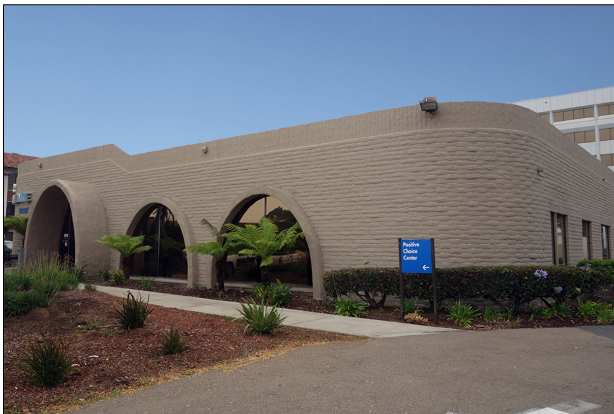
Fig. 21. A Kaiser Permanente site at 7035 Convoy Court. This building's slump block approximates the appearance of an adobe block. IS Architecture, 2018.
