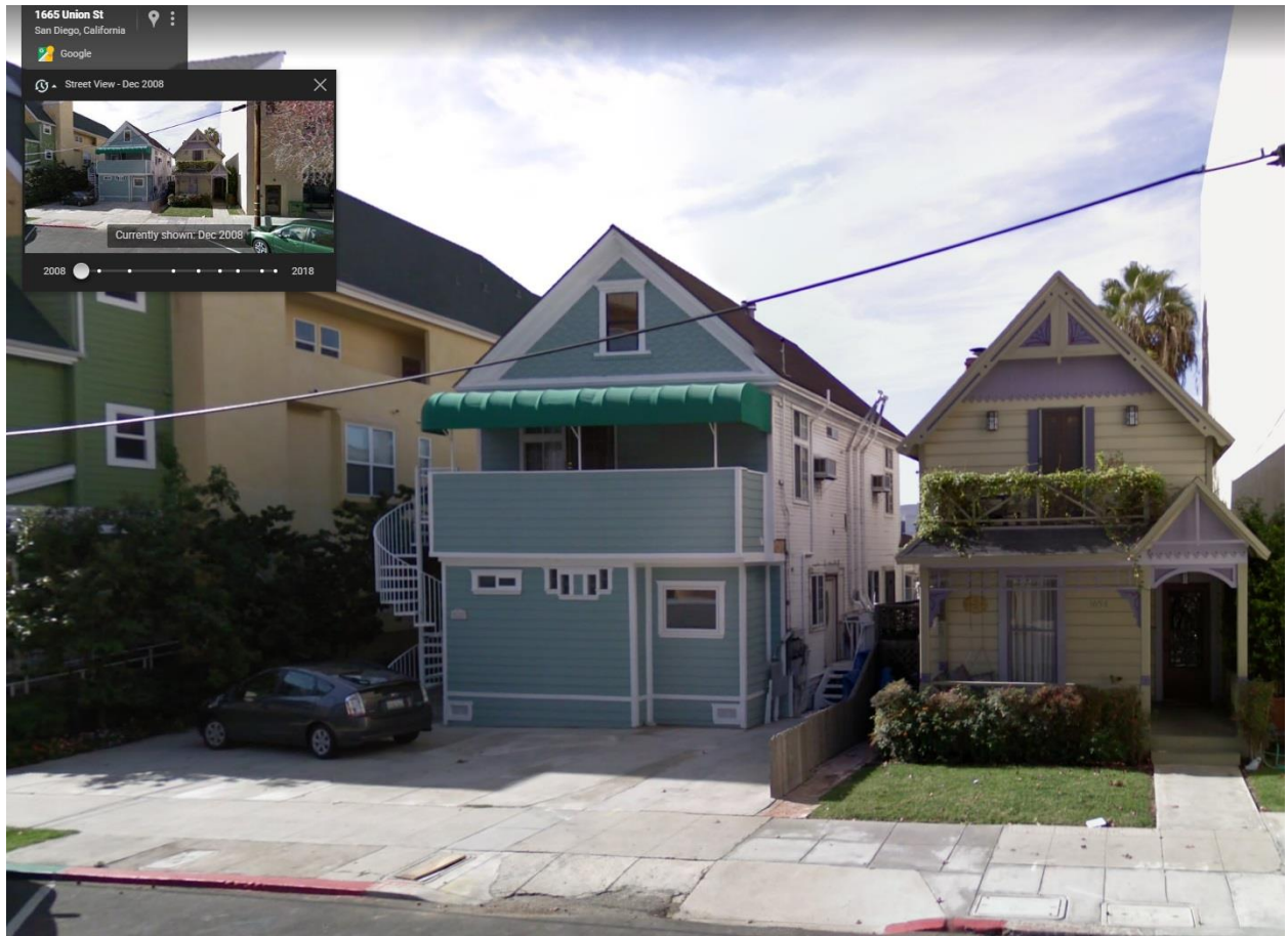
Google Streetview Photo, 1642-1648 Union Street, December 2008
