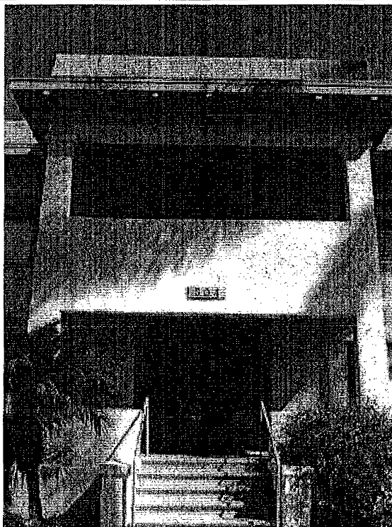
Photo 3: Detail of the main entry with original wood door and window surrounds, colored concrete stair, and non-historic metal pipe railing.
