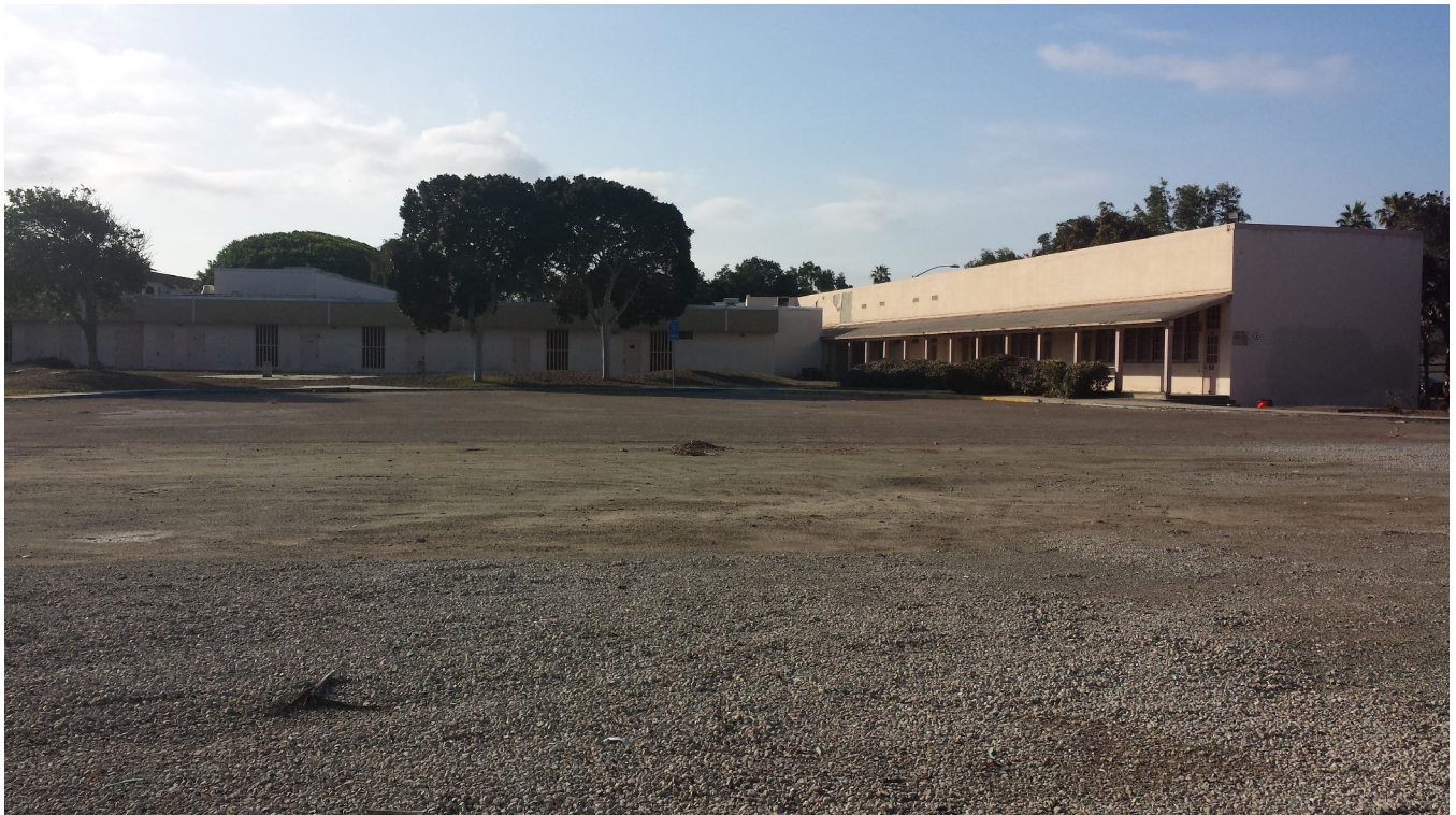
Photo 4: View of gravel parking lot from northern project boundary
