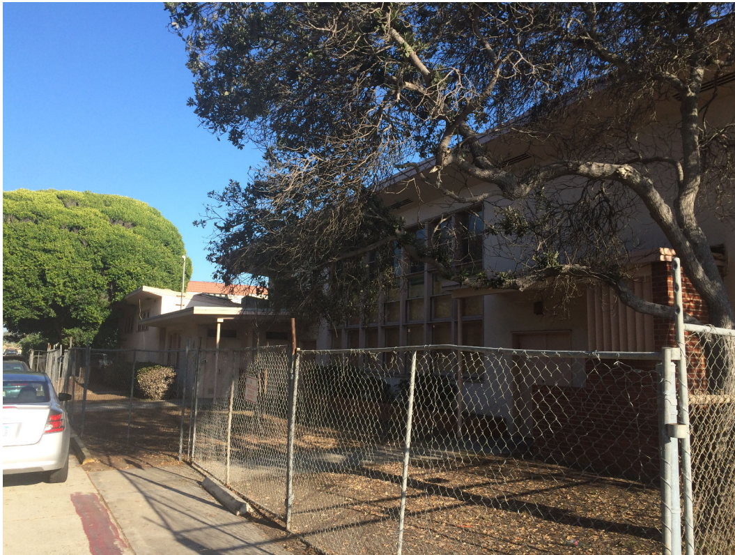
Photo 8: Northwest corner view from Santa Barbara Place
