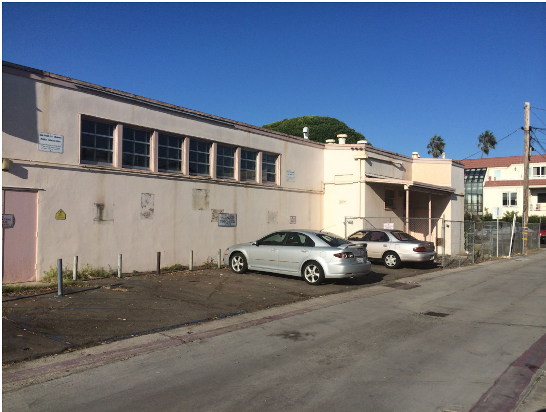
Photo 7: View of Santa Barbara Place south of project site from unnamed alley
