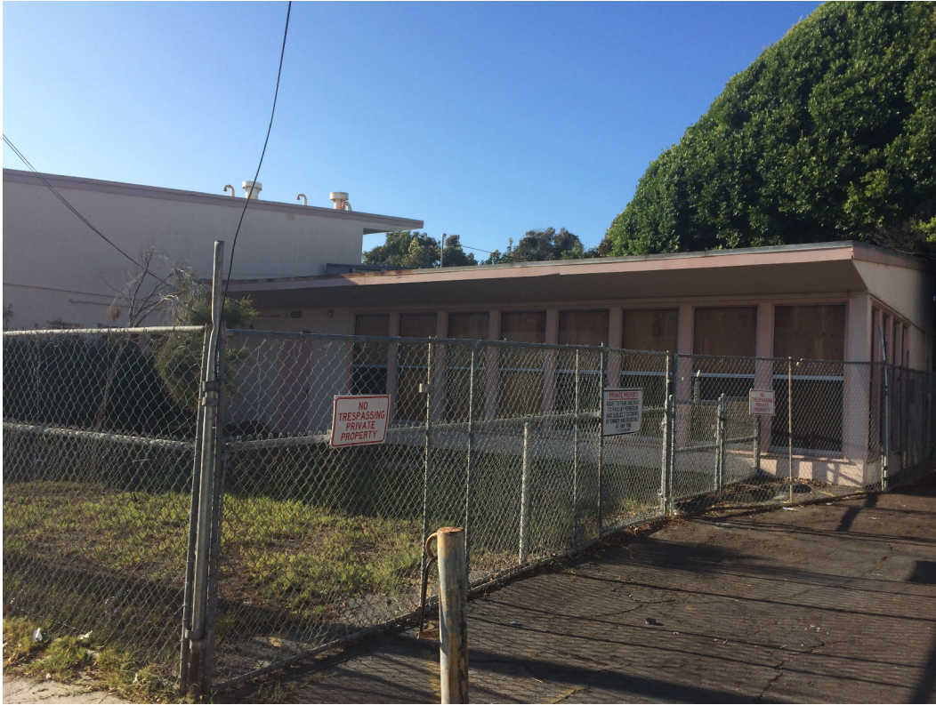
Photo 5: View of southeast corner of project site looking northwest
