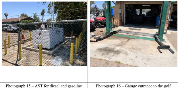
Photograph 15 – AST for diesel and gasoline southwest of the main golf course building and near the golf course maintenance building. Photograph 16 – Garage entrance to the golf course maintenance building with a hydraulic lift and drain in front.
