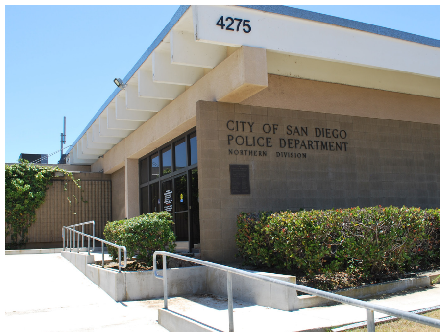
The Northern Division of the San Diego Police Department is stationed in the Planning Area at 4275 Eastgate Mall.
