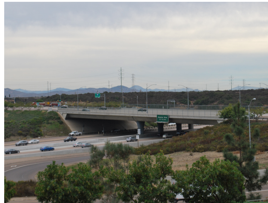
Prominent hillsides are visible from I-805.
