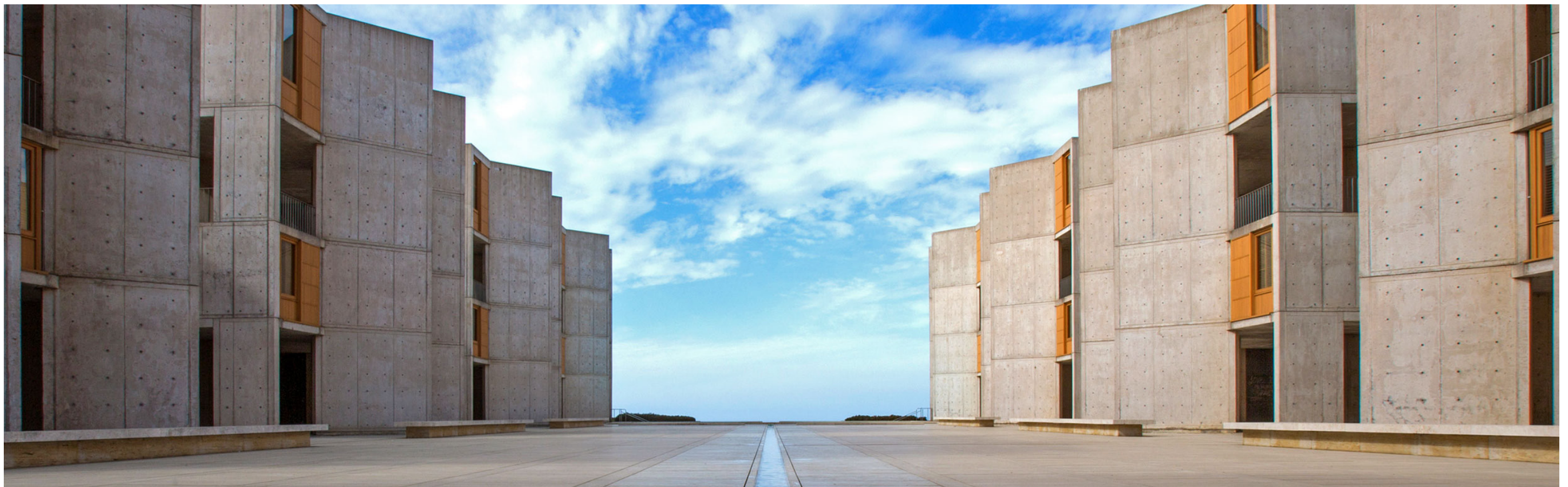
University contains a mixture of building styles, including, clockwise from top left, retail commercial, institutional, office, and research and development. Salk Institute photo credit: Salk Institute for Biological Studies.
