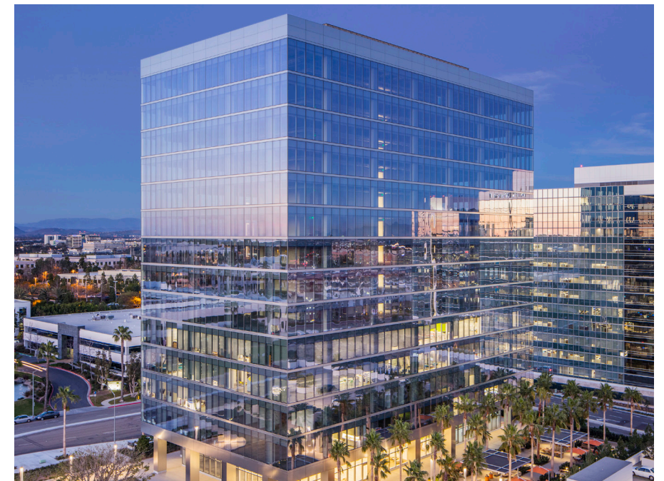
This fifteen-story business center at 4655 Executive Drive, with 350,000 ft 2 building floor area on a 252,648 ft 2 parcel, has an FAR of 1.4.
