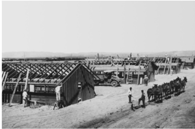
Camp Kearny under construction, c.1917. Image courtesy of the San Diego History Center.
