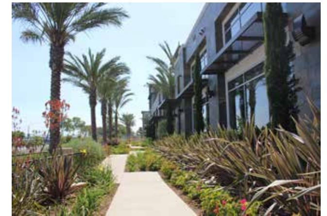
New development orients toward the street, including public realm pathways as defining features of the site plan.
