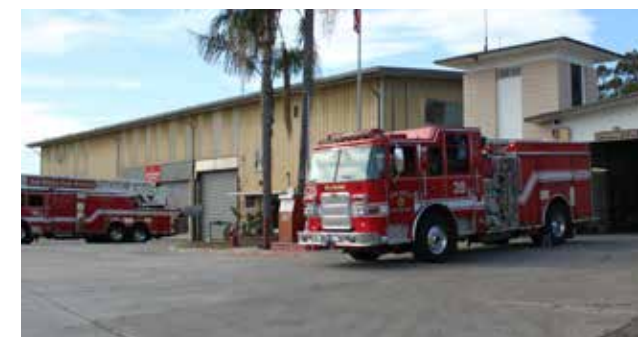
Fire Station 28 located on Kearny Villa Road is centrally located to serve Kearny Mesa and adjacent communities.
