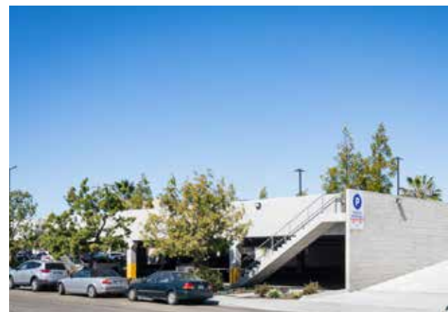
Shared parking structures, like the one built in the Convoy District, can help make parking resources available to many users during peak times.
