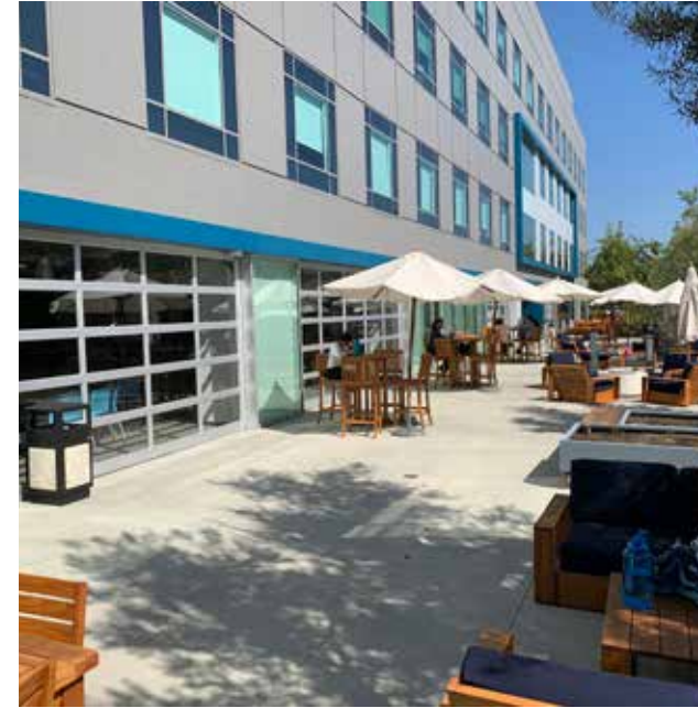
The former FBI headquarters and garage were converted into a modernized multi-tenant office building in 2016.
