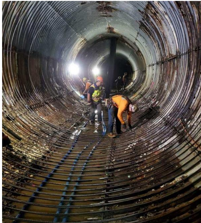
Figure 21: Villa La Jolla Drive stormwater main replacement
