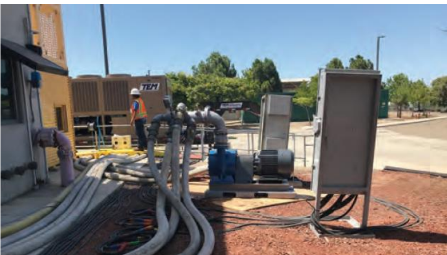
Temporary pump installed during construction
