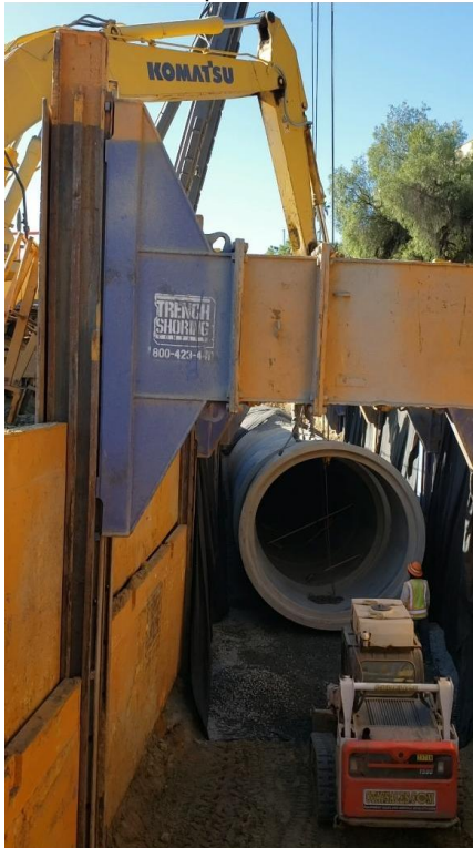
Florida Drive drainpipe installation
