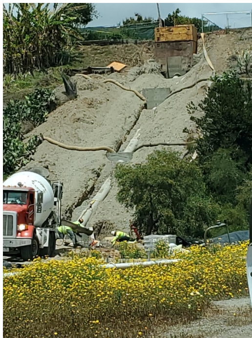
Figure 22: Prairie Mound storm drain repair
