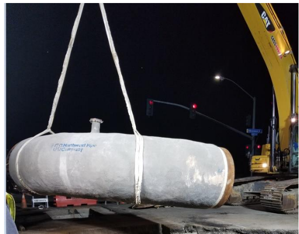
Otay 2 nd Pipeline phase 2 watermain installation
