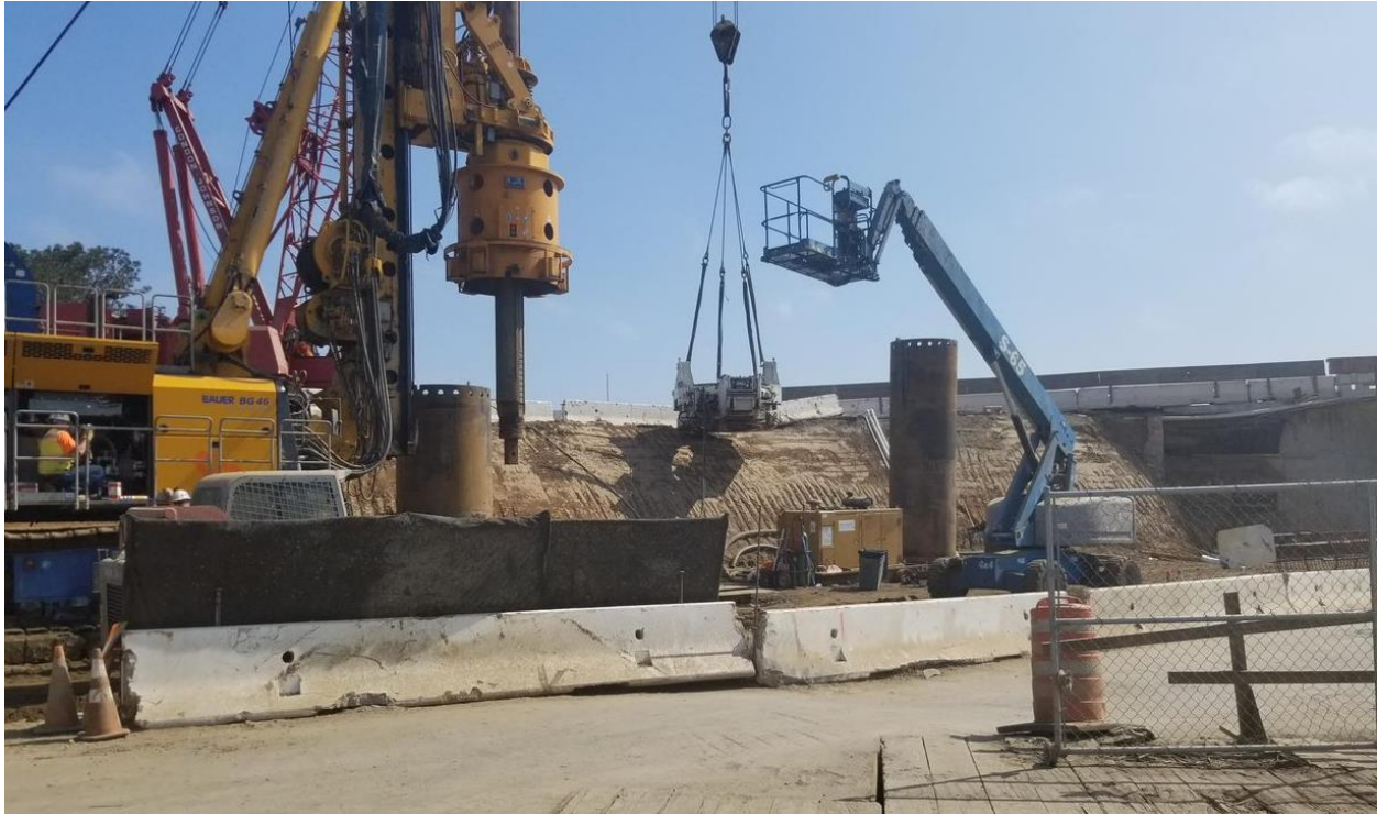
Figure 10: Construction on West Mission Bay Drive Bridge abutment
