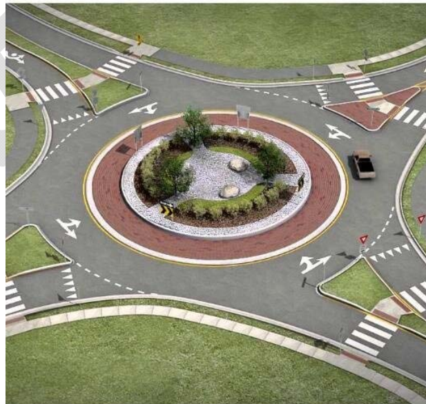
A modern roundabout
