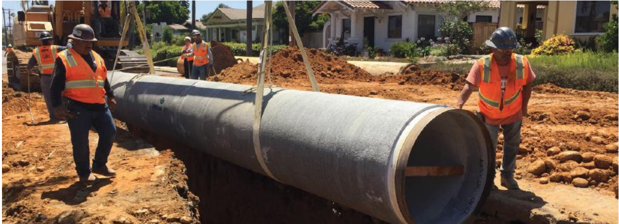
30 th Street water main installation
