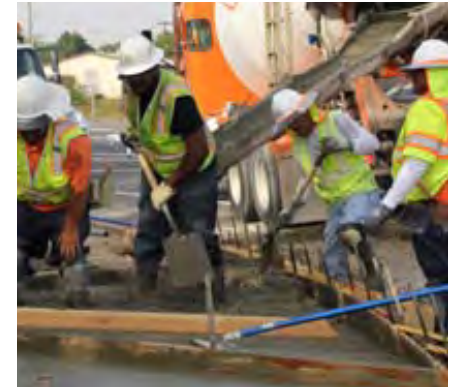
The City can use grants to dedicate funding to priority infrastructure needs, especially in historically underserved communities.
