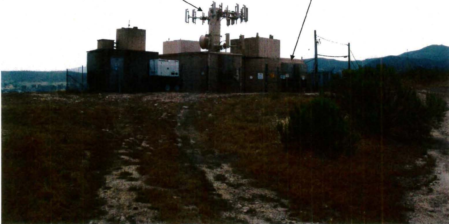
PHOTO SURVEY VIEW 1: Looking east towards the existing project site with the Verizon Wireless components of this multi-carrier site called out (overall site managed by American Tower, Inc.).
