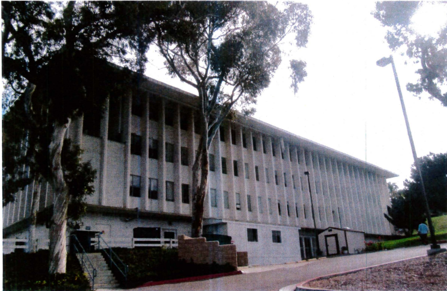
Overall View of Site (Looking East): Photo taken 8/6/14
