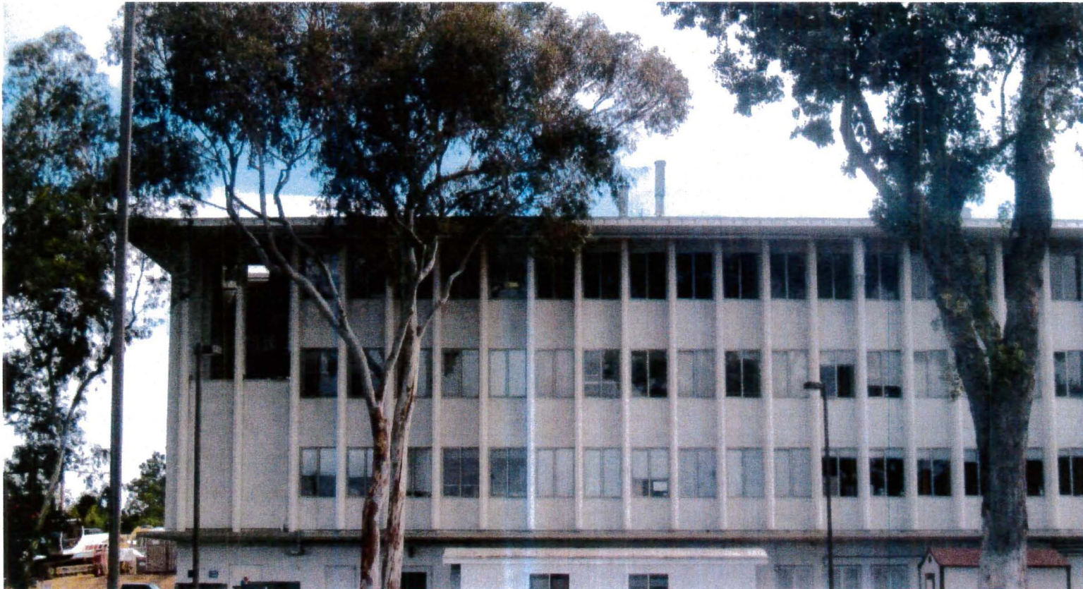
View of Site (Looking North): Photo taken 8/6/14
