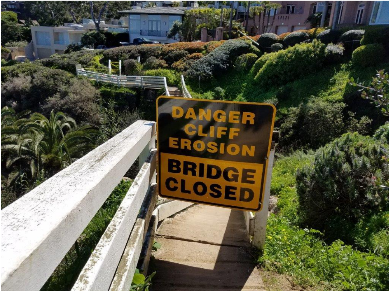
Location "D" – Looking northeast from other side of canyon/bridge
