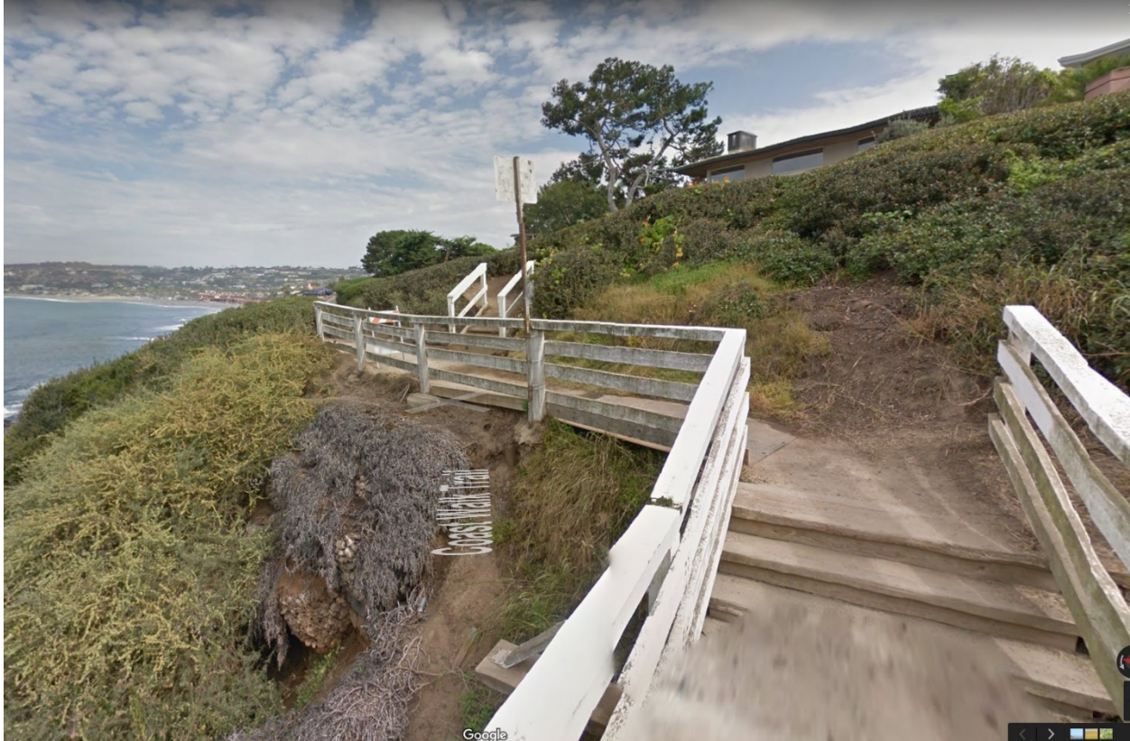
Location "E" – Looking northeast from bridge
