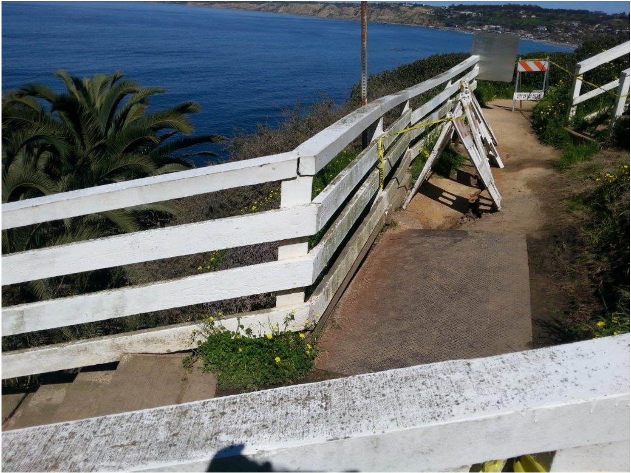
Location B – Looking northeast
