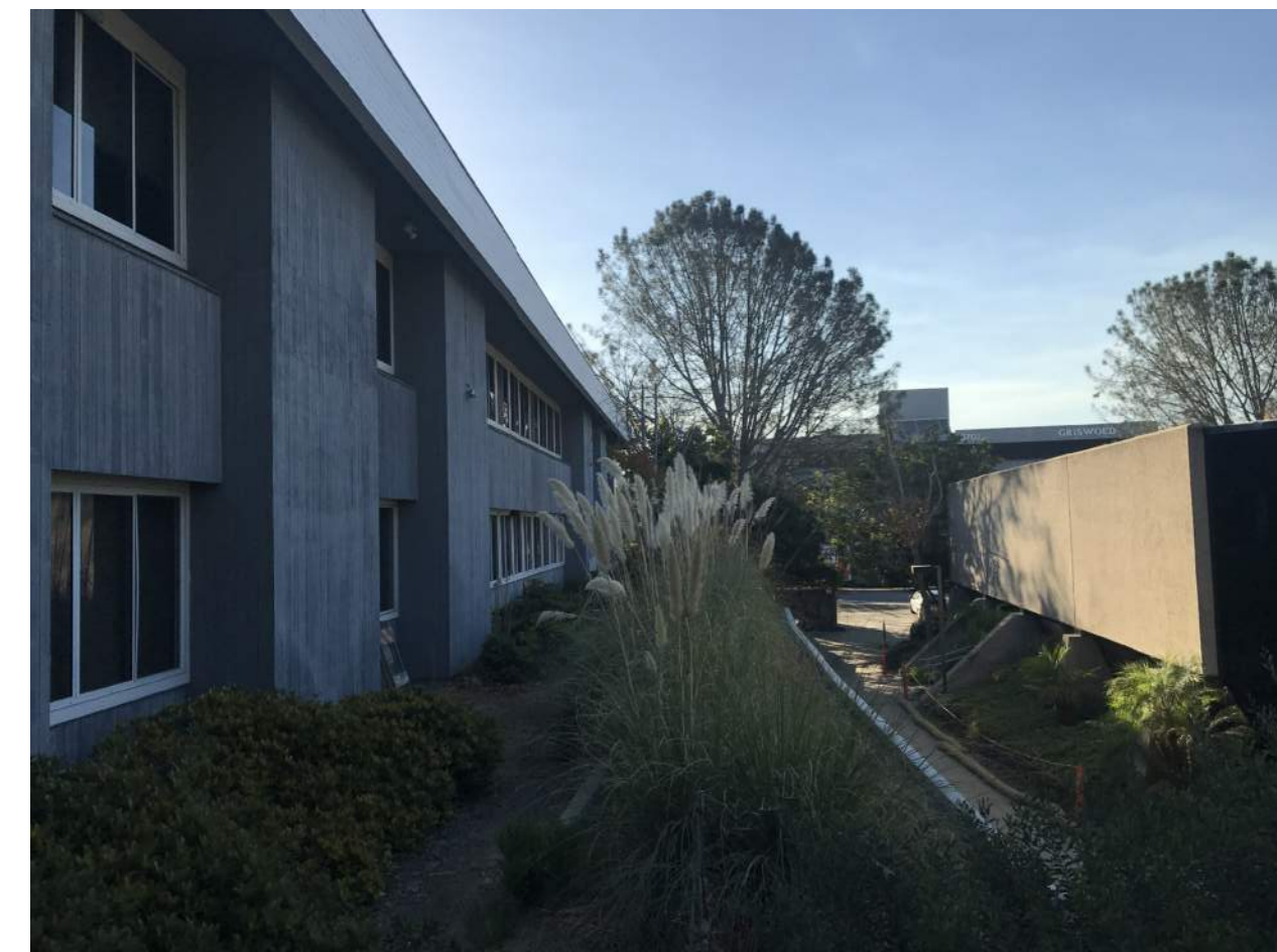
10 BUILDING WEST SIDE LOOKING SOUTH EAST A.7
