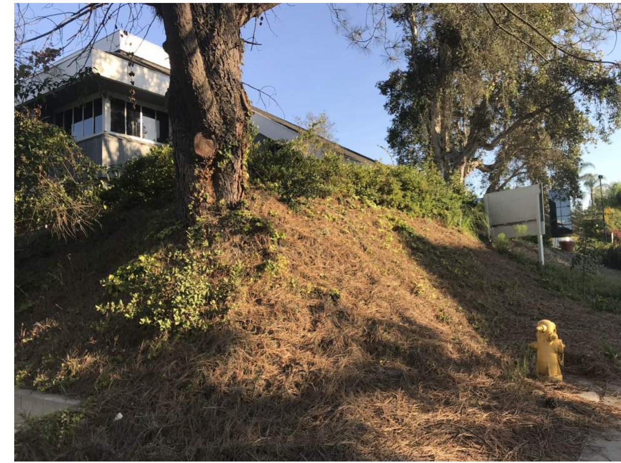
2 OBERLIN DRIVE LOOKING NORTH A.7
