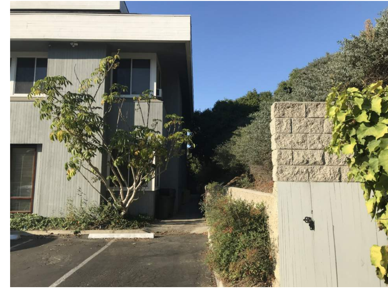
9 BUILDING NORTH END LOOKING SOUTH WEST A.7
