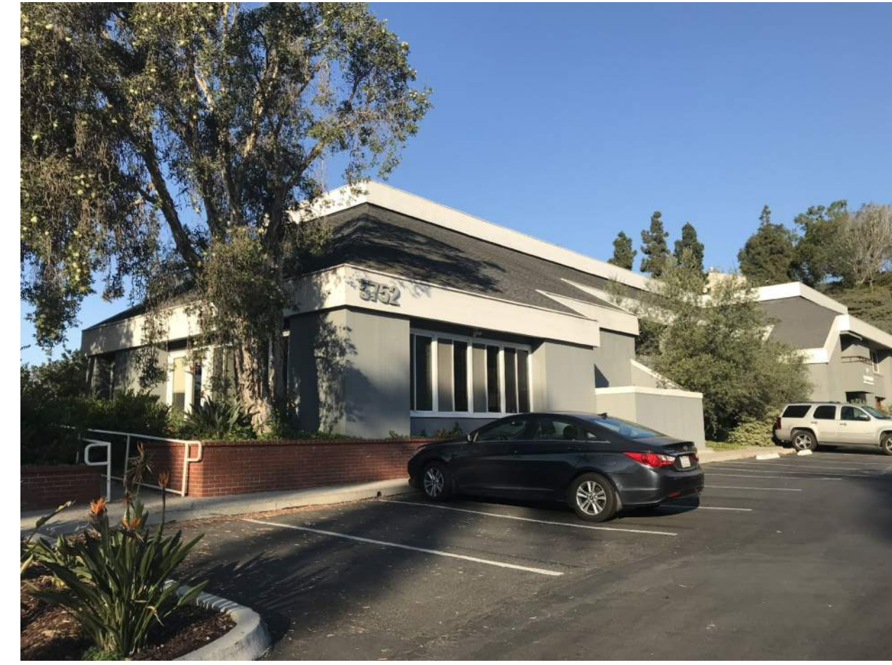
7 BUILDING SOUTH END LOOKING WEST A.7
