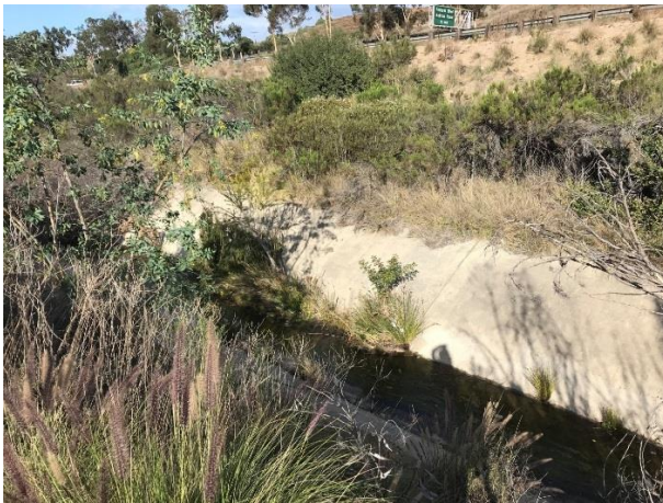
PHOTO NOTES: Map 101, looking downstream from the east end of the maintenance area (2/21/18).
