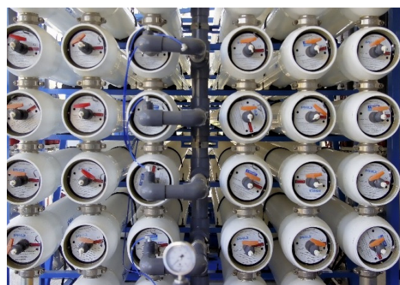
Reverse Osmosis pressure vessels located at the North City Pure Water Demonstration Facility
